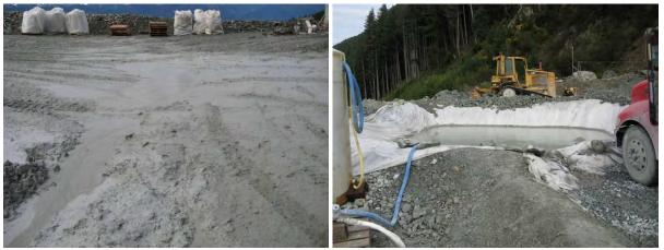
Photos 1 & 2 – Cement slurry at the Comet portal and the cement truck wash sump.
