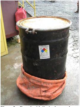
Photo 5 – Barrel with limited secondary containment.
