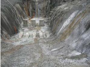
Photo 15 – Seep, possible cavity in shotcrete. Photo 16 - Seeps at the spillway plunge pool.
