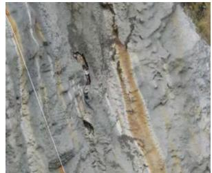
Photo 13 – Spalling shotcrete
