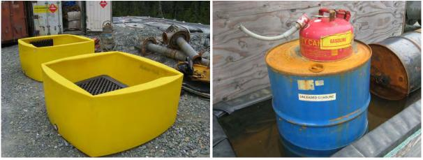
Photo 4 – New secondary containment units Photo 5 – Secondary containment full of water
