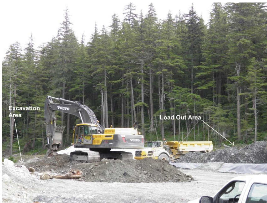
Figure 3 Equipment used to load and haul the graphitic phyllite.
