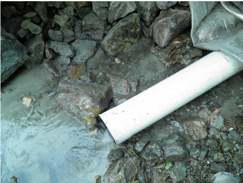
Figure 14 After the culvert was installed.
