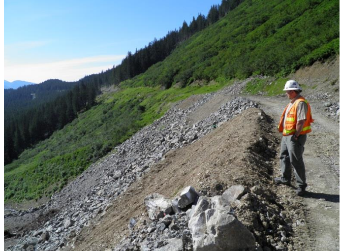
Figure 12 Completed Revegetation Test Plots
