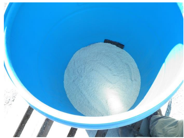
Figure 7 Outlet covered with geotextile at the bottom of the barrel. About 2 more inches of sand was added.
