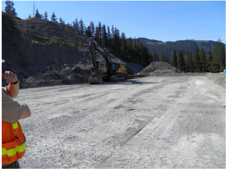
Figure 5 Containment cell near completion.
