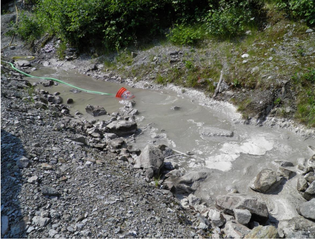
Figure 13 Before the culvert was installed.
