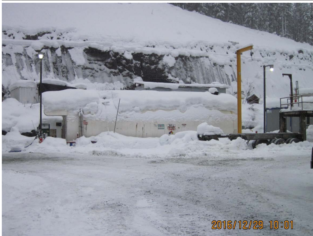
Photo 1. 30,000-gallon “day tank”. Isotainers are placed on the rack (trailer) located on the right side of this photo during refueling. Fuel flows through a filter before entering the day tank.
