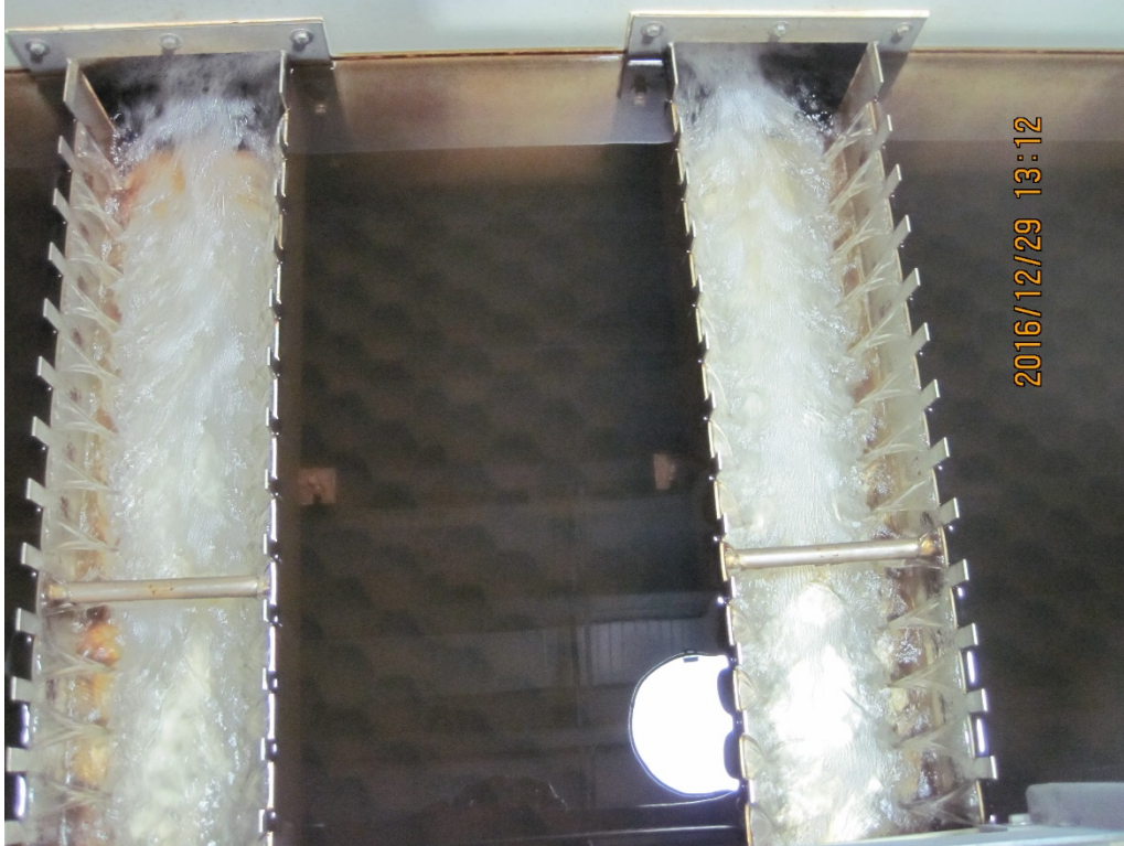
Photo 10. Looking down into the TTF Water Treatment Plant clarifier tank. Operators frequently check the tank for signs of diesel contamination.
