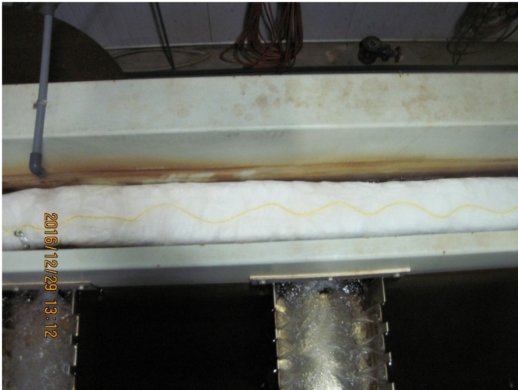
Photo 11. Although no sign of diesel has been observed at the TTF, Coeur Alaska crews placed an oil containment boom at the clarifier tank outlet to catch potential contamination. Crews will change the boom regularly and checked it for diesel.
