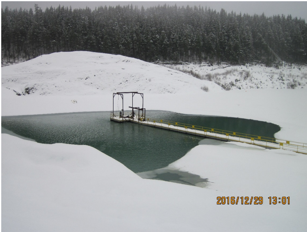
Photo 9. TTF water reclaim barge. Located about 100 meters south of the tailings barge, the reclaim barge pumps water to the TTF Water Treatment Plant. Agitators on the barge keep the surrounding area ice-free and provide another window to observe potential sheens.
