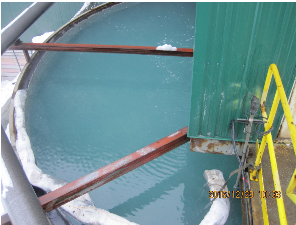
Photo 7. Tailings thickener tank. Coeur Alaska crews placed oil containment booms on the surface of the tank to contain and capture diesel. Crews originally spotted a sheen on the tank on December 22.
