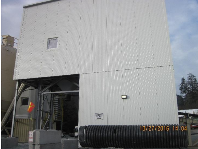
Photo 13. Pug plant at Pit 4.
