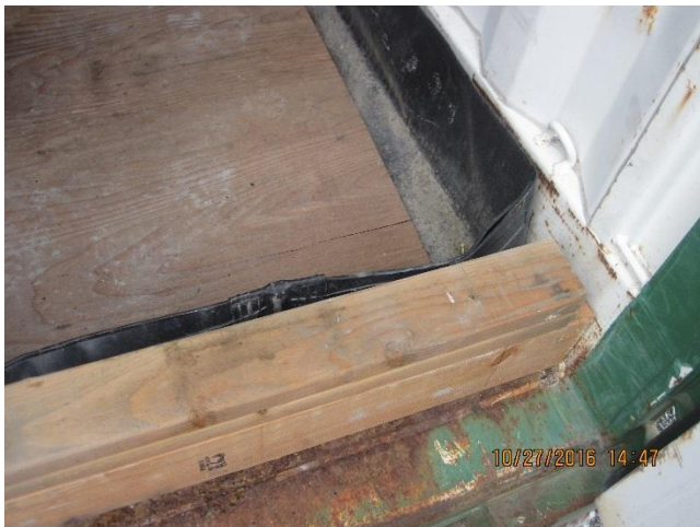
Photo 21. TTF storage containers with secondary containment.
