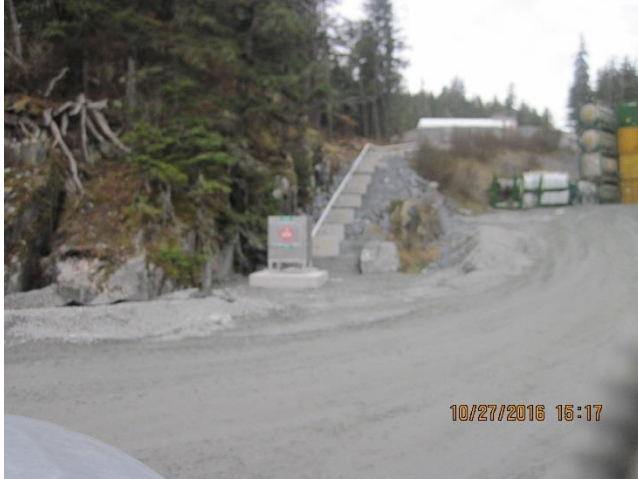
Photo 28. The Kensington port fuel transfer pipeline.
