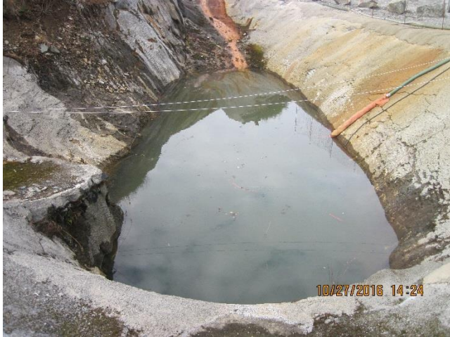
Photo 19. The TTF dam plunge pool.
