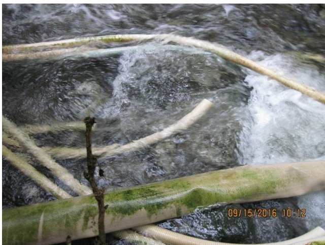
Photo 6. Sherman Creek Outfall (Outfall 001).
