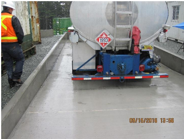
Photo 26. Fuel depot concrete fueling pad.
