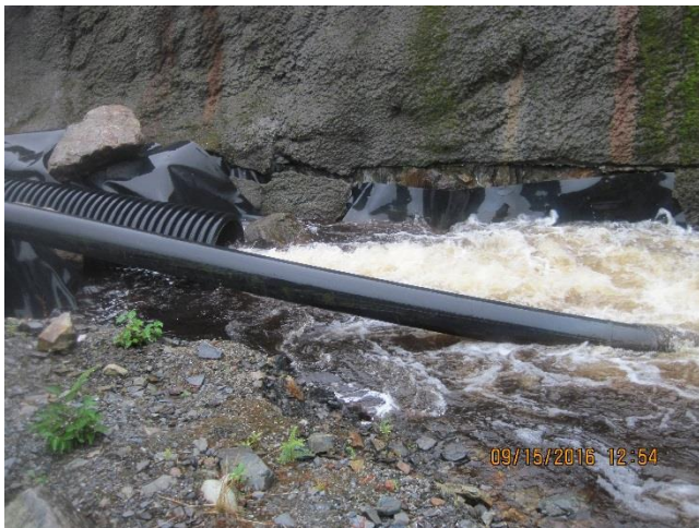
Photo 17. TTF spillway and Slate Creek bypass.
