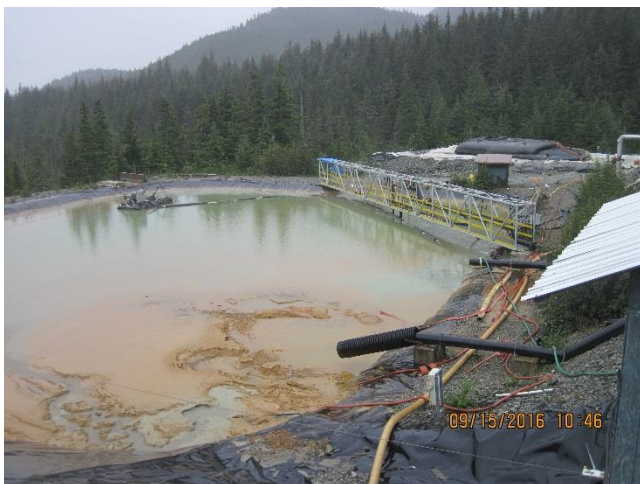
Photo 3. Comet water treatment plant Pond-2.
