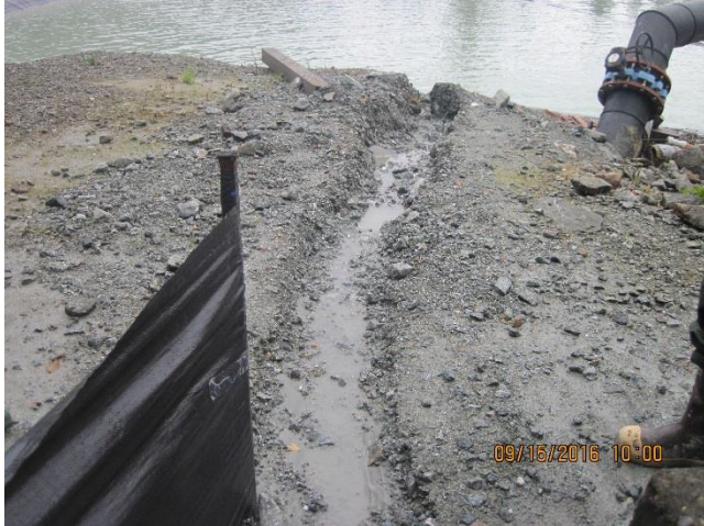
Figure 4. Silt fence and trench for conveying stormwater runoff to Pond-1.
