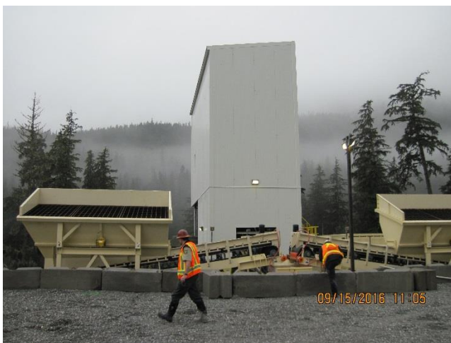
Photo 15. Pug plant at Pit 4.
