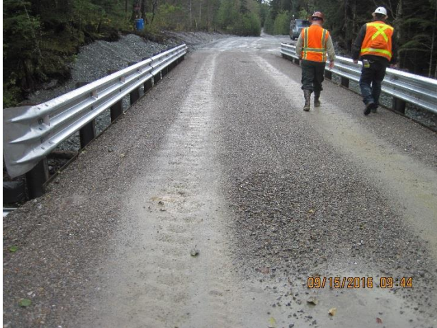
Photo 10. Lower Sherman Creek Bridge for the Comet access road is installed.
