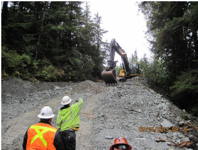
Photo 14. Image shown is 2 of 2 upper Sherman Creek Bridge abutment.
