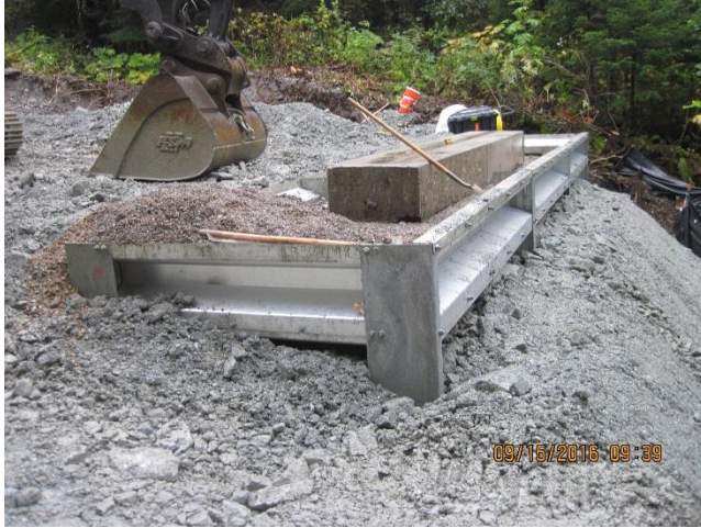
Photo 13. Image shown 1 of 2 upper Sherman Creek bridge abutments have been installed.
