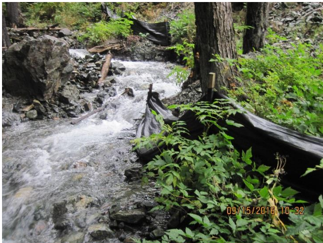
Photo 8. A section of silt fencing crossing Ophir Creek has been removed.
