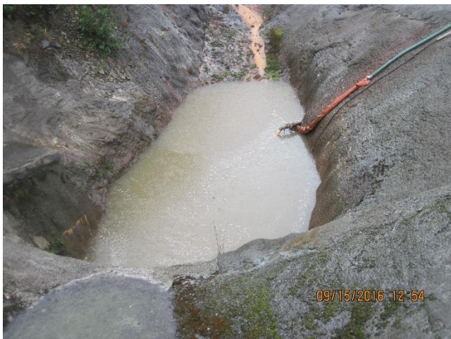
Photo 18. TTF dam spillway/plunge pool.
