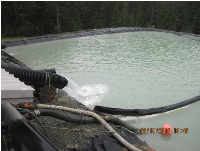
Photo 2. Comet water treatment plant Pond-1.
