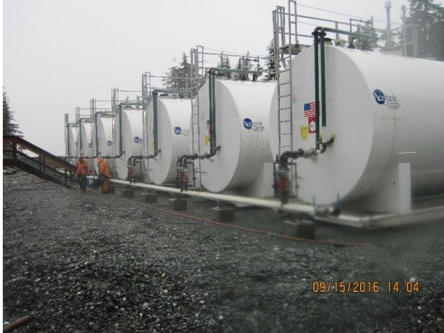
Photo 22. Seven fuel tanks installed.
