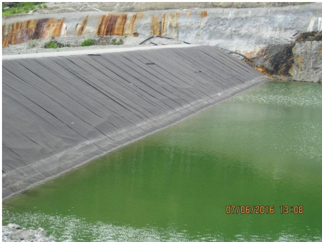
Photo 26. TTF water level is 694.3 feet.
