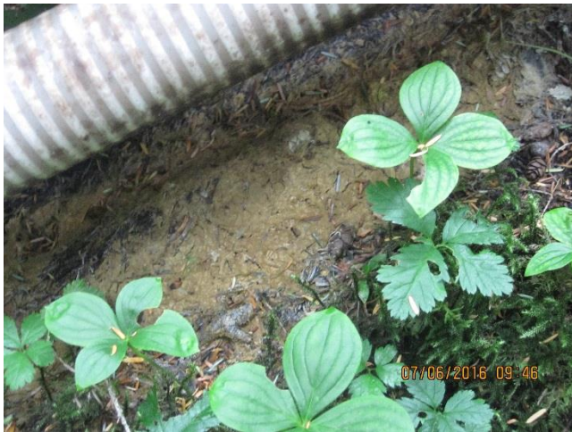
Photo 17. White material observed under other outfall hoses.
