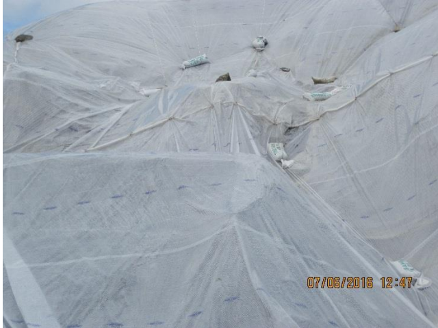
Photo 25. Pit 7 GP liner repaired.
