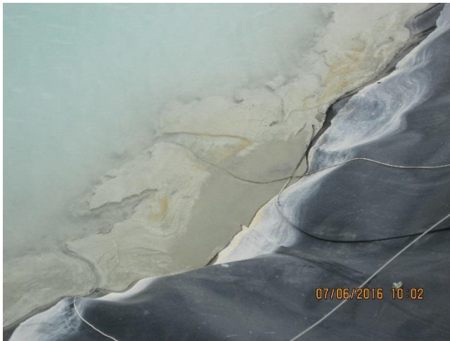
Photo 5. Pond-1 liner with white material.
