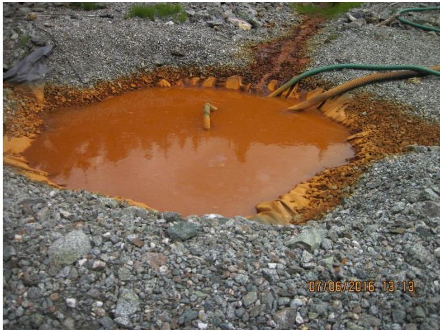
Photo 29. Zoomed in image of an ARD catchment at the northern section of the TTF.
