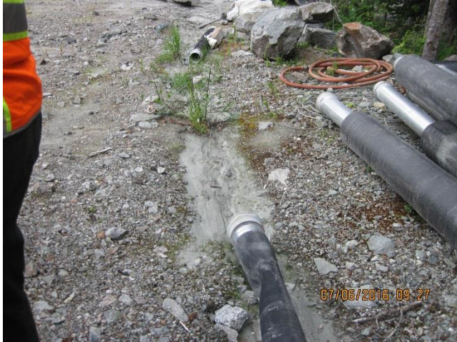
Photo 10. Diversion ditch located behind the Comet water treatment plant.
