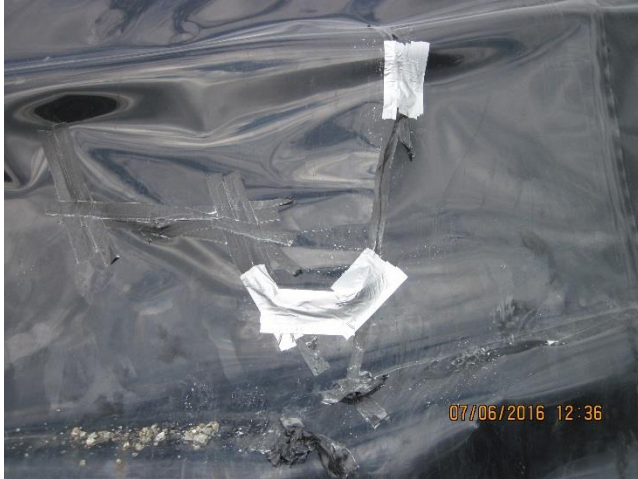
Photo 22. Mud Dump GP liner repaired.
