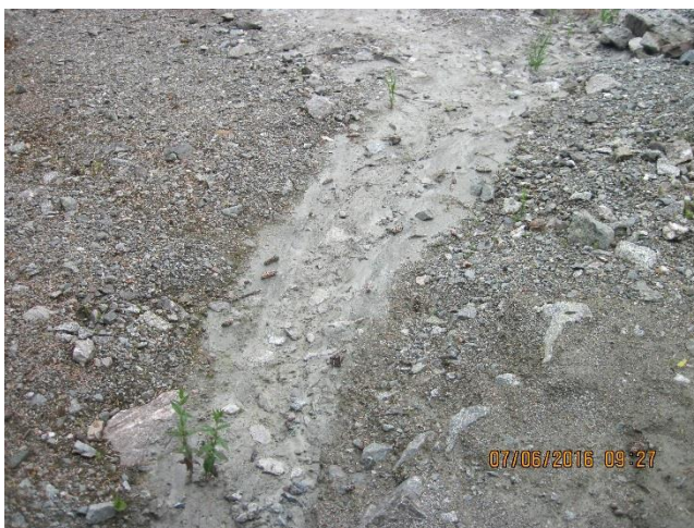
Photo 9. Diversion ditch behind the Comet water treatment plant.
