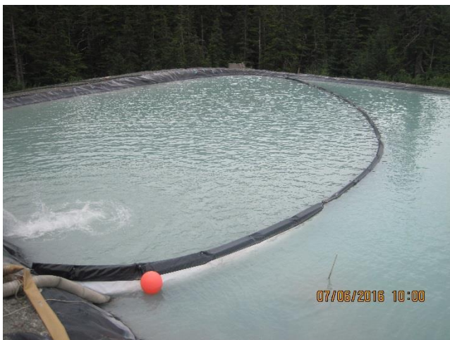
Photo 3. Pond-1 with a silt curtain for sediment area reduction.
