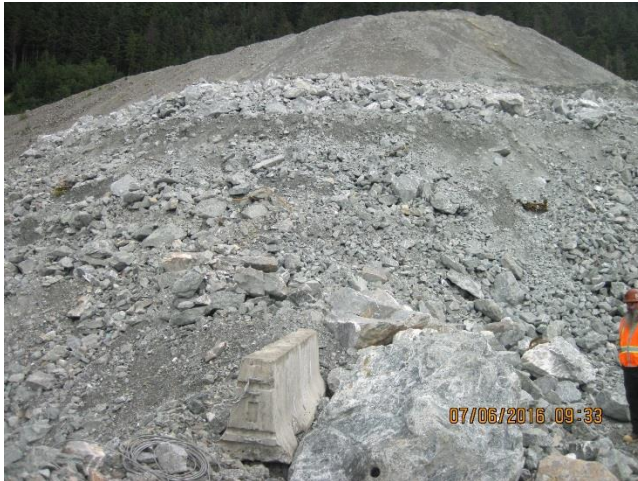
Photo 2. Comet development pile South-West toe expansion.
