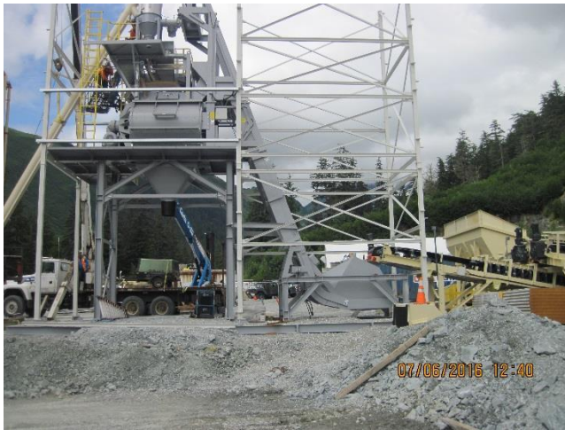
Photo 23. Plug plant structural steel construction.
