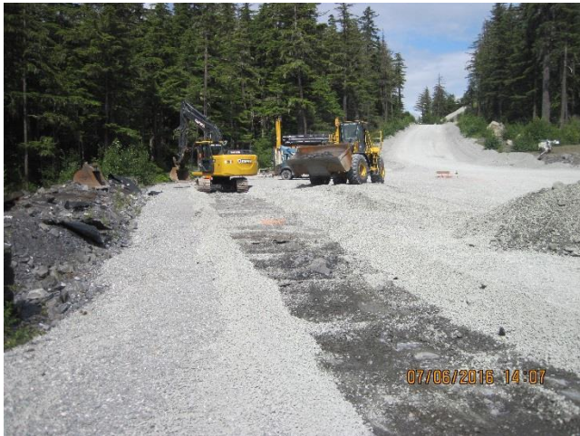
Photo 32. New fuel depot location.
