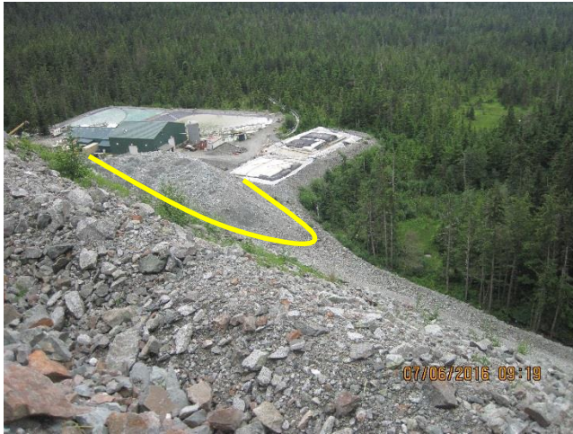
Photo 1. The area within the highlighted line is the location for the Comet development pile toe expansion.
