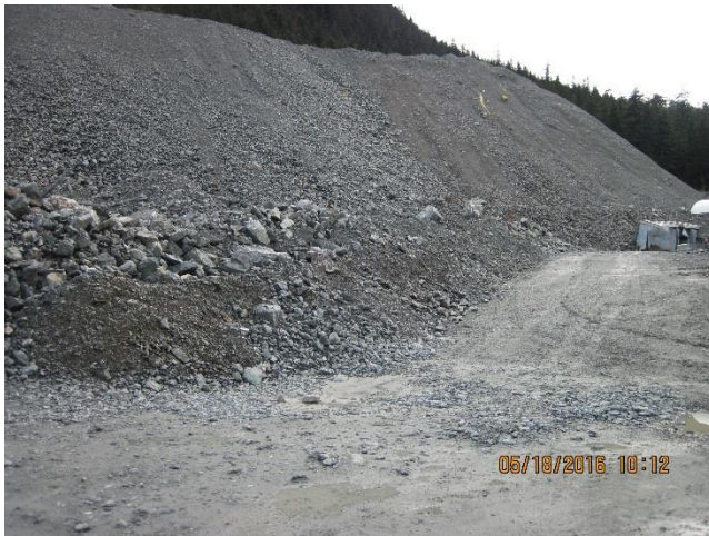
Photo 2. The base of the Comet Development Pile's toe expansion.
