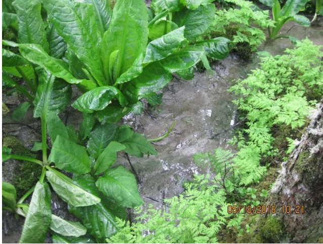
Photo 7. Sediments deposited onto the forest duff due to a washed out diversion ditch.
