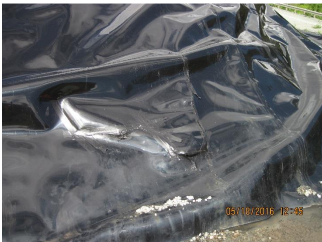
Photo 18. Repaired liner for GP material at the Mud Dump.
