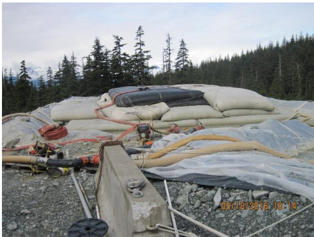
Photo 6. Dewatering bags used for removing sediments from water.
