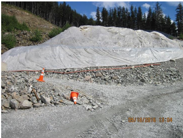
Photo 17. GP material covered with a poly liner at Pit 4.
