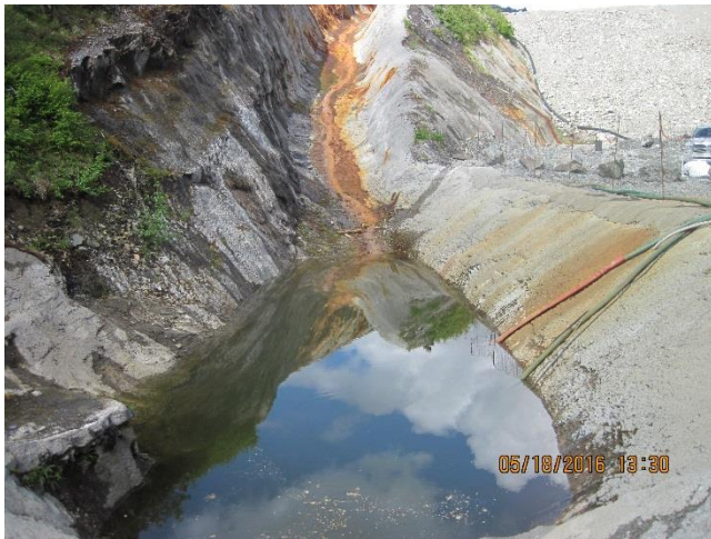
Photo 23. TTF dam spillway and plunge pool.
