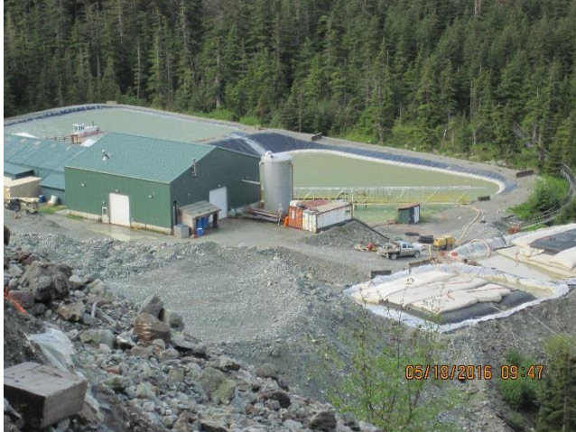
Photo 1. Comet Development Pile's toe expansion.
