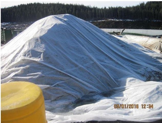
Photo 2. Covered sludge material from the GP seep treatment plant.
