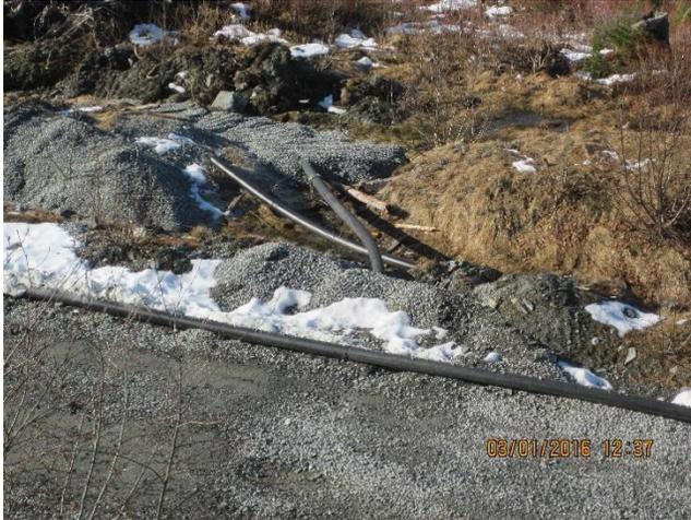
Photo 1. Infiltration gallery for effluent water pumped from the GP seep plant.
