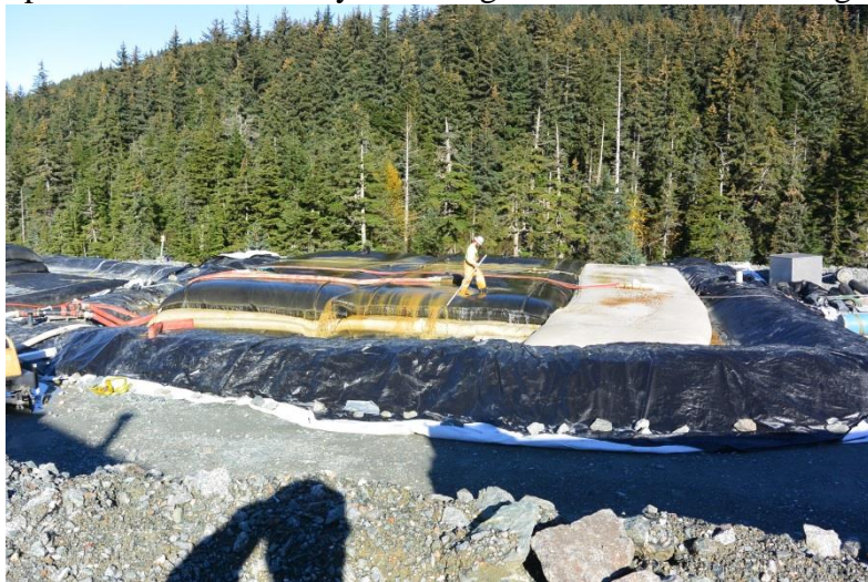
Figure 3 Dewatering bags inside lined containment.
