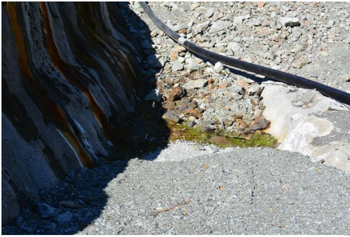
Figure 10 Filled Stage One Emergency Spillway. upstream of the TTF Dam.
