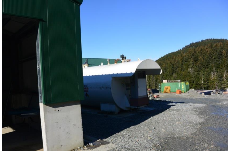
Figure 5 New building and fuel tank.
