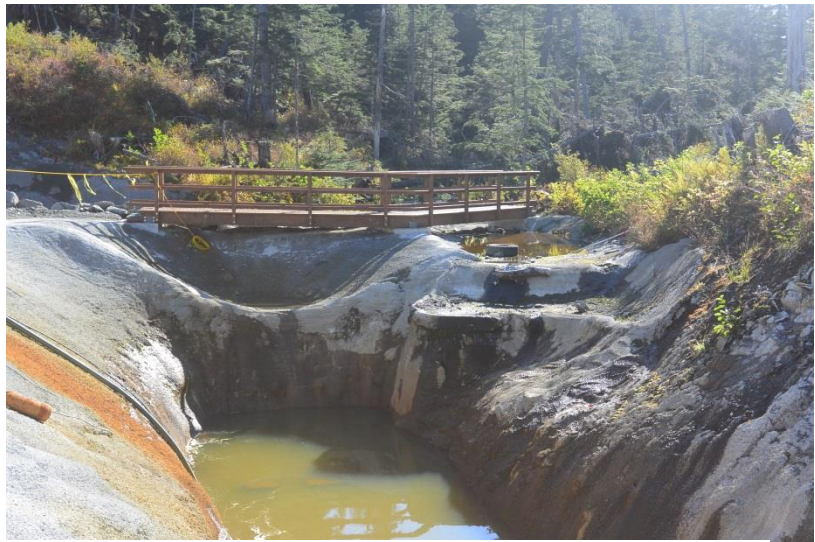
Figure 9 New walkway leading to a water quality monitoring site.
