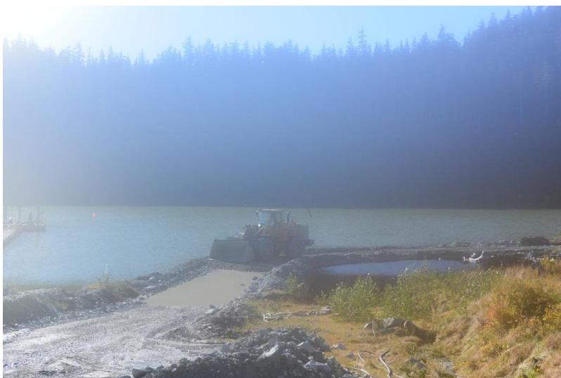
Figure 12 A loader raising the elevation of the road bed. The haze is caused by a fogged up camera lens.
