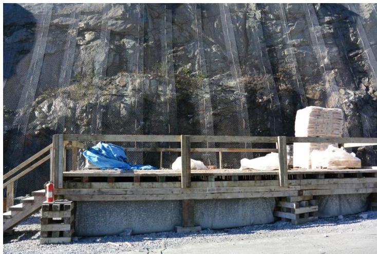
Figure 6 Site of the proposed new portal.
