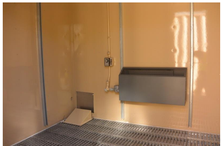
Figure 4 Inside of a new 20 foot container. Note the integrated secondary containment, heater and floor vent.
