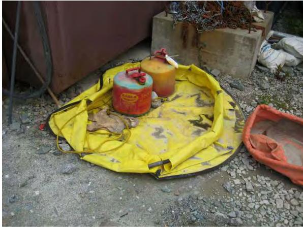
Photo 6 – Collapsed secondary containment
