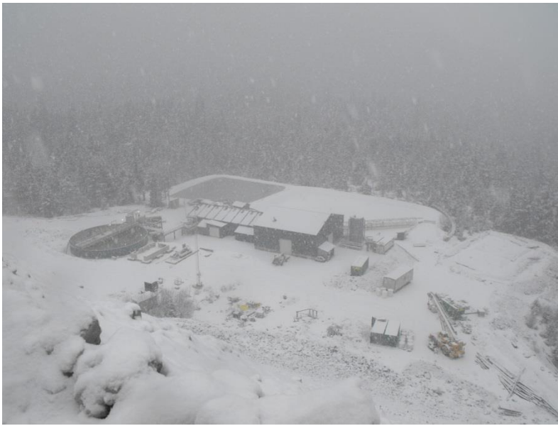
Figure 3 Comet water treatment plant. Looking southwest from the wasterock pile.
