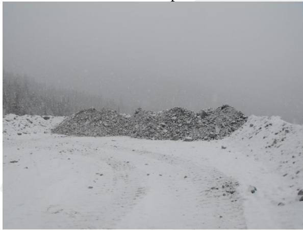
Figure 1 Looking south on the top of the Comet wasterock pile.
