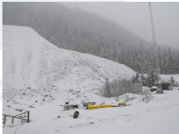
Figure 2 Lift at the south end of the wasterock pile. Looking southeast from the Comet WTP.
