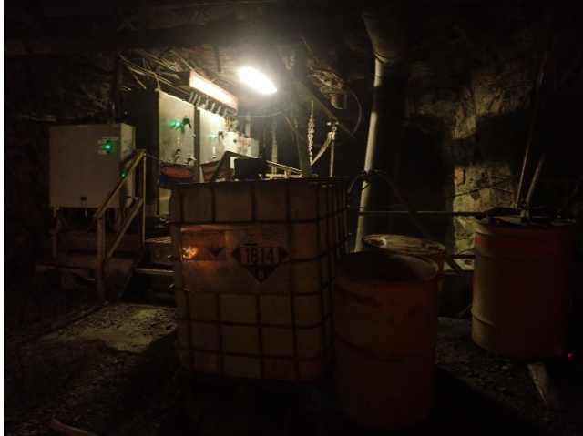
Photo 4. Z-Clear 129 being added to mine water at sump.
