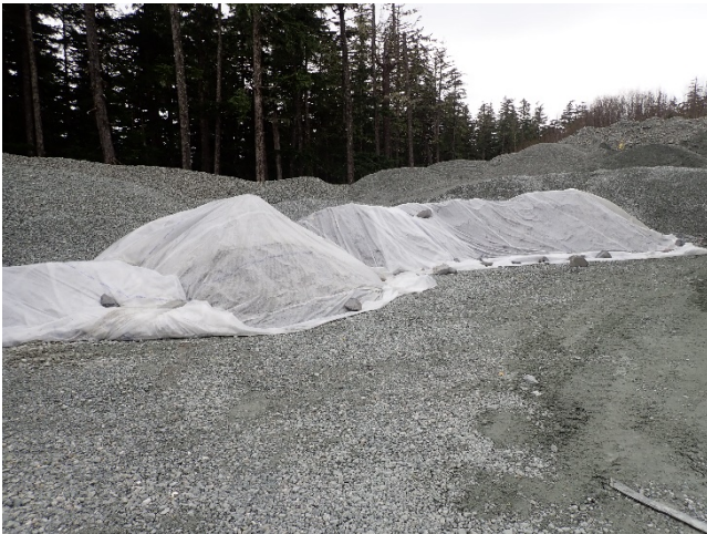
Photo 18. Stockpiled fuel-contaminated soil.
