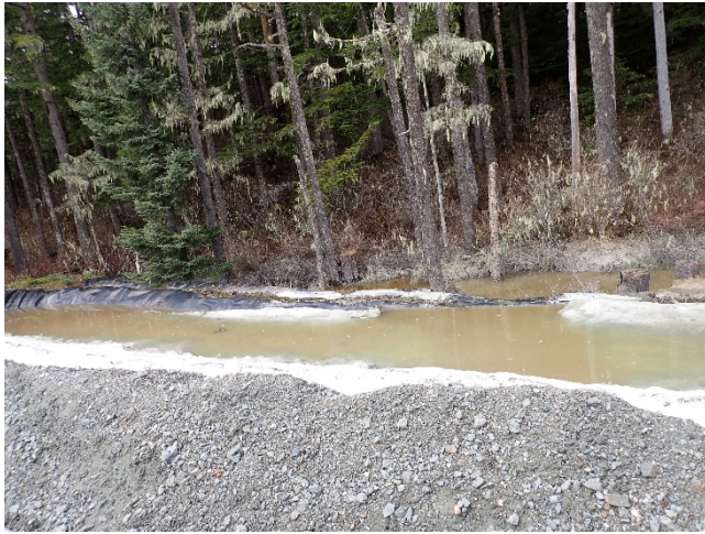
Photo 1. Overflow on TTF Spur Road.
