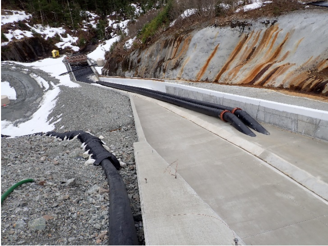
Photo 22. TTF dam spillway.
