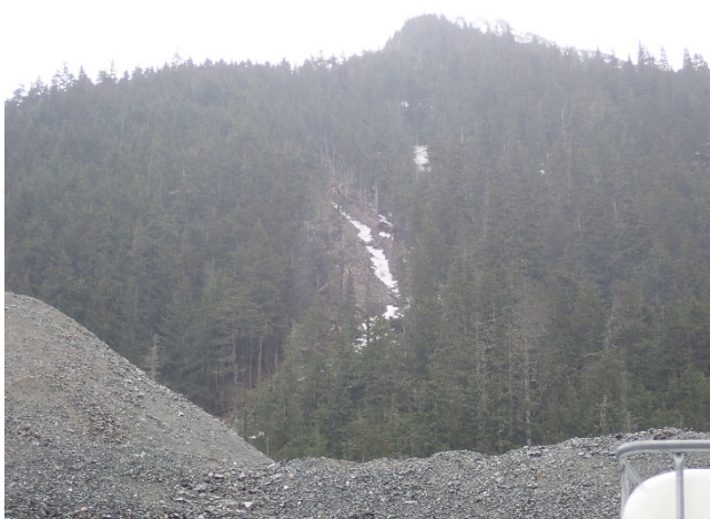
Photo 6. Landslide scarp above Comet Road.
