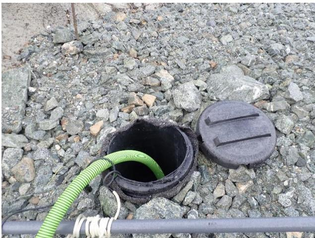
**Photo 14. Acid rock drainage (ARD) seepage collection drain.**
