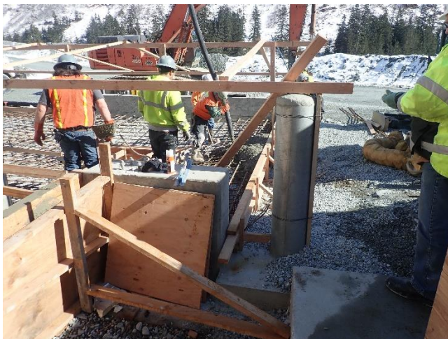
Photo 14. Contractors pouring cement for the new refueling pad.
