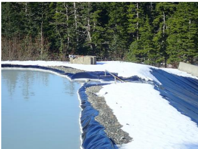
Photo 5. Water flowing over Pond-1's spillway and into Pond-2.
