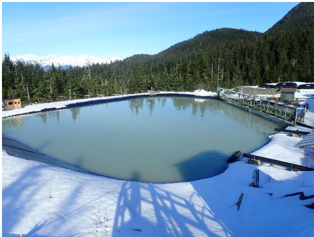
Photo 4. The CWTP's Pond-2.
