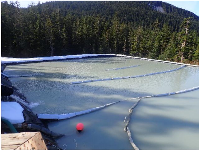
Photo 3. CWTP's Pond-1 requires dredging and installation of new silt curtains.
