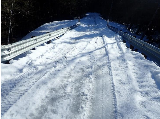
Photo 9. The South fork Sherman Creek Bridge.
