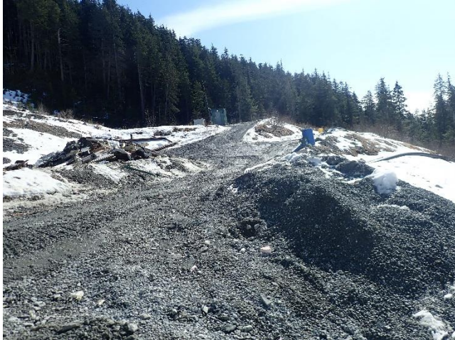
Photo 21. The decommissioned seep plant was removed for the TTF's dam construction.
