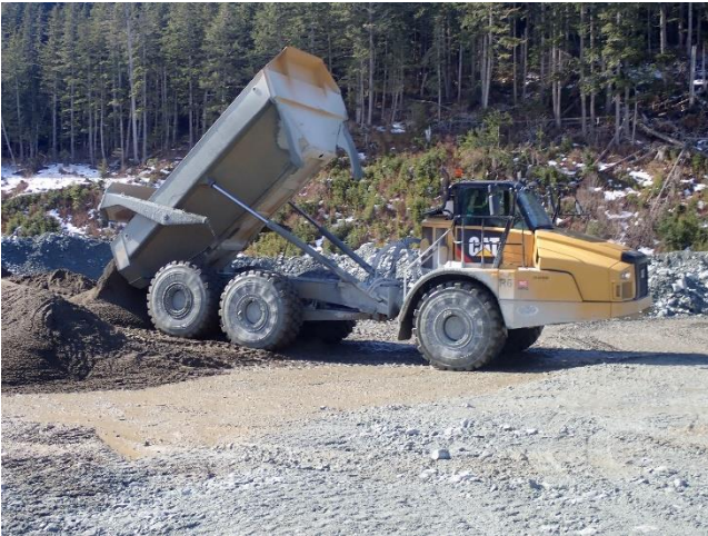
Photo 19. Cement aggregates staged at the TTF laydown yard.
