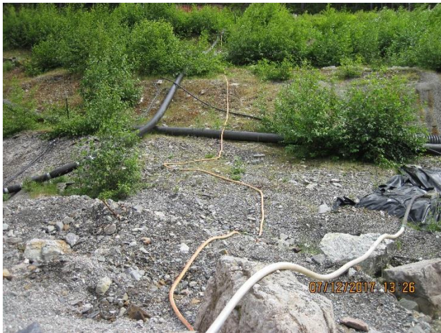
Photo 17. Water hoses for the geo-tech drilling pad located in the southern TTF area.
