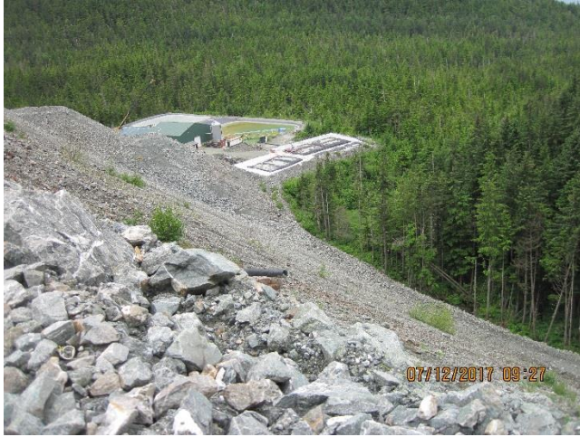
Photo 1 Comet Development Pile.
