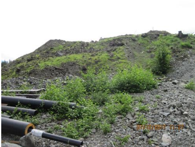
Photo 11. 8,000 yd 3 of reclamation soil was hand seeded at the Mud dump.
