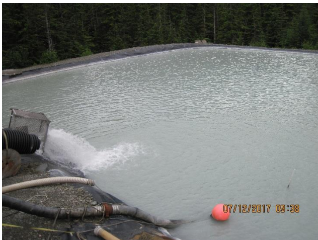
Photo 3. Comet Water Treatment Plant's Pond 1.
