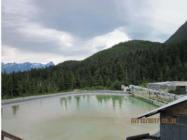
Photo 4. Comet Water Treatment Plant's Pond 2.
