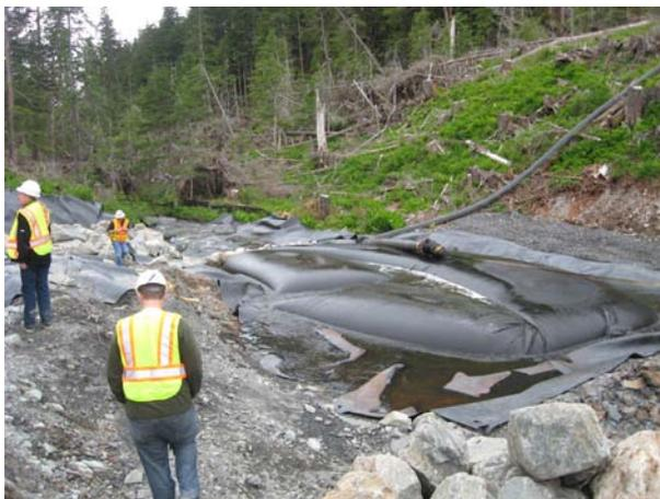
Sediment bag for dewatering water into E. Fork Slate Creek
