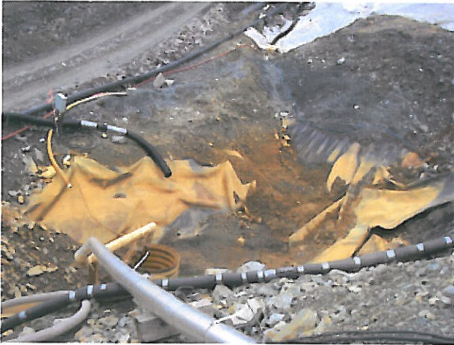
PHOTO 13: ARD SEEPAGE COLLECTION SUMP WAS EMPTY
