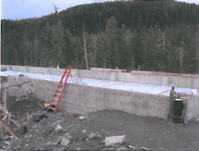
PHOTO 15: TTF WATER TREATMENT PLANT UNDER CONSTRUCTION
