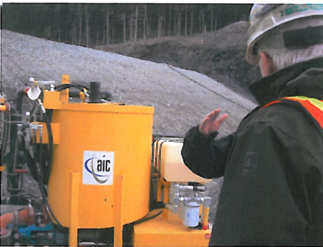
PHOTO 3: KNIGHT-PIESOLD PERSONNEL EXPLAIN GROUTING OPERATION TO MR. TOM CRAFFORD/ADNR
