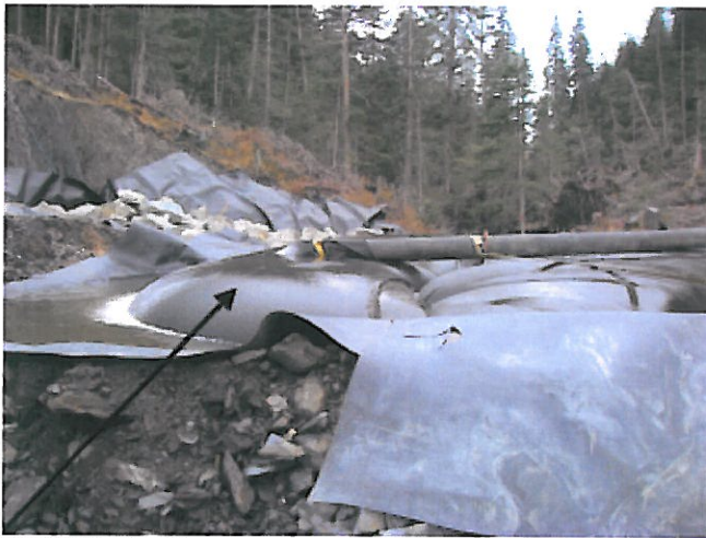
PHOTO 9: SEDIMENT BAG FILTERS WATER PRIOR TO DISCHARGE (UPSTREAM OF SAMPLE LOCATION # 5)
