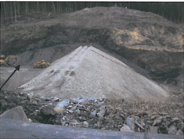
PHOTO 5: COFFERDAM AT TTF FROM FLUME.
