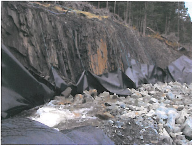
PHOTO 11: BLACKISH MATERIAL ON FACE ABOVE LINER IS GRAPHITIC PHYLLITE WHICH WILL BE REMOVED, THEN CAPPED
