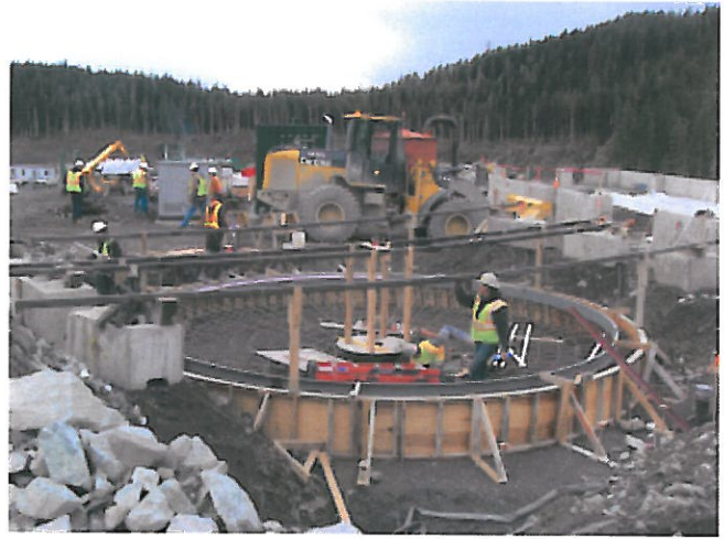
PHOTO 14: TTF WATER TREATMENT PLANT. FOUNDATION FOR CLARIFIER IN FOREGROUND
