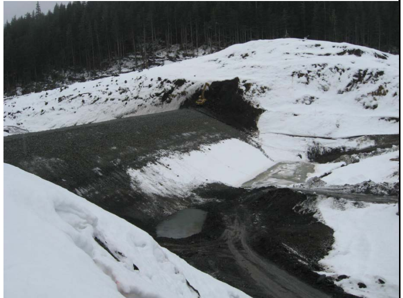
PHOTO 2. DAM FROM EAST EMBANKMENT
