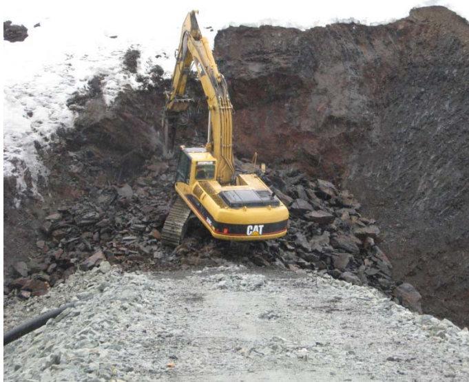
PHOTO 3. PREPARATORY WORK ALONG GROUT TRENCH
