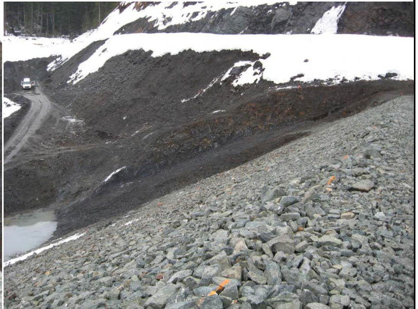
PHOTO 4. EAST EMBANKMENT PREPARED FOR DRILL RIG
