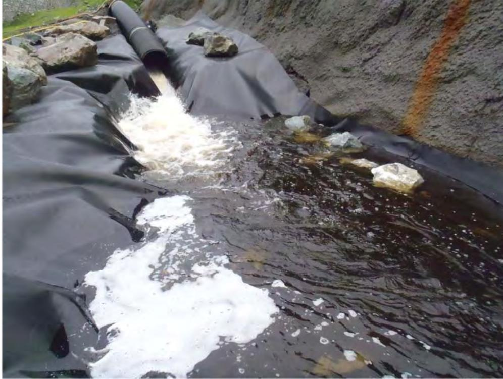
**Figure 4:** Plunge pool into which diverted water spills before entering Lower Slate Creek.
