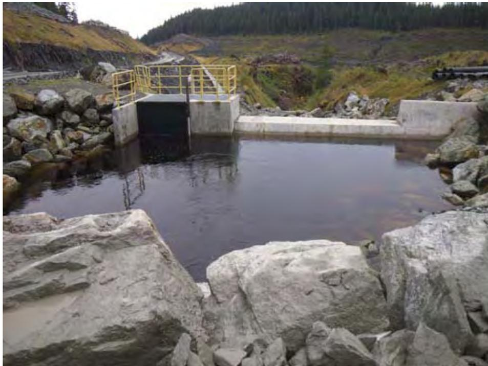
**Figure 3:** Concrete weir and intake structure.
