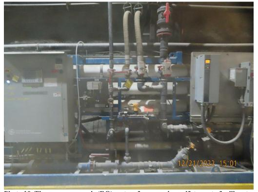
Photo 10. The reverse osmosis (RO) system for removing sulfates out of mill water.
