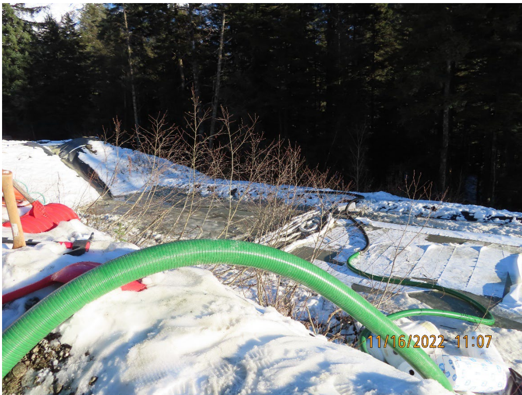
Photo 11. Absorbent pads placed in the Wolf ponds.
