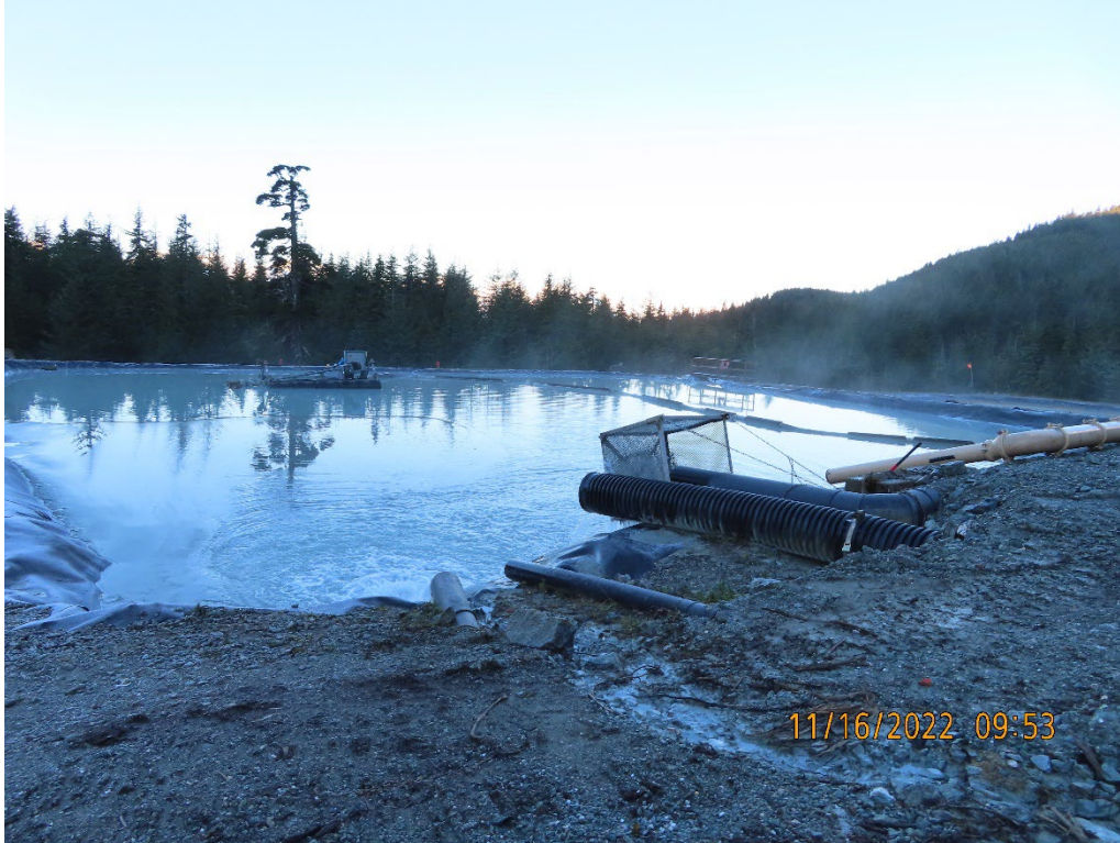
Photo 4. Comet Water Treatment Plant (CWTP) Pond 1.
