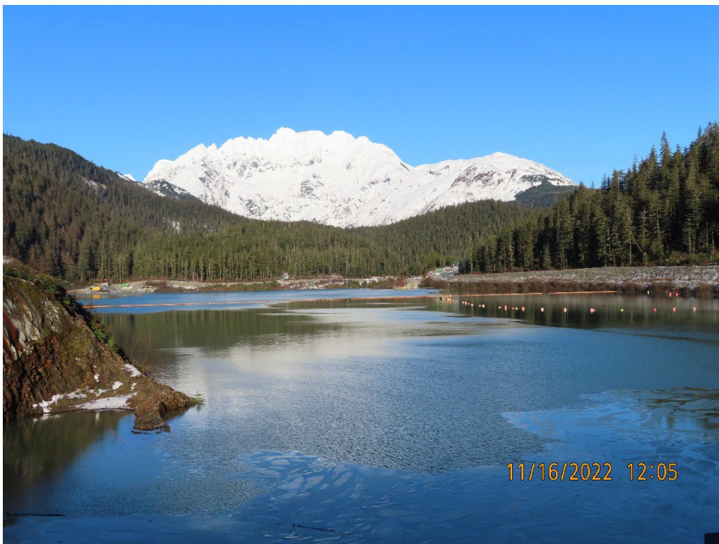
Photo 17. TTF looking north
