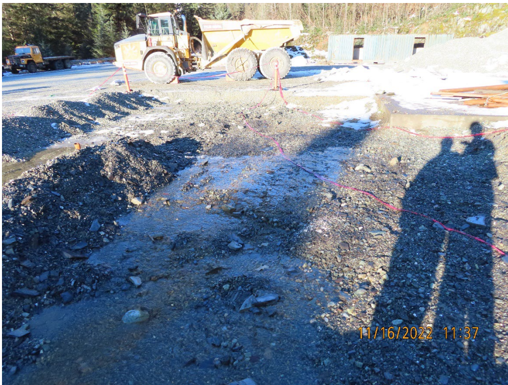
Photo 15. Surface discharge near the abandoned drill casing in Pit 4.
