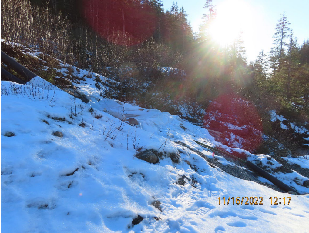
Photo 20. Seepage near the TTF dam access road and constructed containment sump.
