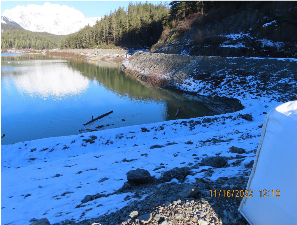
Photo 18. TTF dam face with large woody debris present.
