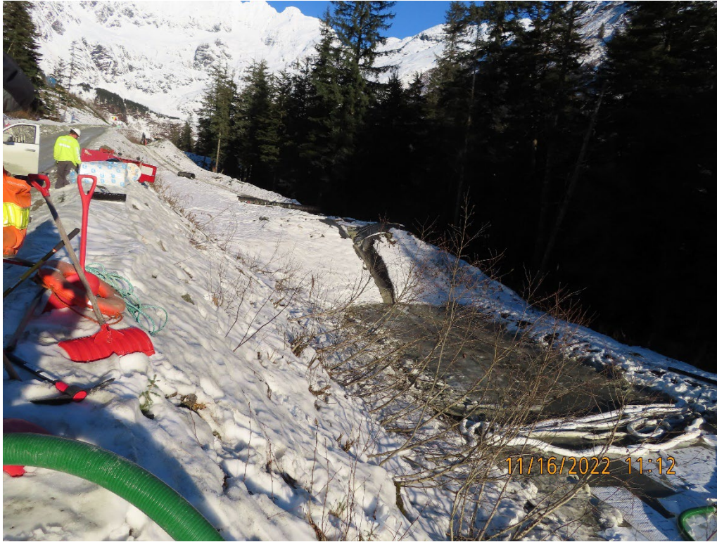
Photo 12. Absorbent pads and boom placed in the Wolf ponds.
