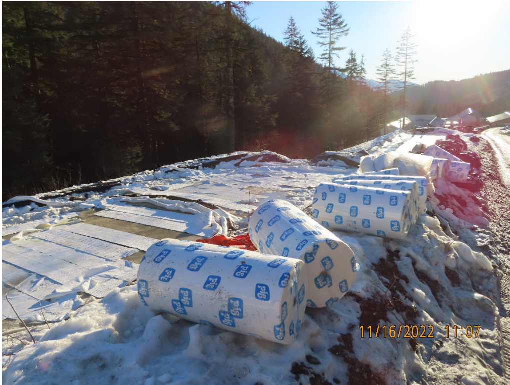
Photo 10. Absorbent pads placed in the Wolf ponds.
