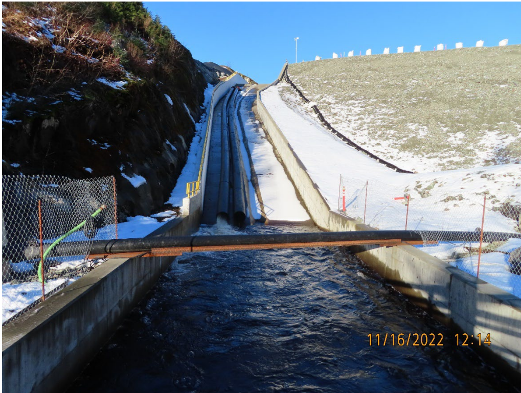
Photo 19. TTF dam spillway.
