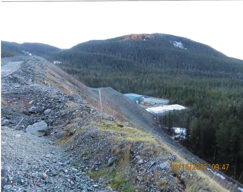
Photo 1. Comet waste rock storage area.
