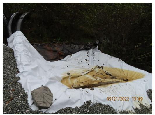
Photo 15. Seepage staining adjacent to lower TTF dam access road and constructed containment sump.
