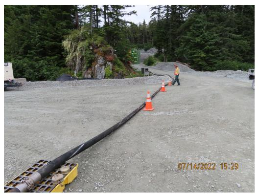
Photo 23. Line connecting the fuel barge to the fuel depot header.
