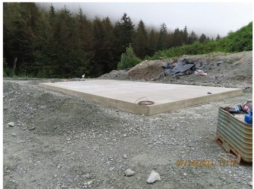
Photo 8. Concrete slab at the north end of the Mud Dump, where the equipment maintenance shop currently located at Pit 4 will be relocated.
