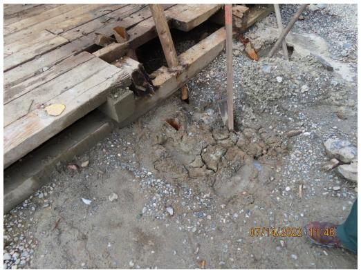
Photo 12. Borehole location at Pit 4 where groundwater had previously been flowing to the surface.
