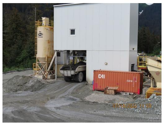
Photo 10. Pug Plant loading an underground haul truck with graphitic phyllite mixed with concrete and aggregate for backfill underground.
