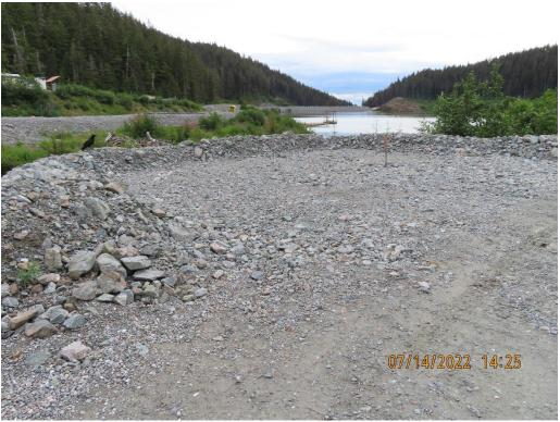
Photo 20. Second drill pad constructed for geotechnical drilling near the Upper Slate Lake bypass intake.
