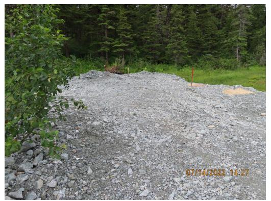
Photo 19. Drill pad constructed for geotechnical drilling near the Upper Slate Lake bypass intake.
