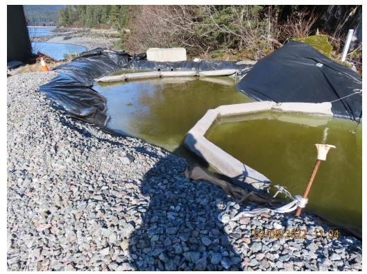
Photo 10. Slate Cove marine facility stormwater sediment BMPs.
