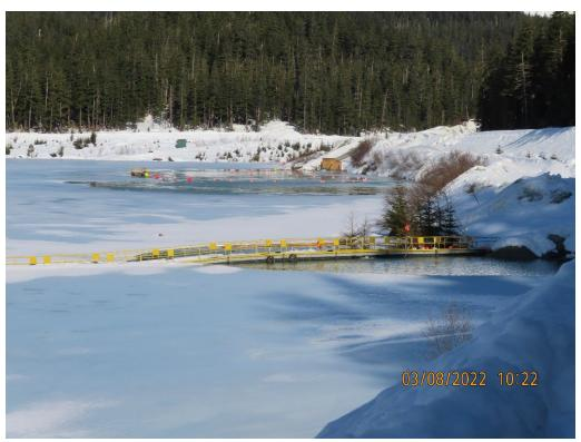
Photo 8. TTF lake. Dark area with open water in foreground is the reclaim barge, tailings deposition area is in the background.
