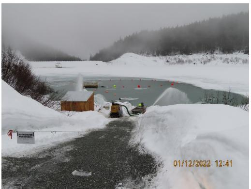
Photo 13. Tailings deposition area showing spraying water used to maintain open water for deposition barge maneuverability.
