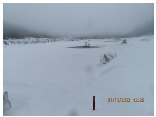
Photo 12. TTF lake. Dark area with open water in foreground is the reclaim barge, tailings deposition area is dark area up and to the right of reclaim barge.
