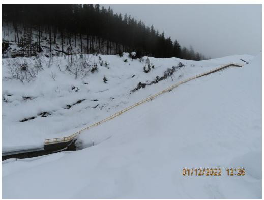
Photo 11. TTF dam spillway with new handrail.
