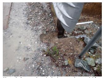
Photo 9. Concern here is the increased potential for erosion at the bridge end.
