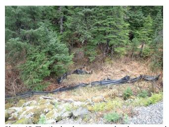
Photo 15. The tire has been removed and new secondary silt fencing was installed.
