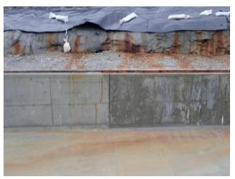
Photo 20. Coeur personnel recently applied additional cement to the spillway walls to indicate if any new ARD generation has breached the wall.
