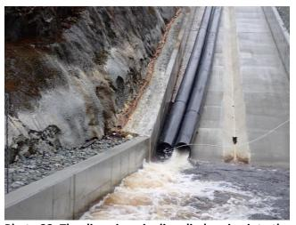
Photo 22. The diversion pipeline discharging into the dam spillway.
