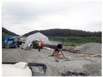
Photo 12. Coeur Alaska personnel fusing together sections of HDPE pipe.
