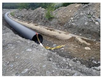
Photo 13. The fused HDPE pipe is being routed to the stage 3 dam.
