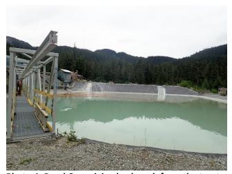
Photo 4. Pond-2 receiving backwash from the treatment plant.
