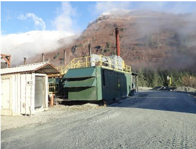
Photo 9. The old generator/new pug plant site.
