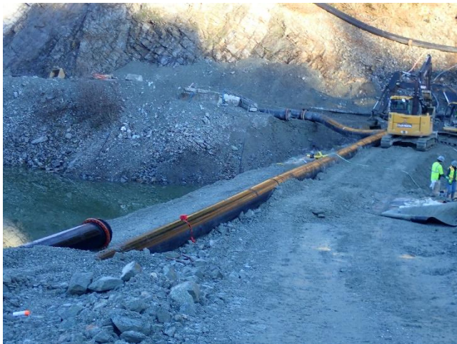
Photo 15. Upper Slate Lake diversion pipeline will have two 28-inch pipes.
