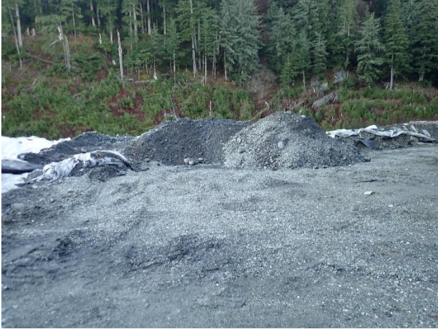
Photo 17. GP material staged in the northern TTF area.
