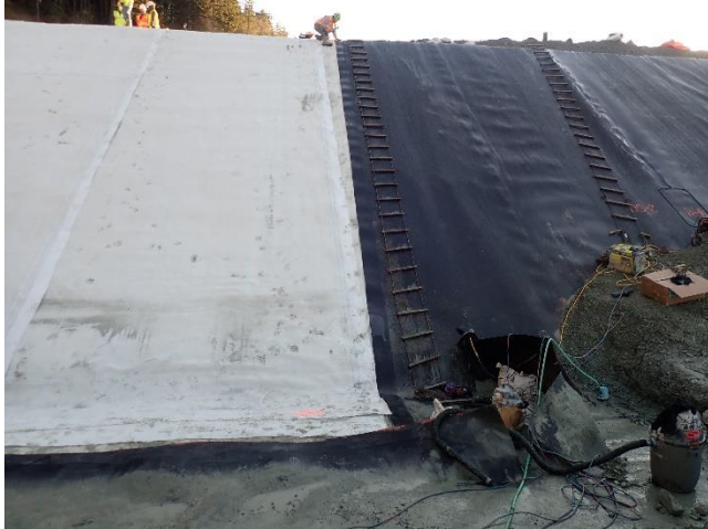
Photo 14. Stage 3 dam liner installation.
