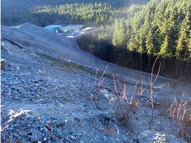
Photo 2. Comet Development pile.
