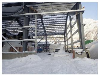
Photo 9. Contractors continue with the construction of the powerhouse steel structure.
