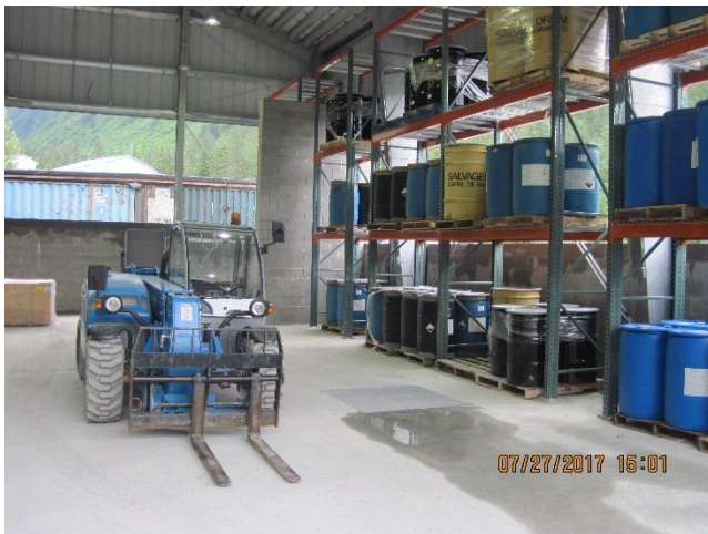
Photo 20. Image shown here is steel shelving that was installed in the chemical cold storage warehouse.
