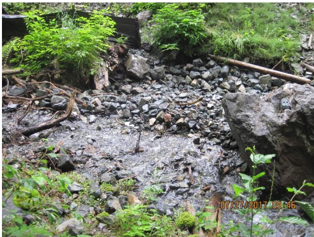
Photo 6. Riprap placed along the cut bank of Ophir Creek.
