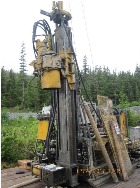
Photo 17. Geo-tech drill BH-006.
