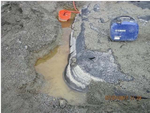
Photo 11. The hand dug trench at the Mud dump.
