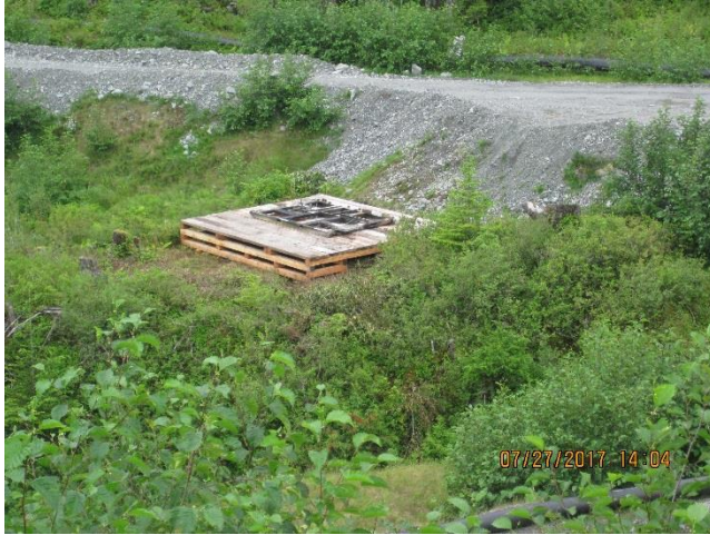
Photo 18. A constructed drilling pad located in the northern TTF area.
