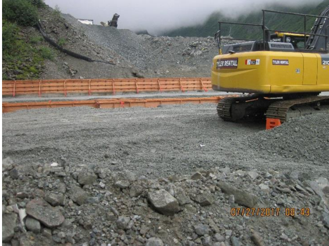
Photo 10. Image shown is the construction for the concrete foundation pad.
