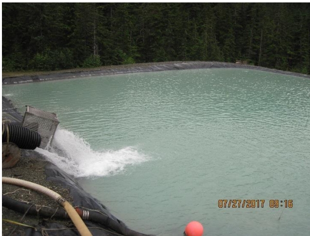
Photo 2. Image shown is Pond 1 at the Comet water treatment plant.
