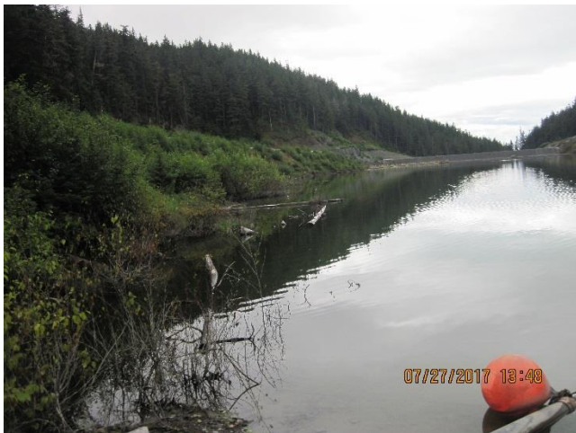
Photo 15. The Tailings Treatment Facility (TTF).
