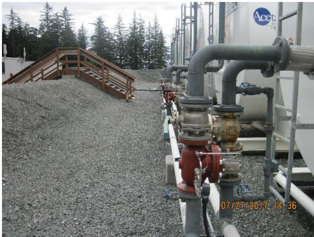
Photo 19. Coeur Alaska's fuel depot.
