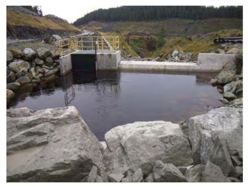
Figure 3: Concrete weir and intake structure.
