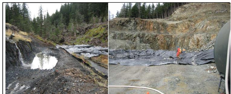
PHOTO 5. TREATED SEEP WATER. PLUNGE POOL BEYOND, NEXT TO DIRT BAG.
