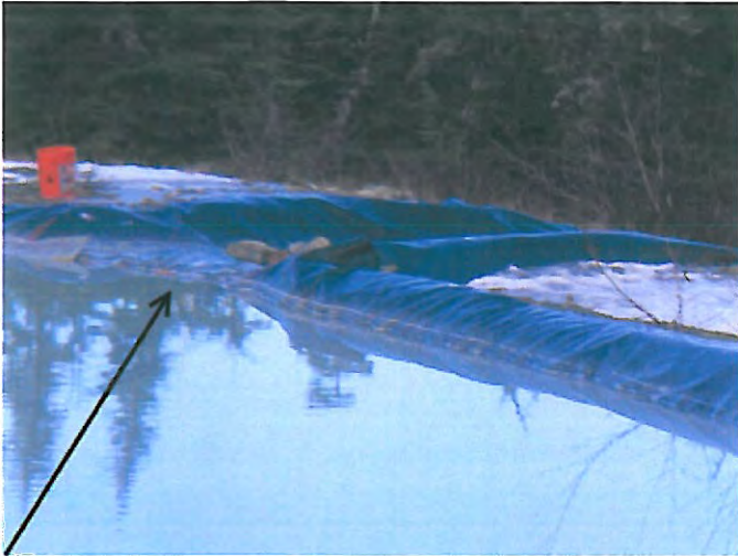
PHOTO 7: CLOSER VIEW OF SPILLWAY FROM POND 1 TO POND 2
