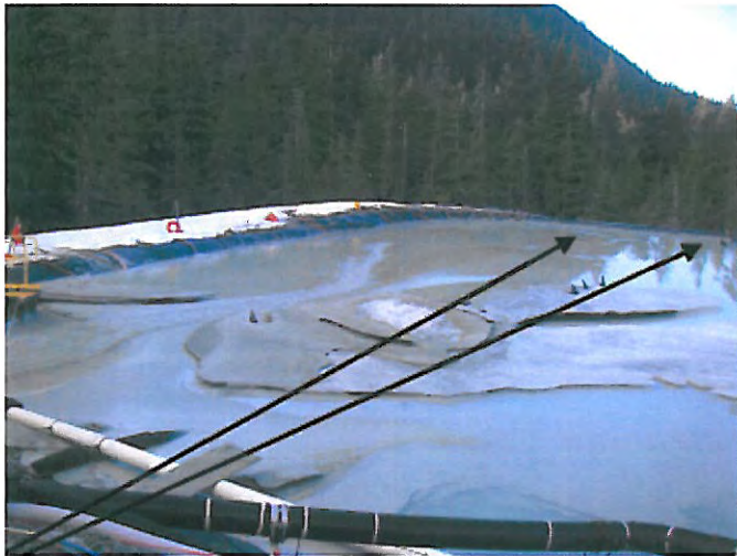
PHOTO 3: POND 1 APPEARS TO HAVE EXTREMELY LIMITED FREEBOARD AVAILABLE
