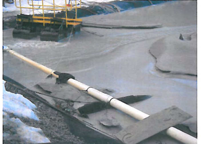
PHOTO 4: WASTE ACCUMULATES AROUND PERIMETER OF POND 1 IN SOME AREAS
