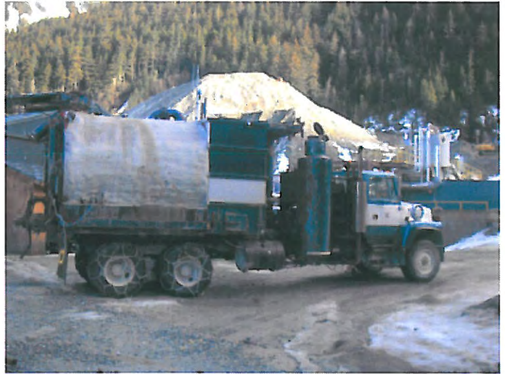
PHOTO 8: "PUMPER TRUCK" USED TO REMOVE SEDIMENT FROM POND 1
