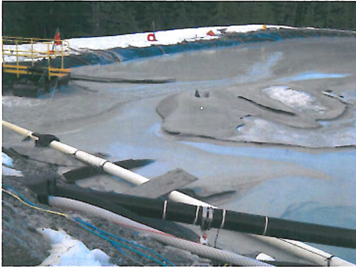
PHOTO 1: ACCUMULATED SEDIMENT IS VISIBLE ON SURFACE OF POND 1
