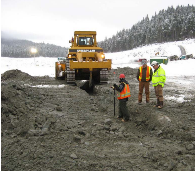
PHOTO 3. TRENCH FOR PIEZOMETER
