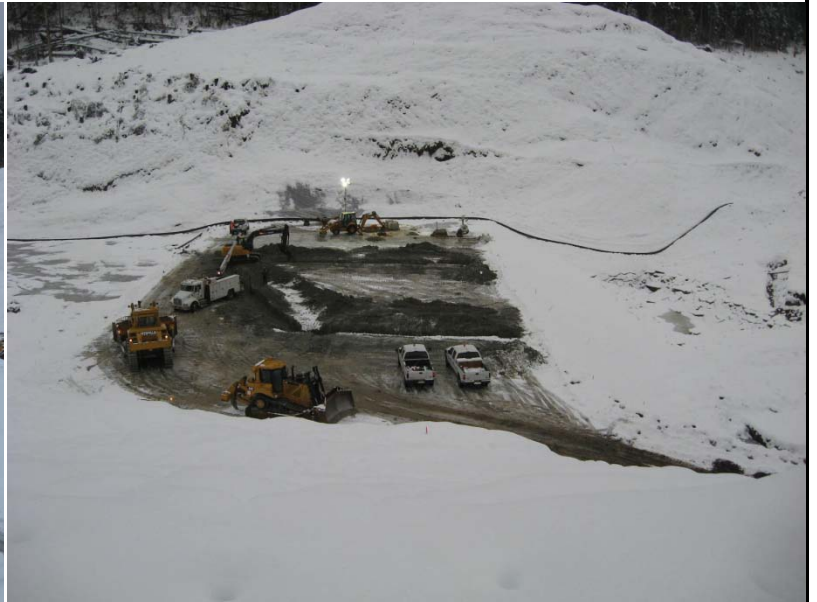
PHOTO 2. DAM FROM EAST EMBANKMENT
