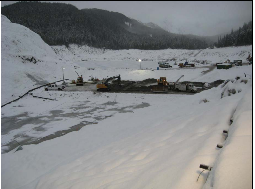
PHOTO 6. DAM AND IMMEDIATELY DOWNSTREAM OF THE DAM
