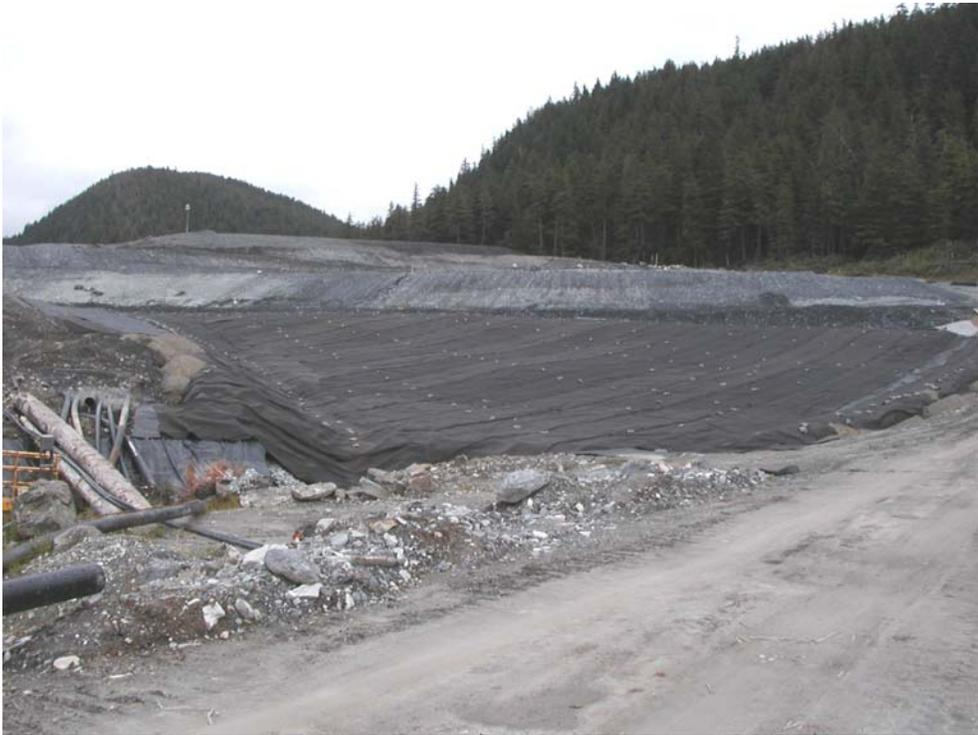
FIGURE 2.35 Southeast Expansion Liner Phase II: July 11, 2005
