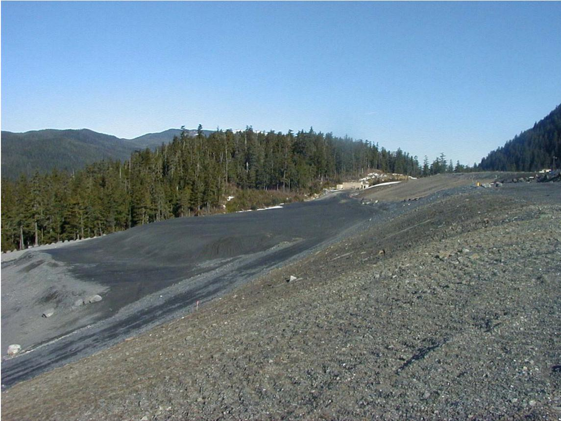
This photograph is a view of the West Buttress placement looking north. Tailings are placed in cells and the 3H:1V outer slope is covered with Class 1 production rock or native materials to minimize erosion.
