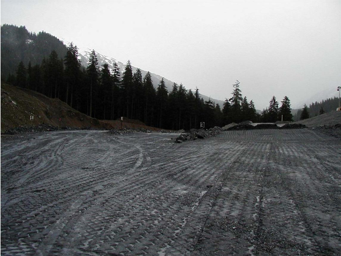
The photograph shows the designated placement zones (Class 1, left; Class 2, center; Class 3, right). Marks from the grid roller are visible on the recently spread and compacted production rock surface. The view is looking east.
