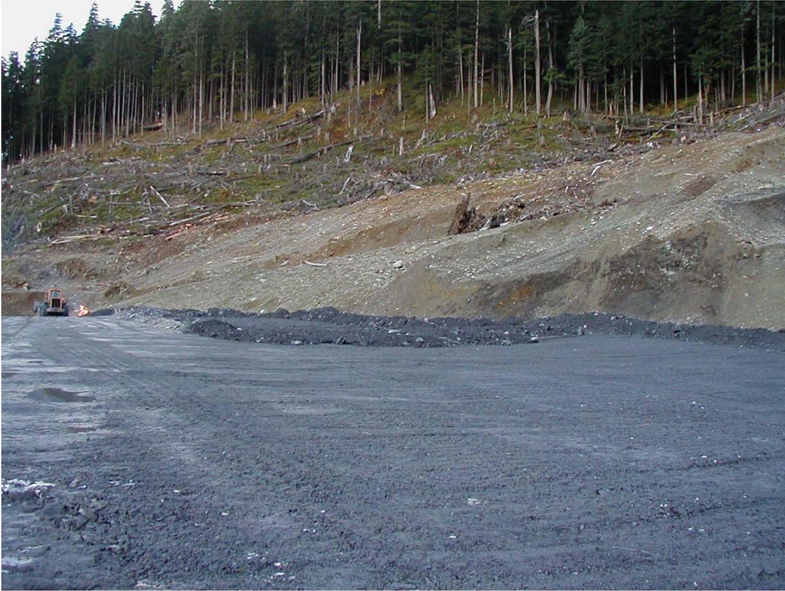
This photograph shows construction of the pile base. Native rock and sediments are removed from the back slope and stockpiled for use in future reclamation projects. Continuation of finger drains (not visible) extend over the prepared surface and a five-foot thickness of Class 1 production rock is placed prior to placement of other classes.
