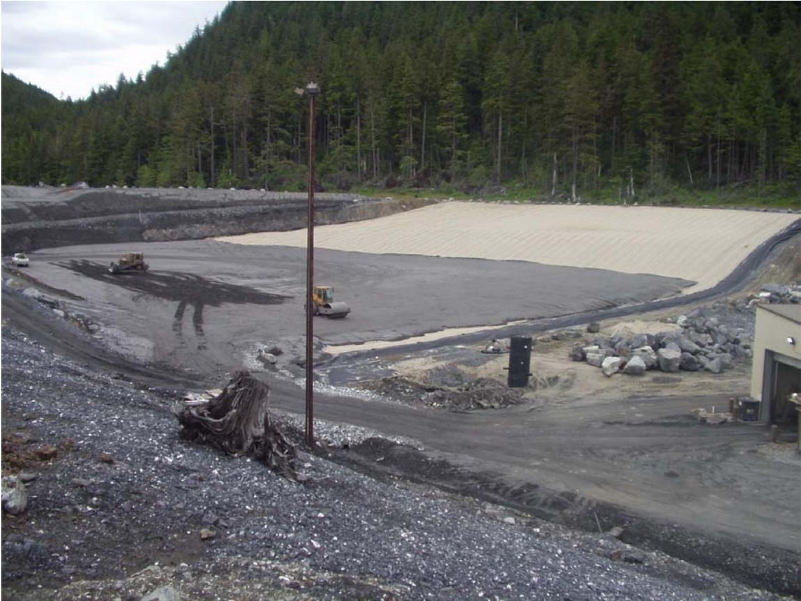
Initial tailings placement in the Southeast Liner Tailings placement area. Tailings are spread in thin lifts with a bulldozer (left) and compacted with a vibratory roller (middle). Ramps (center) provide access to the wheel wash located near Tank 6 (Figure 2.33).
