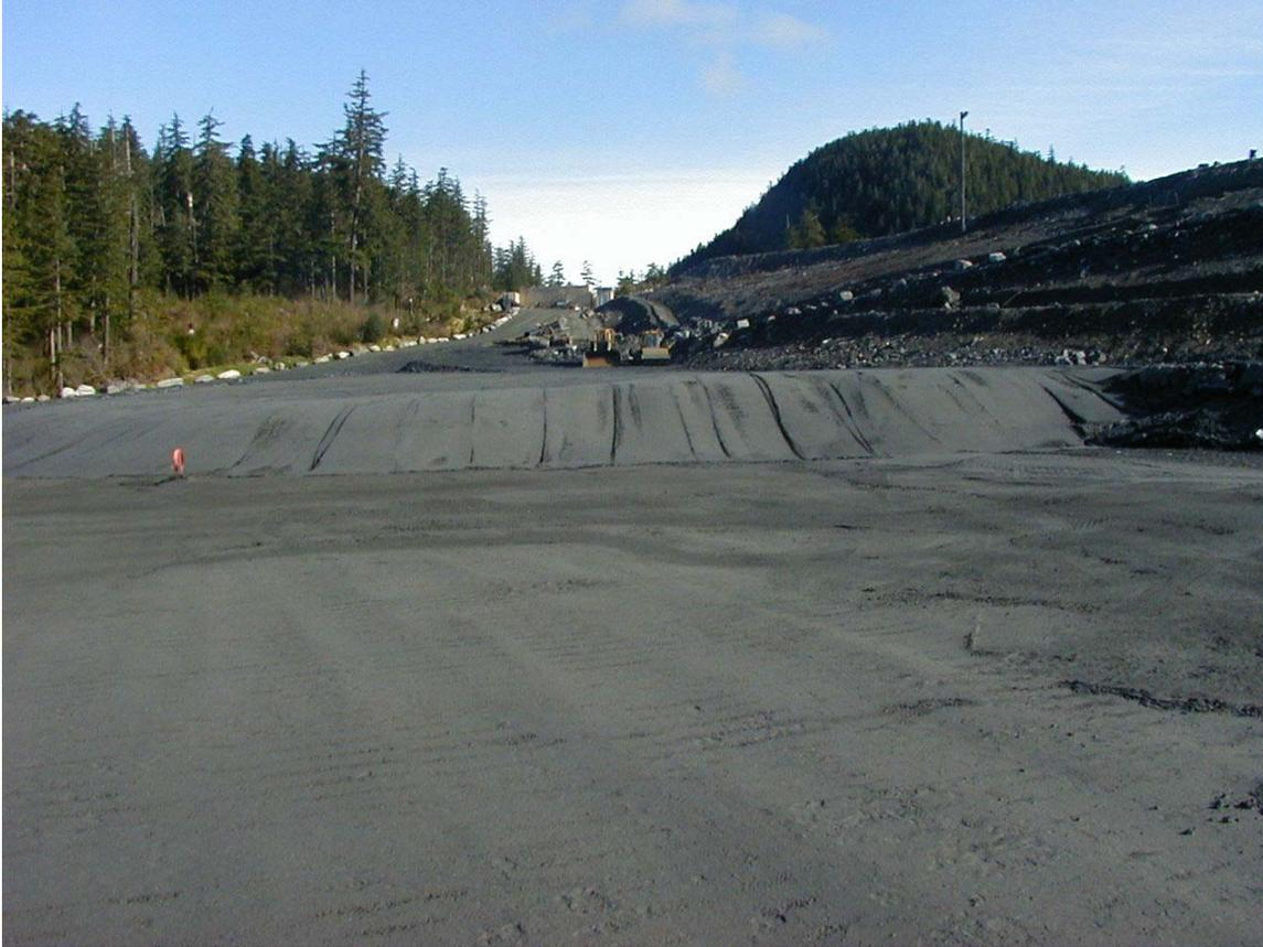
View of compacted tailings in the West Buttress placement area. The tailings are spread and compacted in thin, inclined lifts in a cell that has an overall thickness of approximately five feet. This promotes drainage and dissipation of pore pressures that rise as the material is compacted. 12% of the overall placed tails for 2002 were put into West Buttress.
