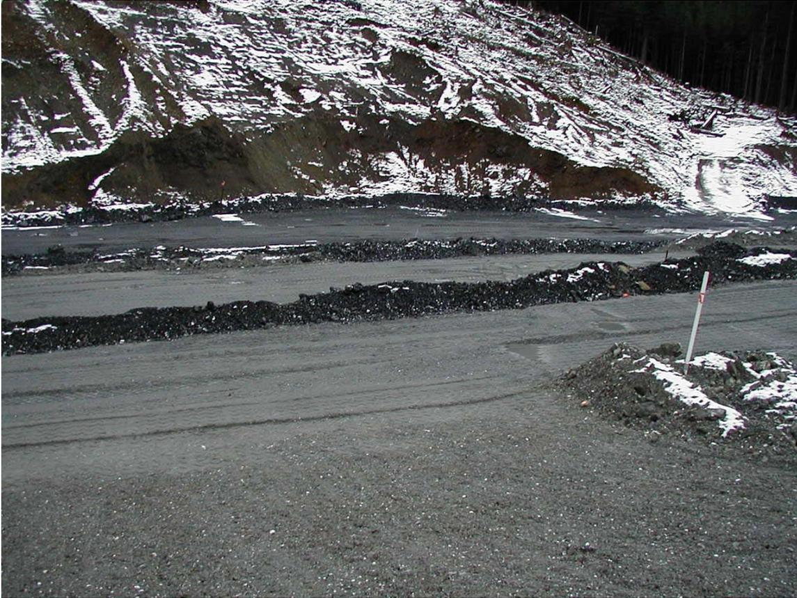
The three designated placement zones are visible in the lower half of the photograph. Class 3 in the foreground, Class 2 at center and Class 1 at base of backslope. Safety berms are left between the placement zones. Excavated material from the backslope (upper half of photo) will be used for site reclamation. Monitoring well MW-23-98-01 is visible in the foreground (right). The view is oriented north.
