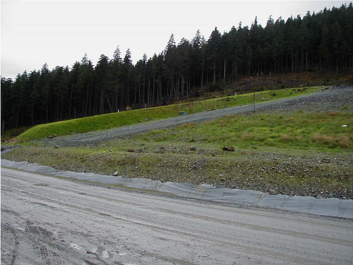
The photograph shows the recently seeded composite soil cover placed on the lower slope of Site 23. A portion of the lower capillary break is visible below the seeded growth layer. The B Road and lined ditch that brings surface waters to Pond 23 are visible in the foreground.
