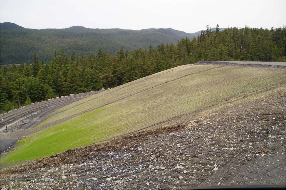
Figure 2.35 Hydroseeded West Buttress July 7, 2004
