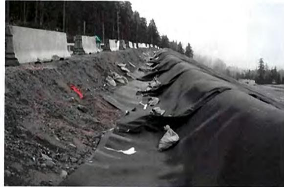
**Upper Liner Anchor Trench – B-Road prism**
