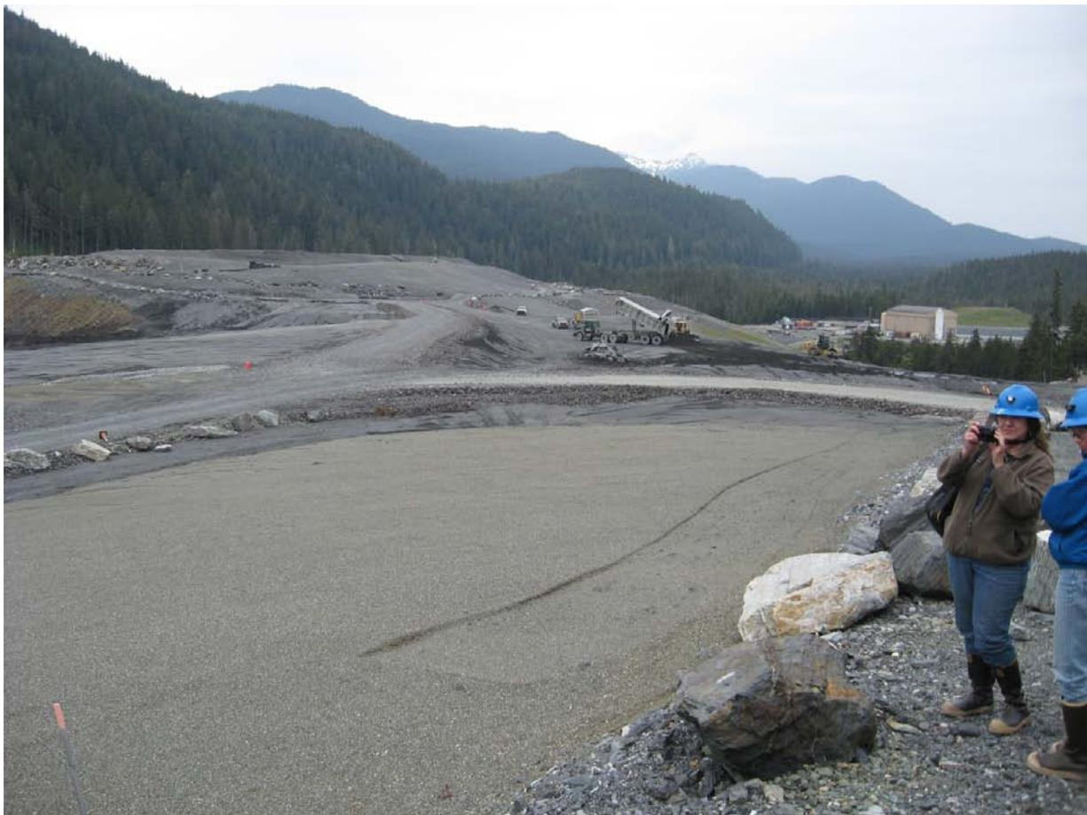
Tailings site; active placement, spreading and rolling under way.
