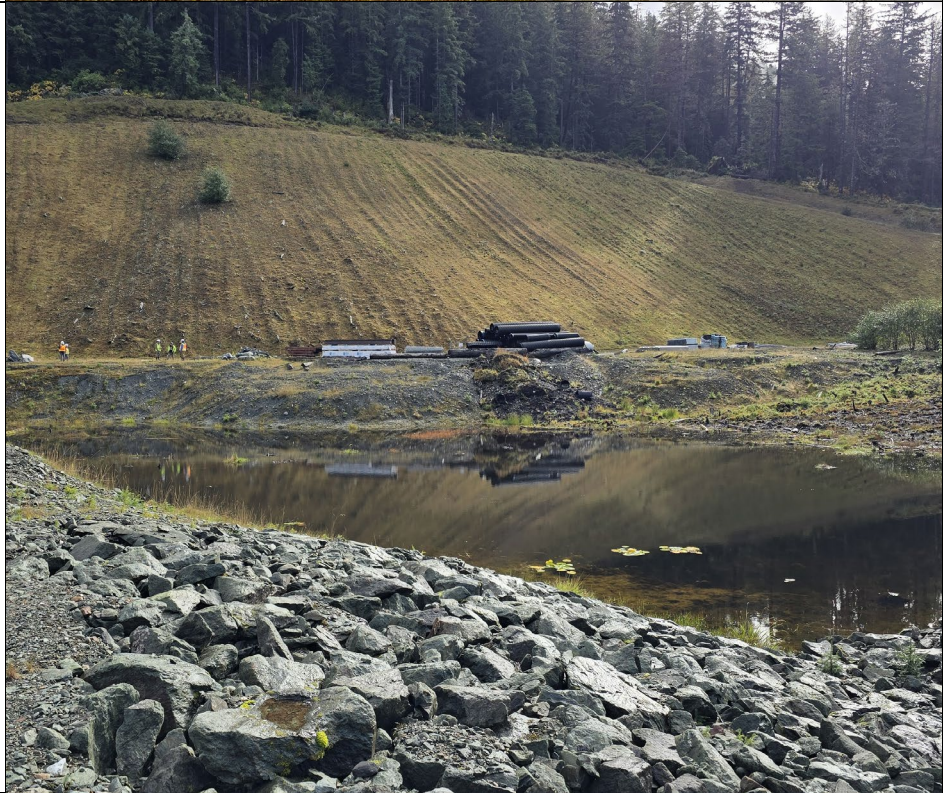
Photo 10: Poned water within Sand Pit observed below the spillway. View of the well vegetated slopes on the eastern side of the facility.
