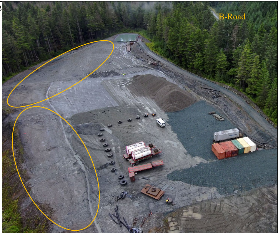
Photo 5: Aerial view looking west. Partial grading along the western and northern edges of Site E (Circled). Storm water drainage pond near capacity at the far end of the facility. Site E is used as a laydown yard and storage facility.
