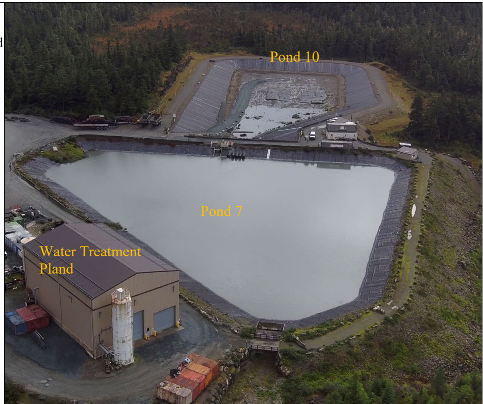
Photo 17: Water storage capacity at Pond 7 is just below culverts that are piped to Pond 10. Ariel view looking south.
