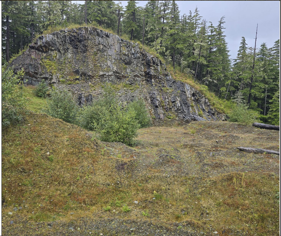
Photo 8: Vegetated slopes leading up to the old rock quarry highwall at Pit 7.
