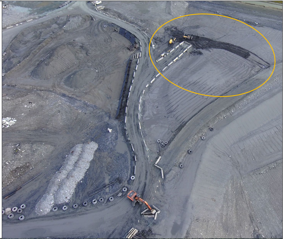
Photo 11: Active tailings deposition atop the TDF using a dozer and roller (Circled). Excavator placing Jersey barriers along access road. Ariel view of the central eastern end of the TDF.
