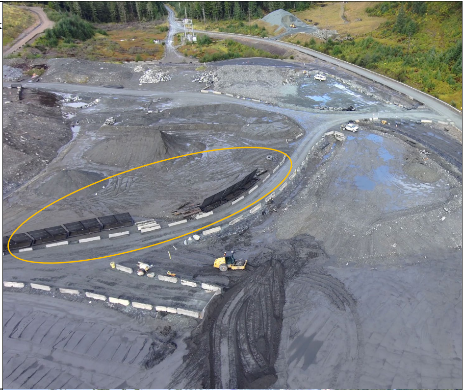
Photo 13: Wind fencing installed along the haul truck access route and eastern TDF edge (circled) to help mitigate fugitive dust.
