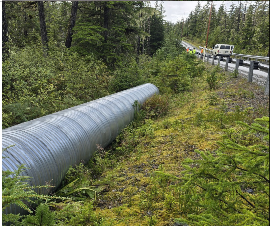
Photo 20: Delivered replacement culvert at MP 2.2 along A-Road for future fish-habitat improvements.
