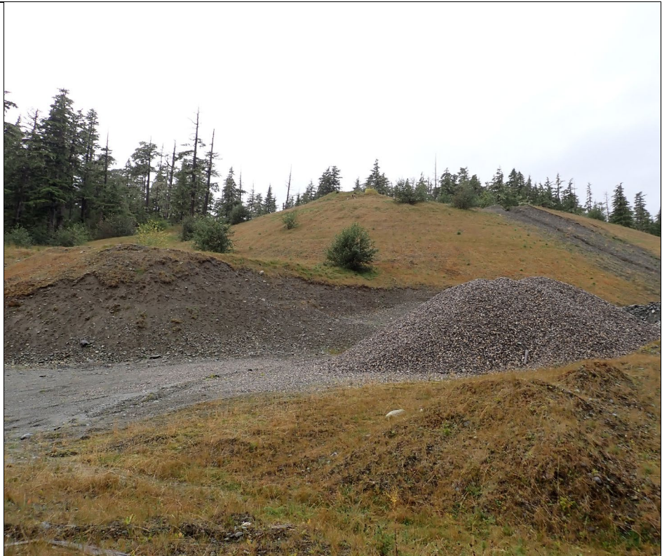
Photo 7: Excavated and stabilized toe of the slope at Pit 7 to enlarge the pad area for aggregate storage. Sloped areas have good vegetative coverage. View looking to the west.
