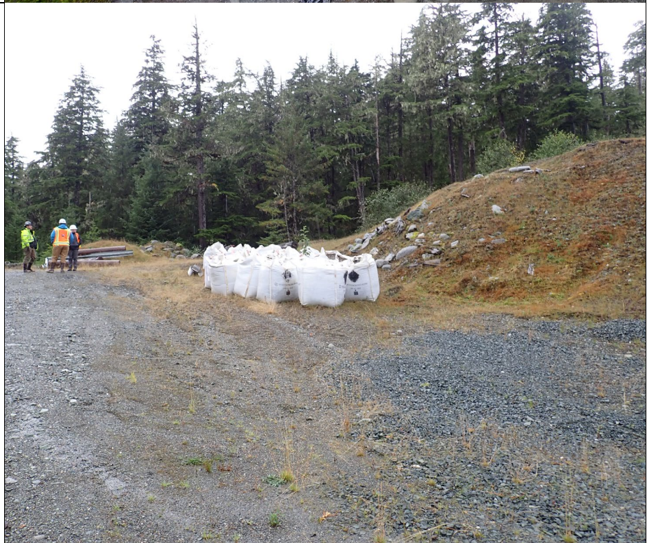
Photo 6: Stockpiled aggregate, super sacks, and metal piping stored at Pit 7. View looking south.
