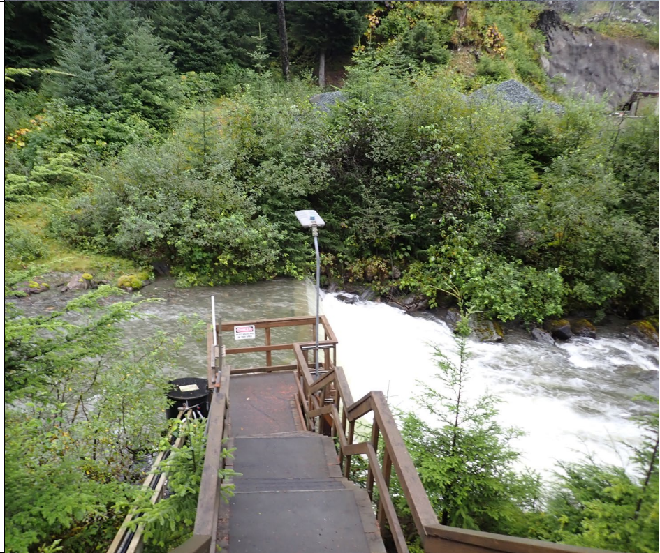
Photo 16: Potable Water Treatment facility next to water draw point near the 920 Portal with maintained walkways to Greens Creek used for water sampling.
