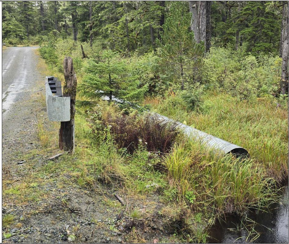
Photo 21: Delivered replacement culvert at Pit 7 access location for planned habitat upgrades.
