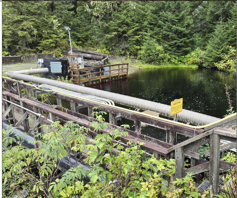
Photo 18: Potable water draw point for Hawk Inlet Camp facilities is well maintained. This area is just off the B-Road along Cannery Creek.
