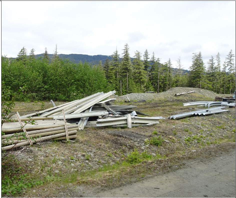
Photo 5: Sand Pit laydown yard with stored culverts, piping, and construction materials. Viewed near the entrance looking northwest.
