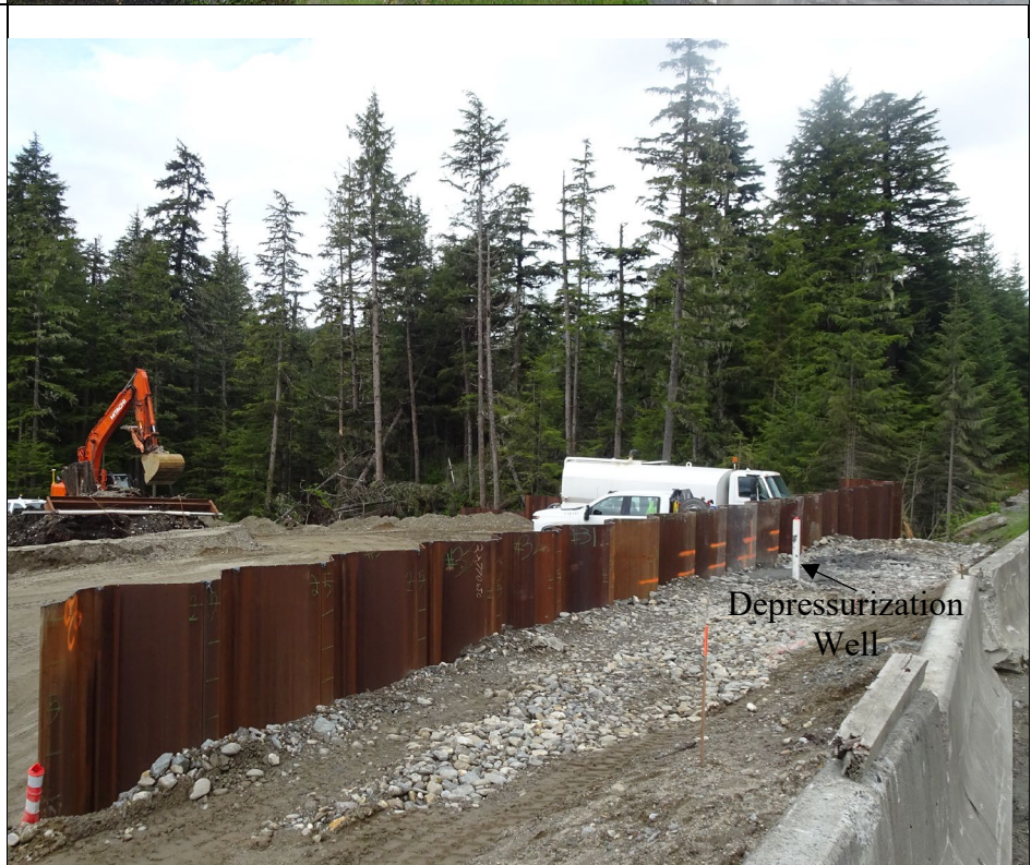
Photo 8: Completed cut-off wall near B-Road for groundwater control.
