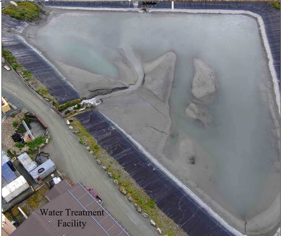
Photo 22: Pond 7 Inlet exhibiting incising into sediment delta .
