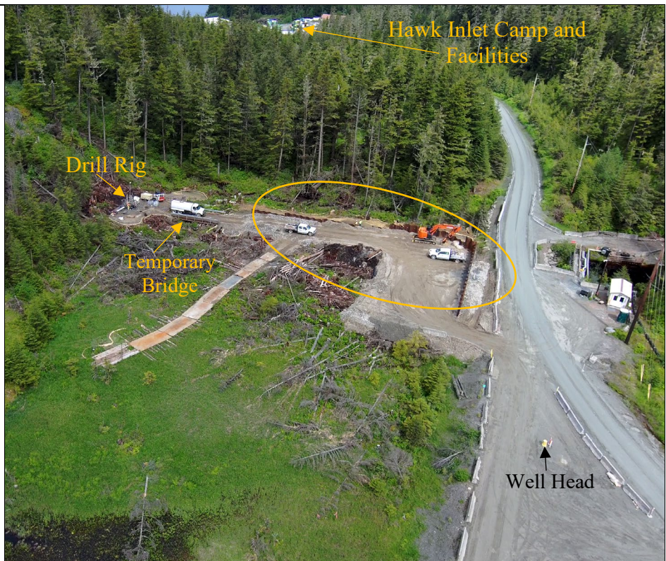
Photo 7: Northern aerial view of the TDF expansion. Active drilling across from the temporary bridge for installation of a depressurization well. The extent of the cut-off wall is circled.
