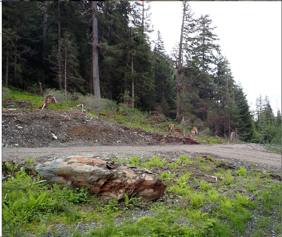
Photo 10: New pad at the junction of A- and B-Roads cleared to construct the new power station. View is to the southeast.
