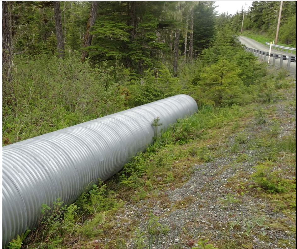
Photo 19: Replacement culvert staged at MP 2.2 of A-Road awaiting installation.
