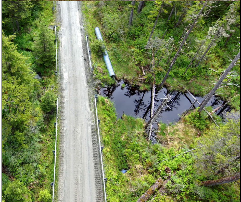
Photo 20: Replacement culvert staged at MP 1.8 just off Pit 7 access road awaiting installation.
