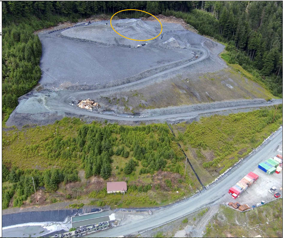
Photo 17: Aerial view looking north of Site 23 Waste Rock Storage. Recent deposition of waste rock was observed on top of the facility (circled). Well-established revegetation has occurred along the base of the facilities southern facing slopes.
