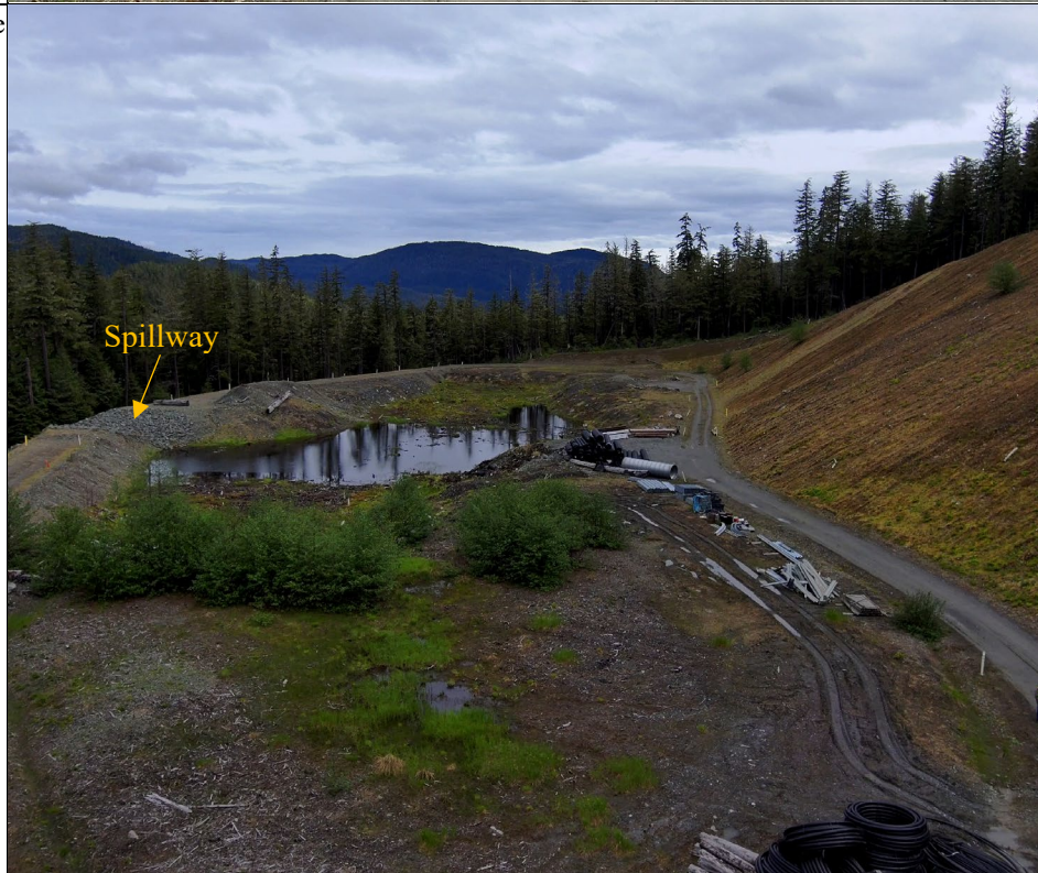
Photo 6: Pondered water in the Sand Pit basin below the spillway elevation. Spillway drains into ditch along A-Road. Well established vegetation on contoured slope. View looking north.
