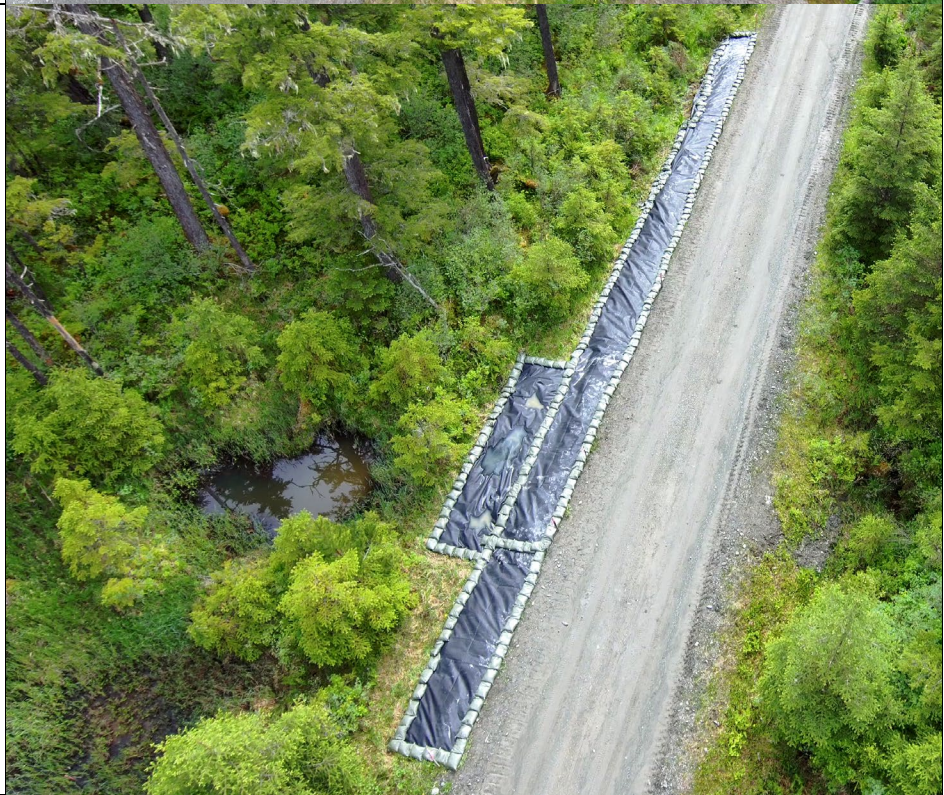
Photo 4: Invasive species BMP's near Pit 7 entrance, using black plastic sheeting pinned with sandbags.
