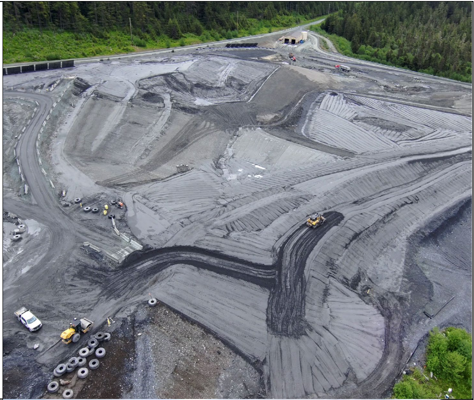
Photo 11: Active tailings deposition with dozer spreading material to build a new lift within the TDF. Aerial view to the southeast.
