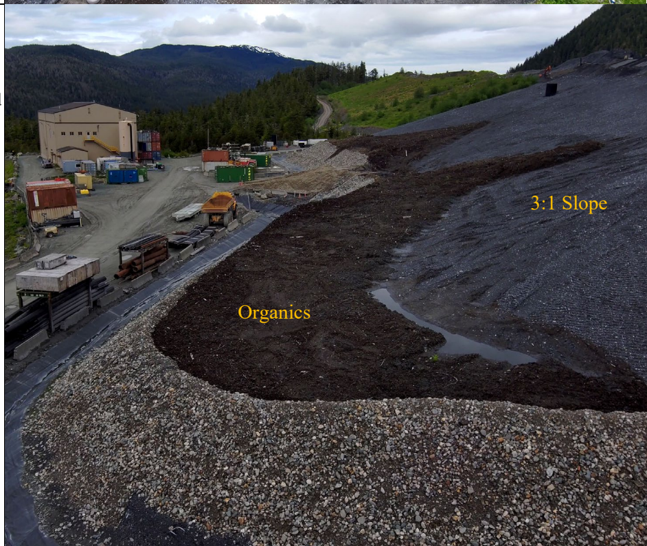
Photo 12: Final grade along the western TDF slope. Fresh organics have been placed on lower slope contours just above the lined stormwater ditch.
