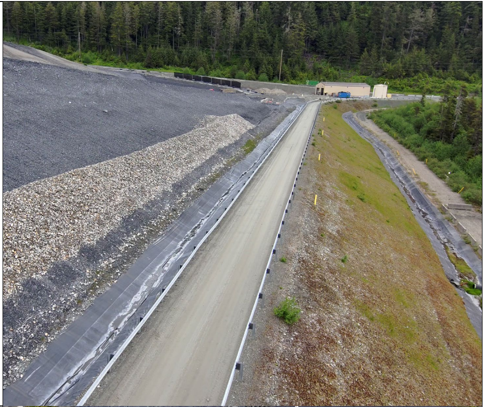
Photo 21: Lined stormwater ditches around the TDF. Aerial view looking to the east.
