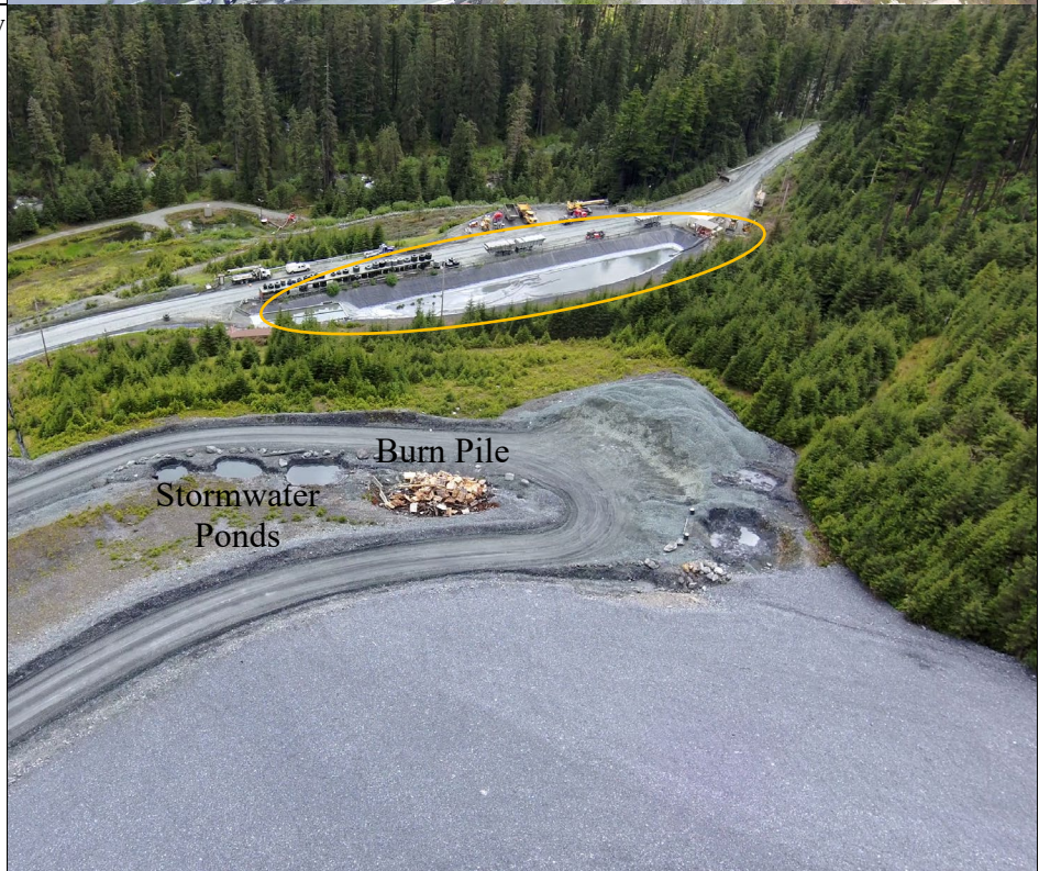
Photo 18: Site 23 aerial view to the south looking at stormwater ponds and staged wood debris planned for burning. Site 23 Water management pond can be seen in the background (circled).
