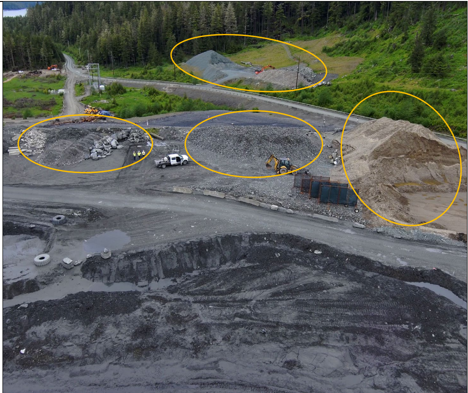
Photo 13: Organized material sites (circled) near the northeastern TDF and along B-Road, used for road construction and base material for TDF expansion area. Aerial view to the north.
