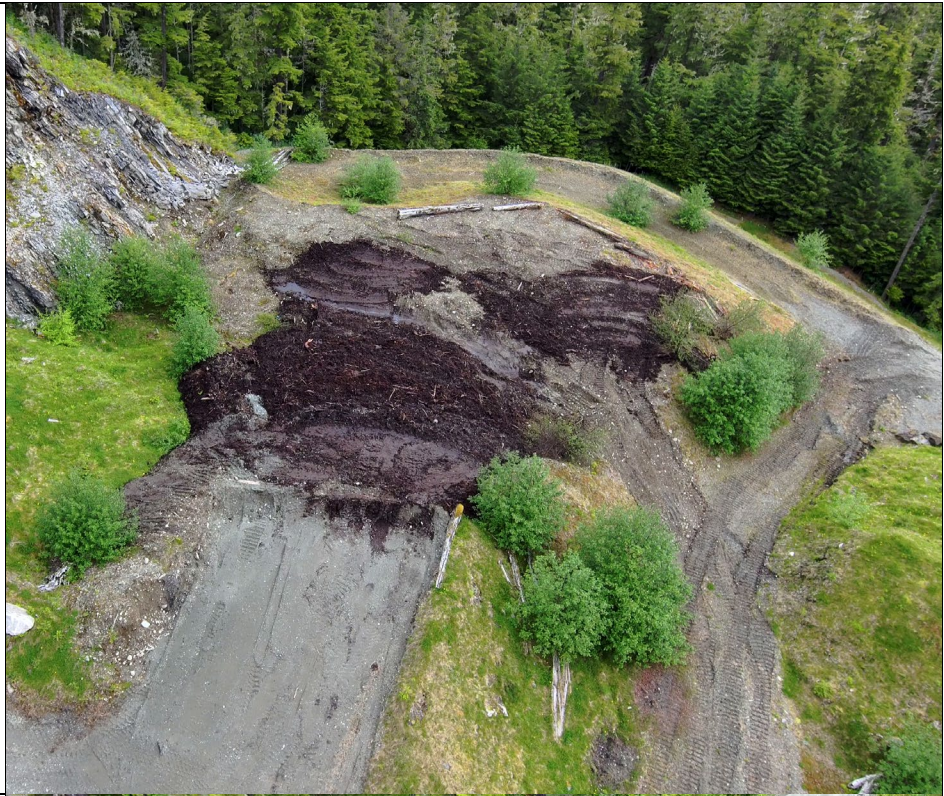
Photo 3: Stockpiled peat excavated from the TDF expansion, stored below the highwall of Pit 7.
