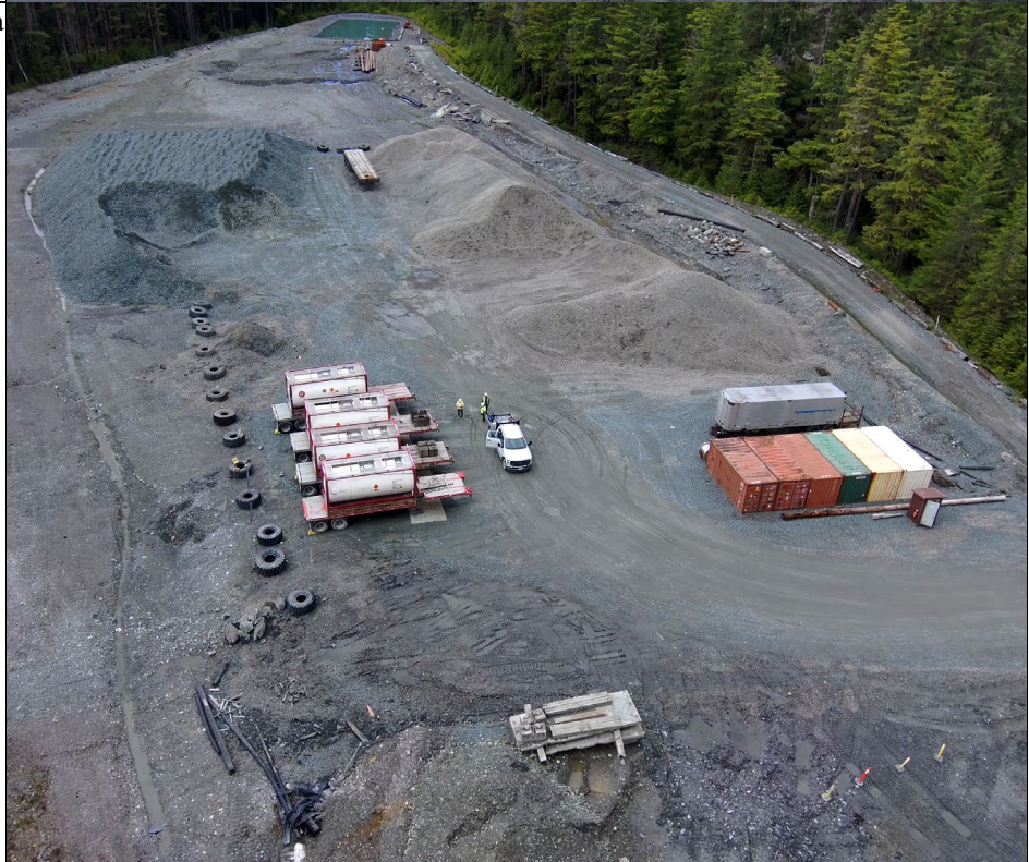
Photo 14: Site E storage area with aggregate, equipment, and explosives.
