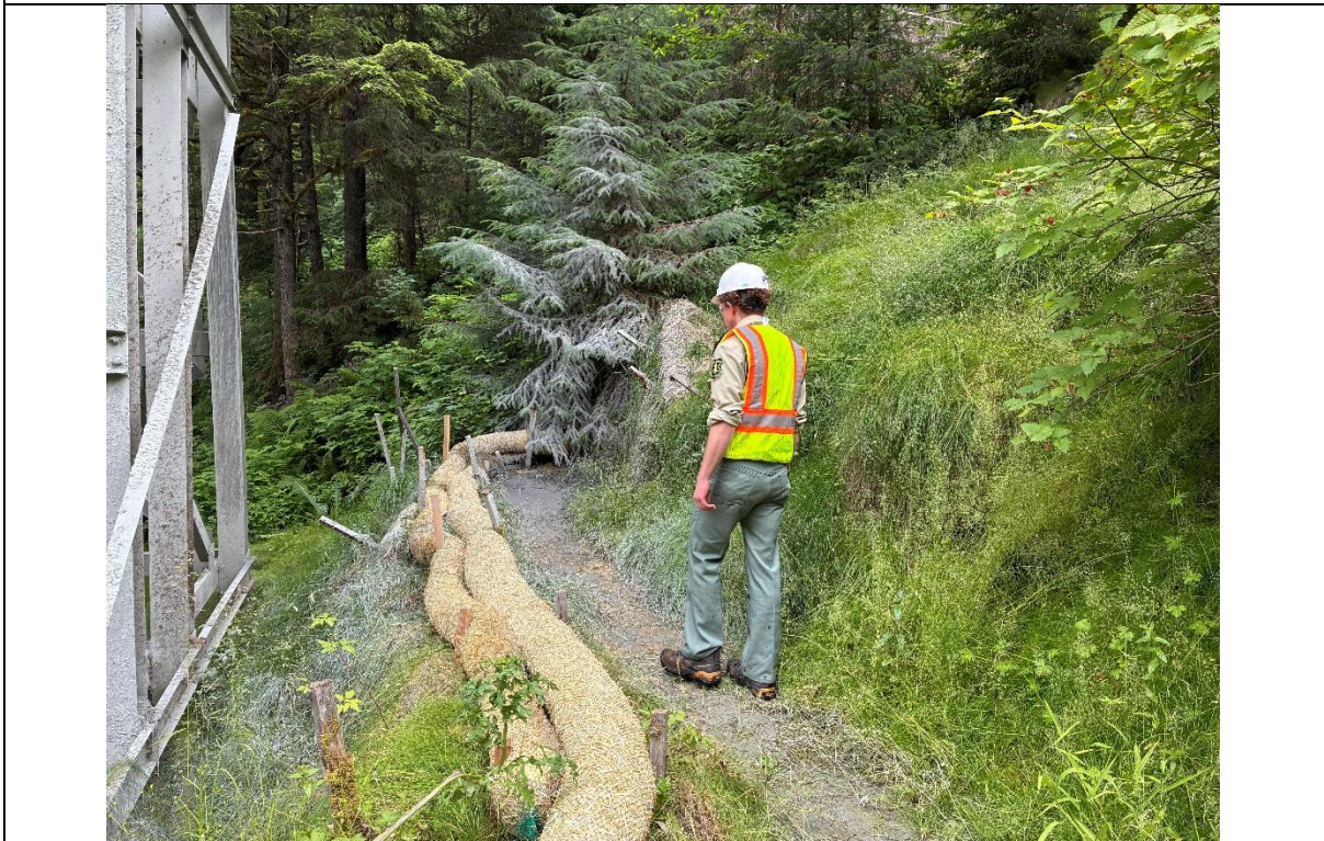
Photo 28: 3.0 Mile B-Road Bridge (Zinc Creek) sediment collected before decking replacement.
