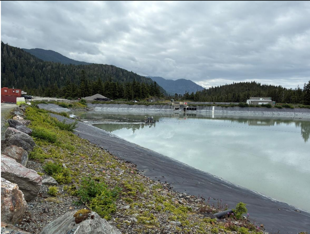
Photo 35: Pond 7 dredge working to pump tails to Pond 10 and into dewatering bags.
