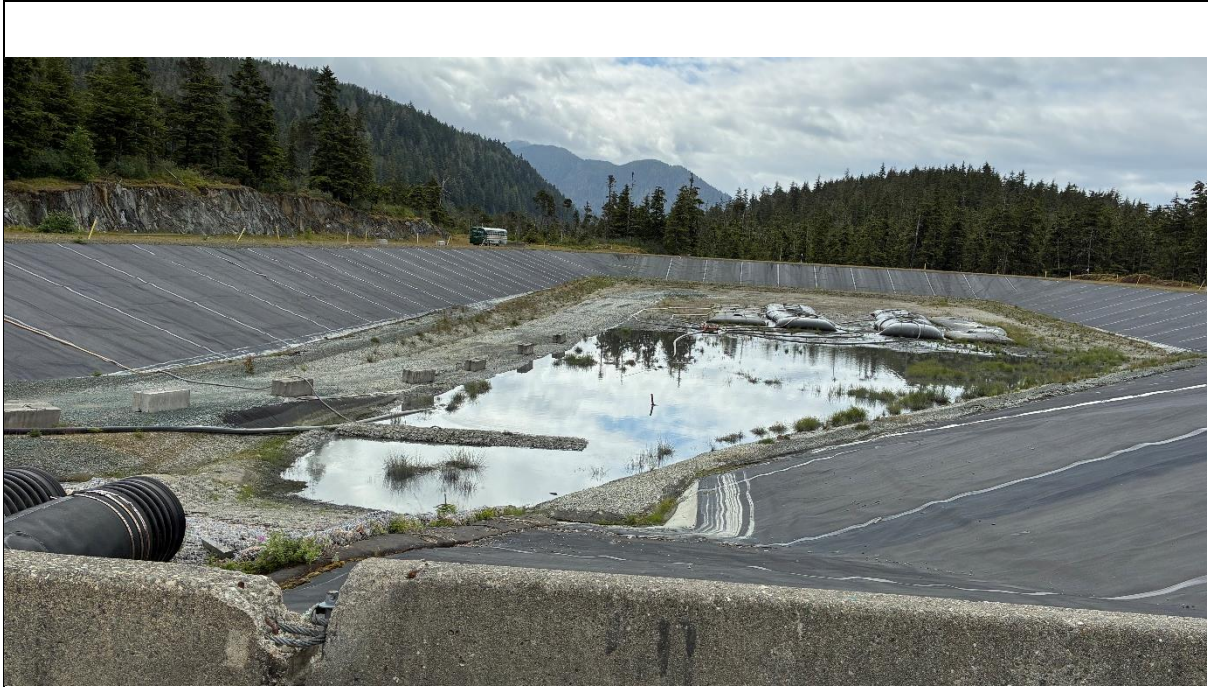
Photo 37: Overview of Pond 10 with tails dewatering bags being filled from dredge in Pond 7.
