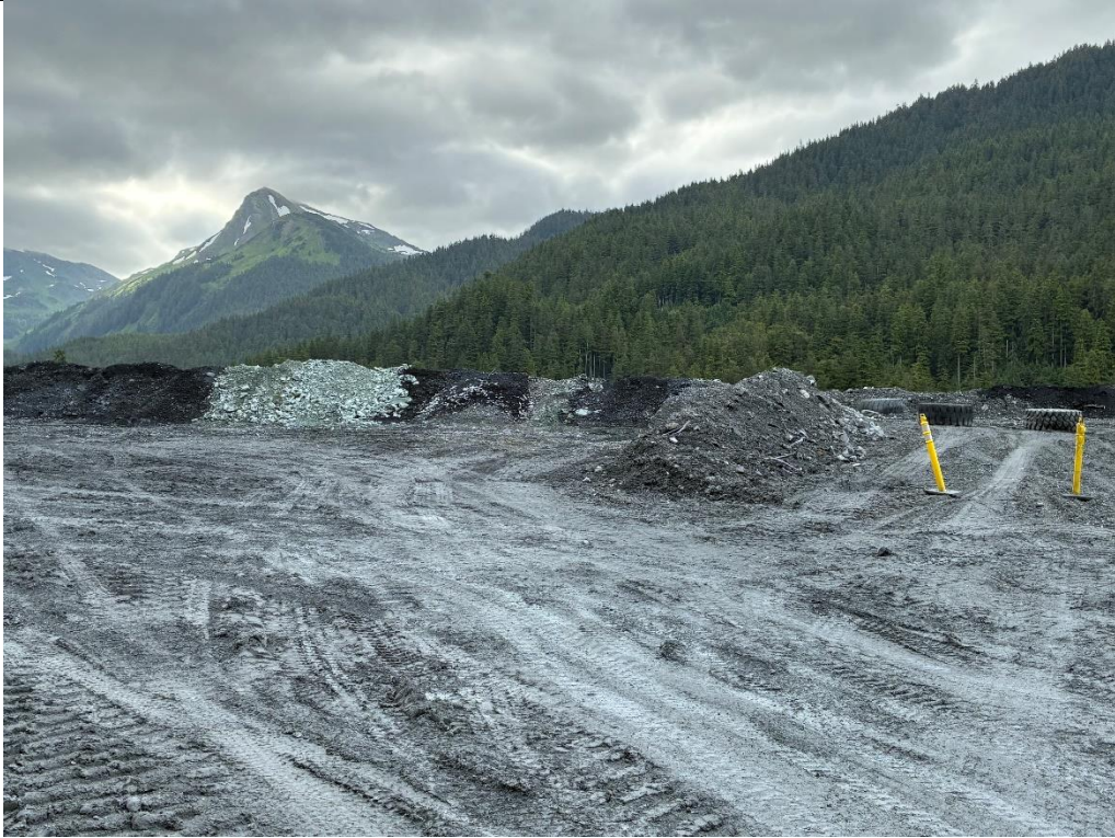
Photo 11: Site 23 Class 2 & 3 Material on top of storage area.
