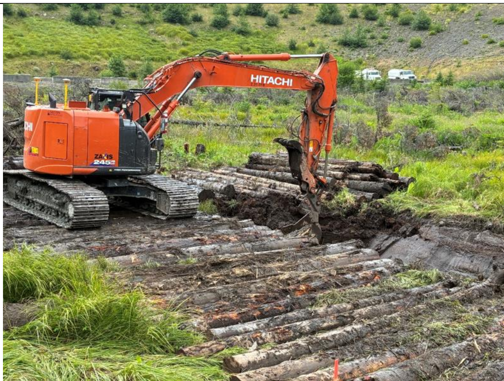
Photo 40: Trenching for dewatering of the NEP. Excavator utilizing corduroy road for minimal ground disturbance.
