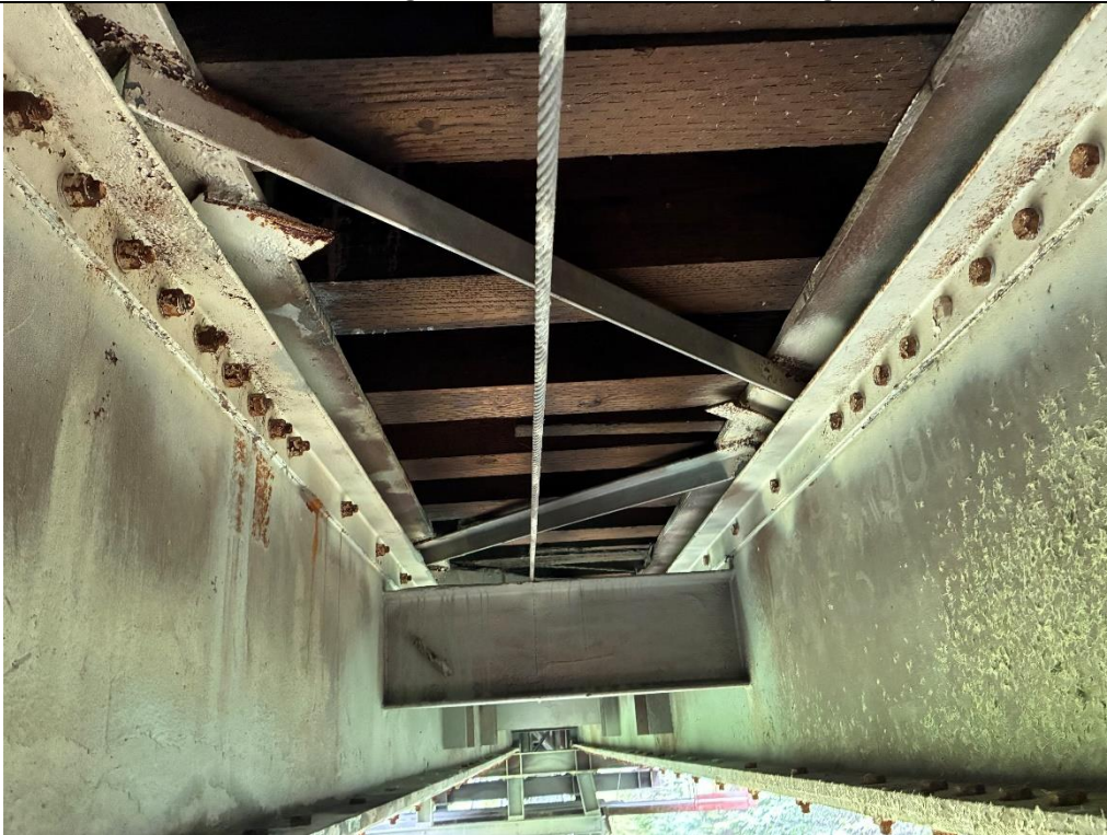
Photo 30: 3.0 Mile B-Road Bridge (Zinc Creek) Center area looking north, the bridge does not appear to be leaking.
