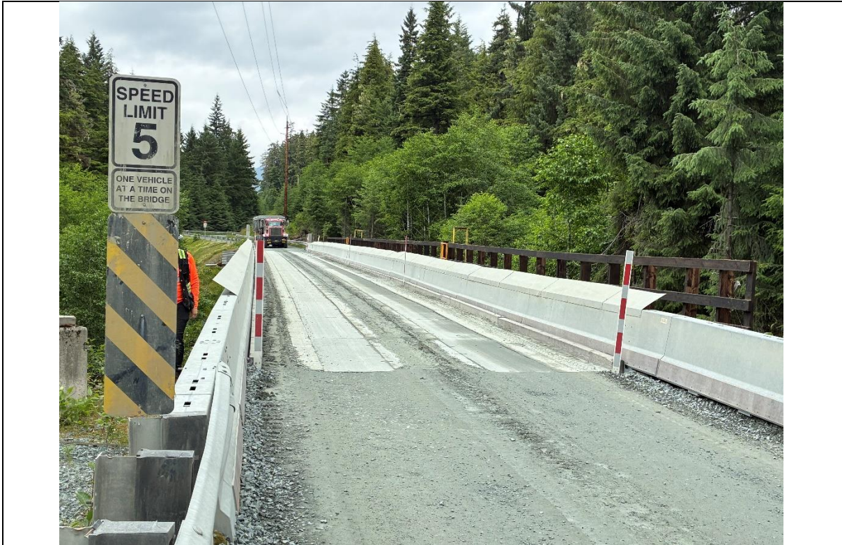
Photo 27: 3.0 Mile B-Road Bridge (Zinc Creek).
