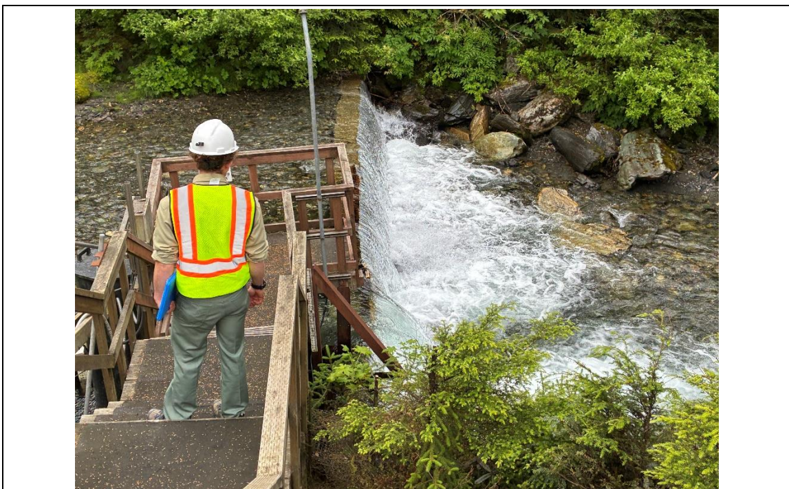
Photo 1: Greens Creek Weir.
