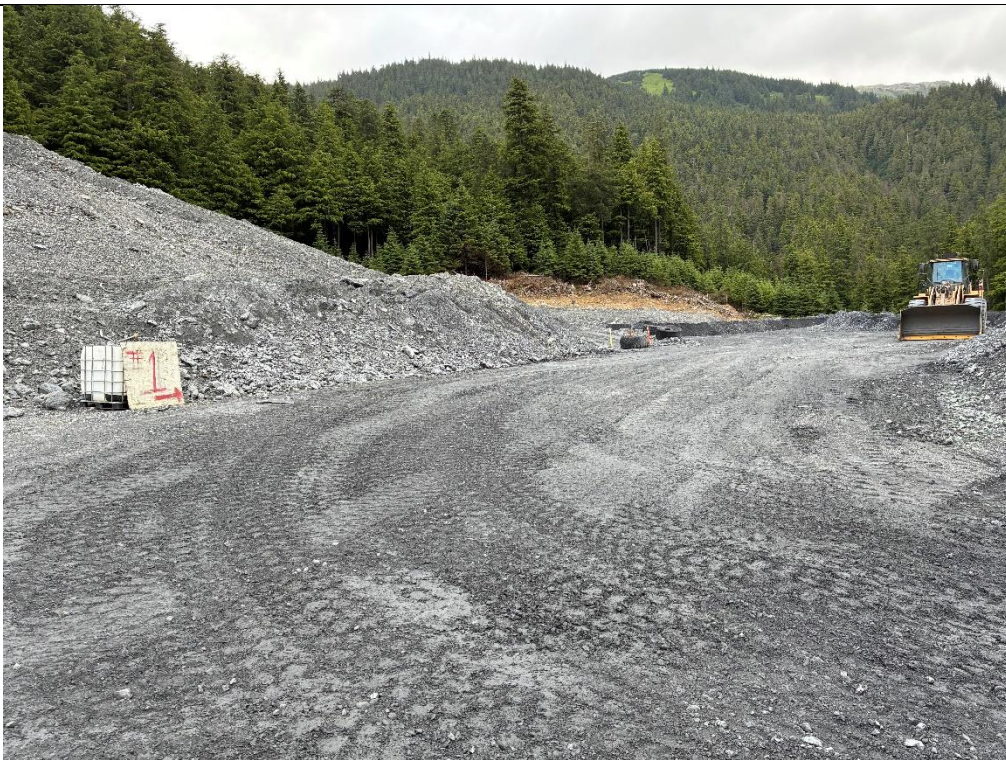
Photo 12: Site 23 Class 1 Material at base of storage area.
