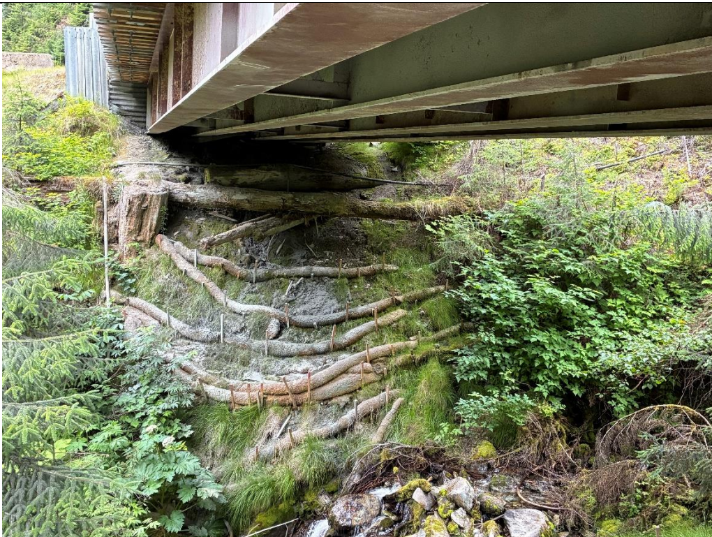
Photo 22: 7.4 Mile Bridge (Killer Creek) waddles collecting sediment (far side of creek).
