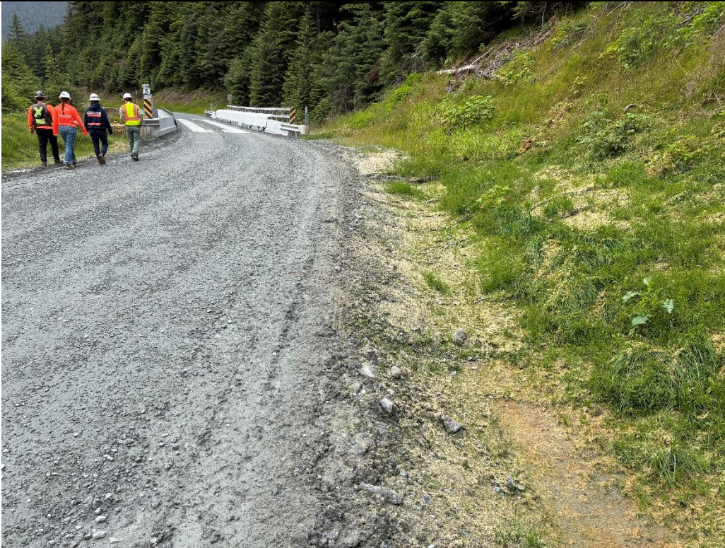
Photo 19: Mucked out and hydroseeded ditch near 7.4 Mile Bridge.
