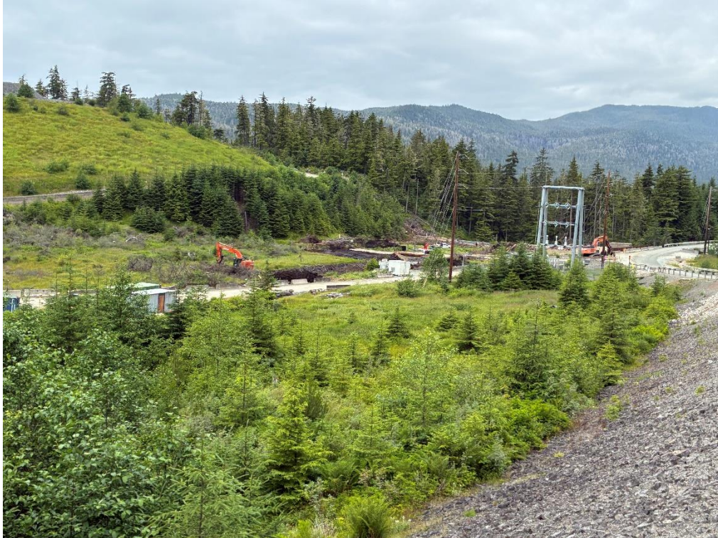
Photo 38: Overview of the NEP as seen from B Road.
