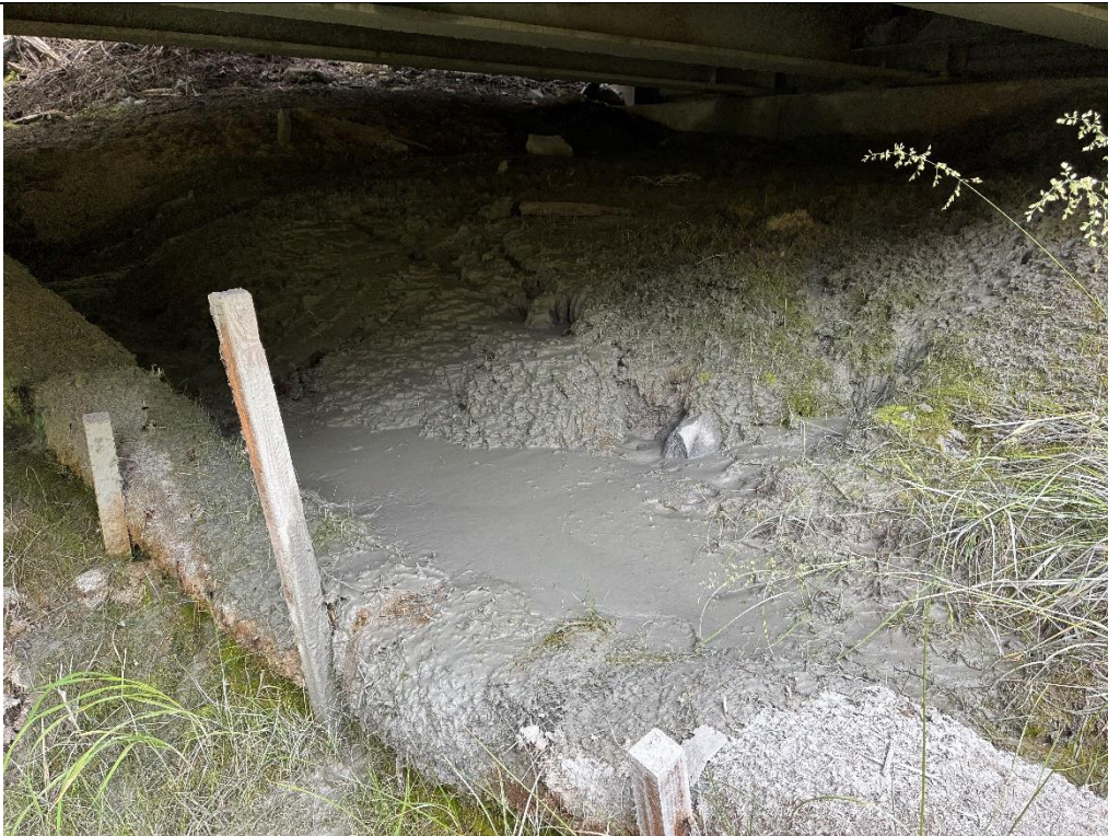
Photo 21: 7.4 Mile Bridge (Killer Creek) waddles and hydroseed present collecting sediment.
