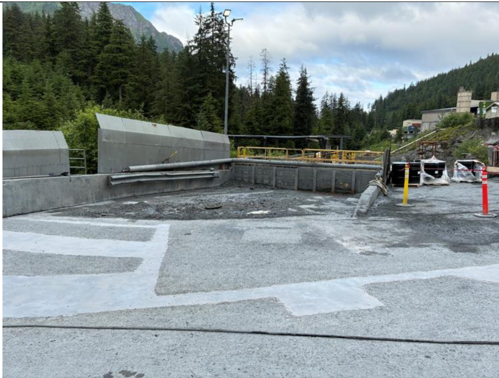
Photo 4: Degrit Basin (DB-01).
