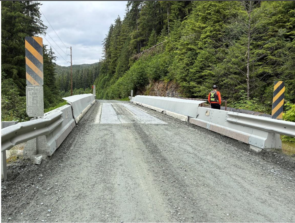
Photo 25: 3.4 Mile B-Road Bridge (Falls Creek).
