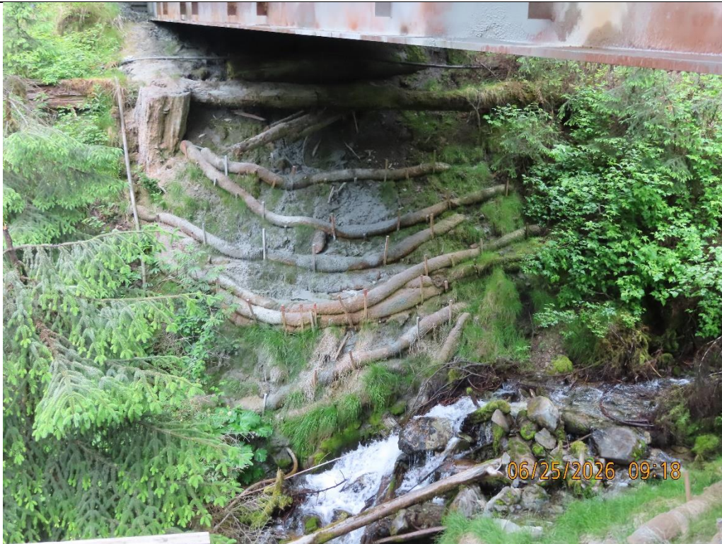
Photo 20: 7.4 Mile Bridge (Killer Creek) waddles collecting sediment (far side of creek).
