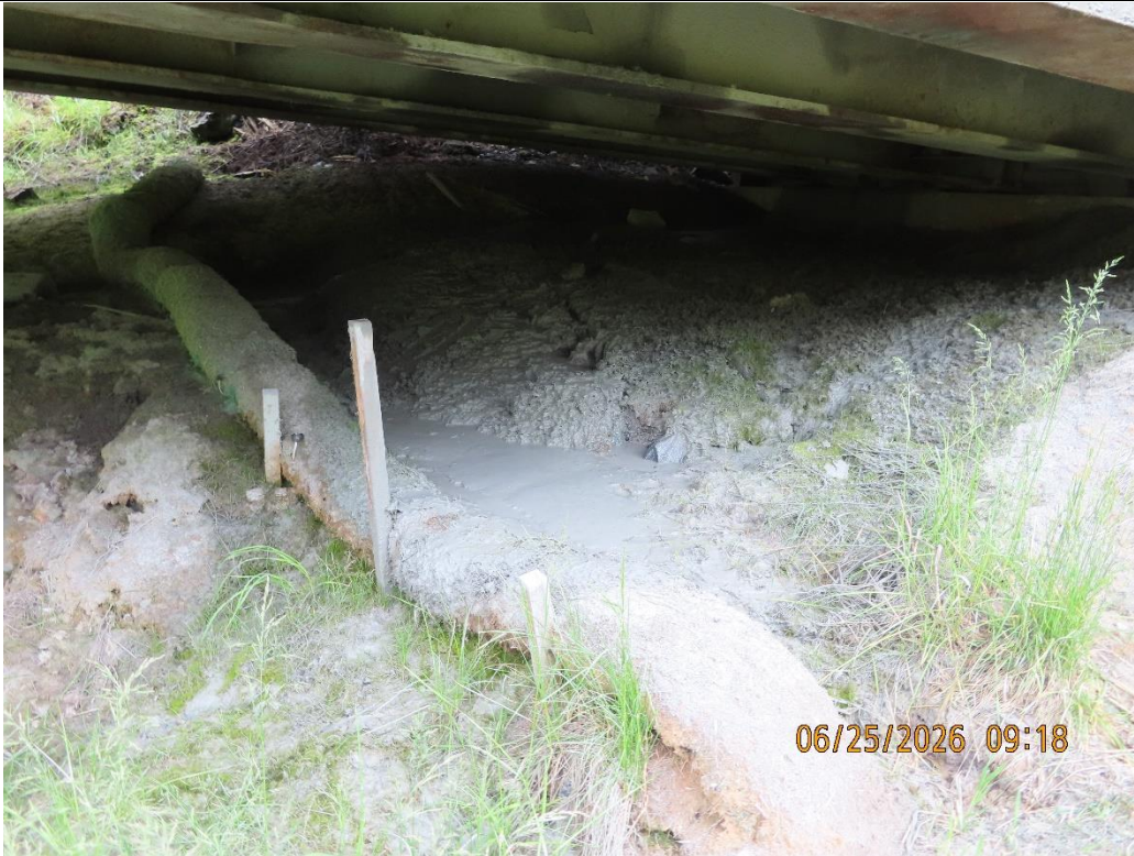
Photo 19: 7.4 Mile Bridge (Killer Creek) waddles and hydroseed present collecting sediment.
