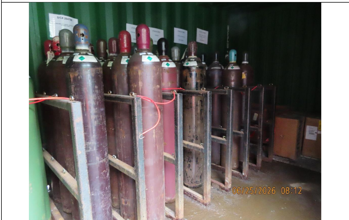
Photo 6: 920 warehouse storage container.
