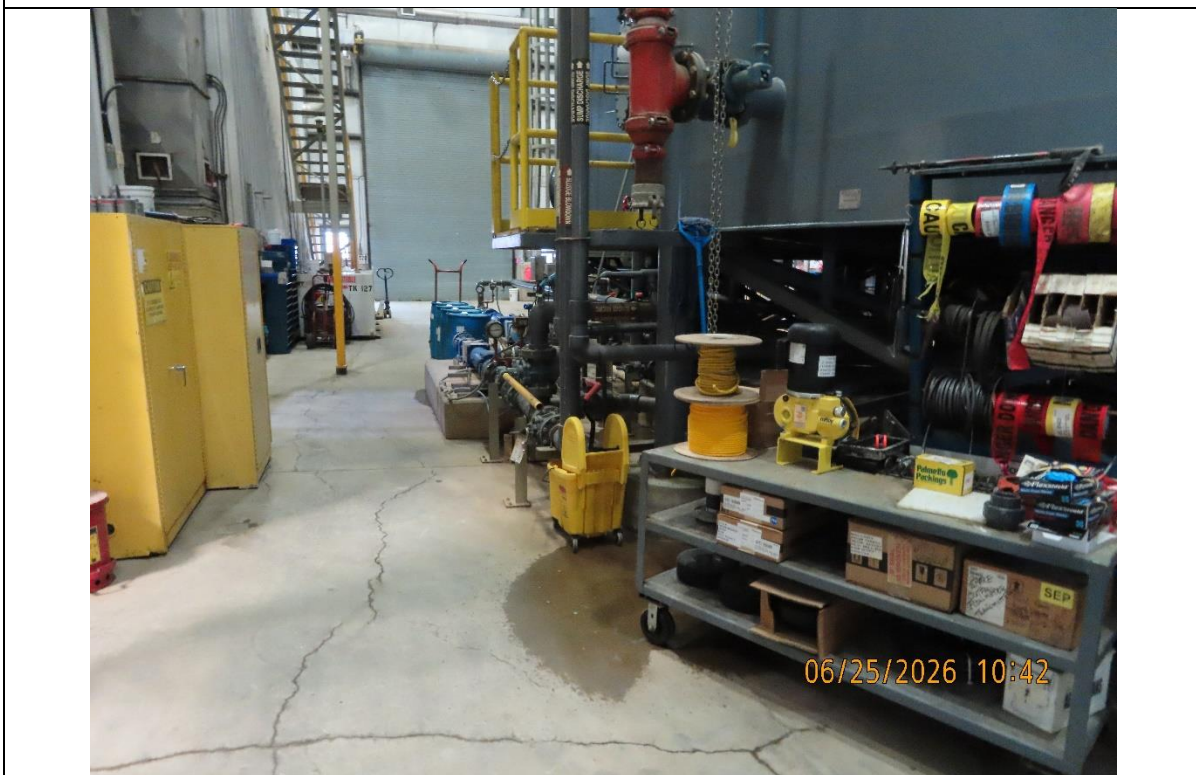
Photo 30: TDF Water Treatment Plant.
