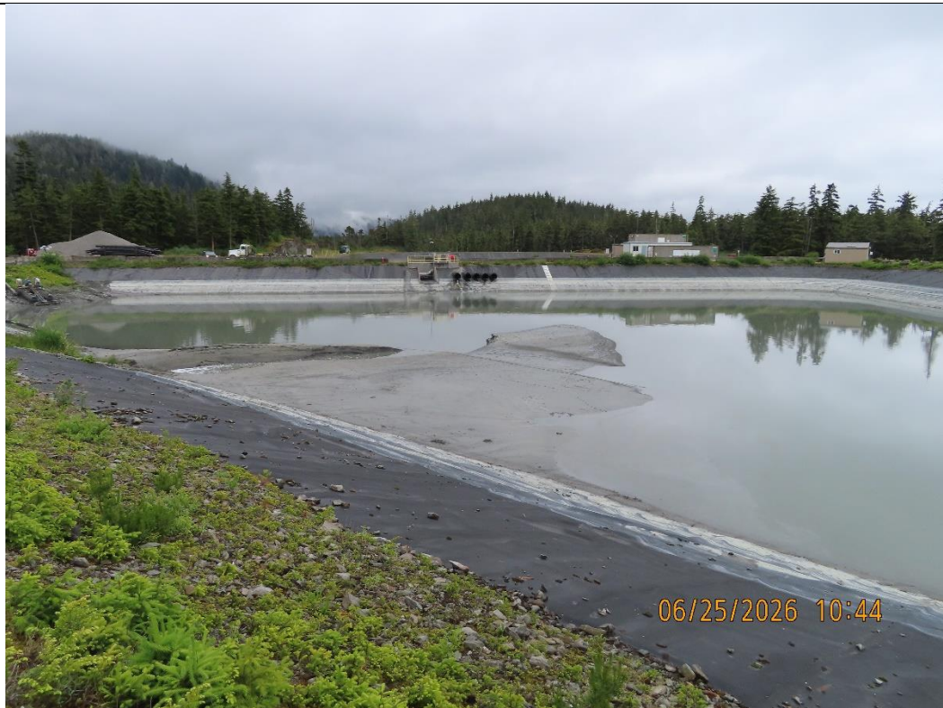
Photo 32: Pond 7 tails to be dredged and pumped to bags in Pond 10.
