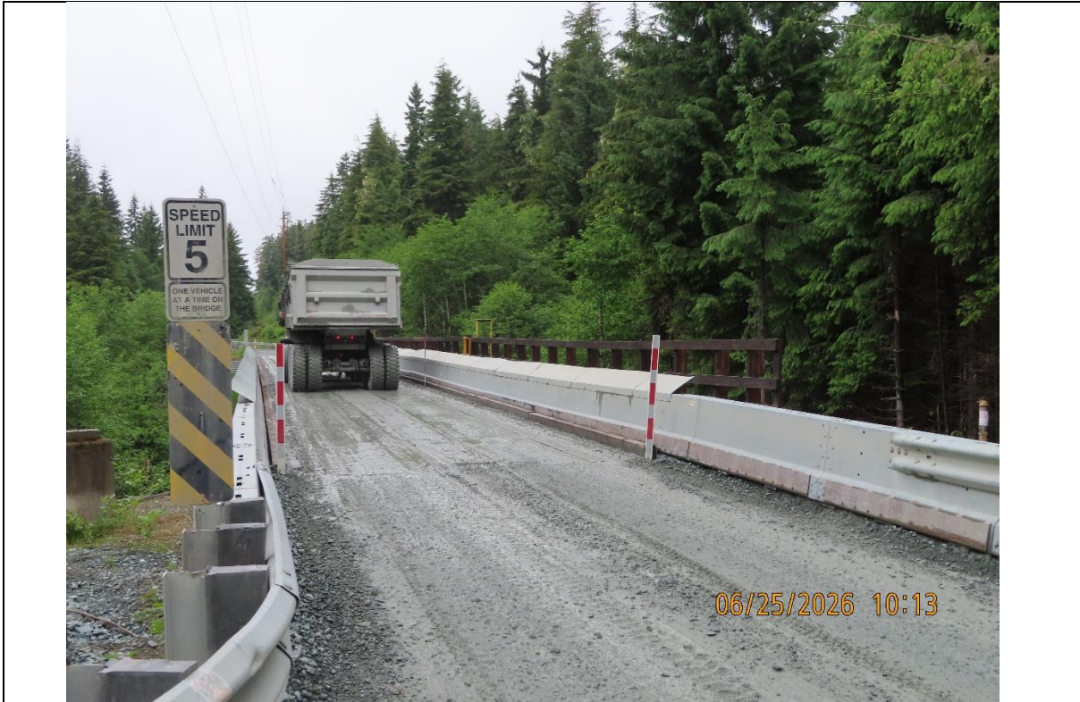
Photo 25: 3.0 Mile B-Road Bridge (Zinc Creek).
