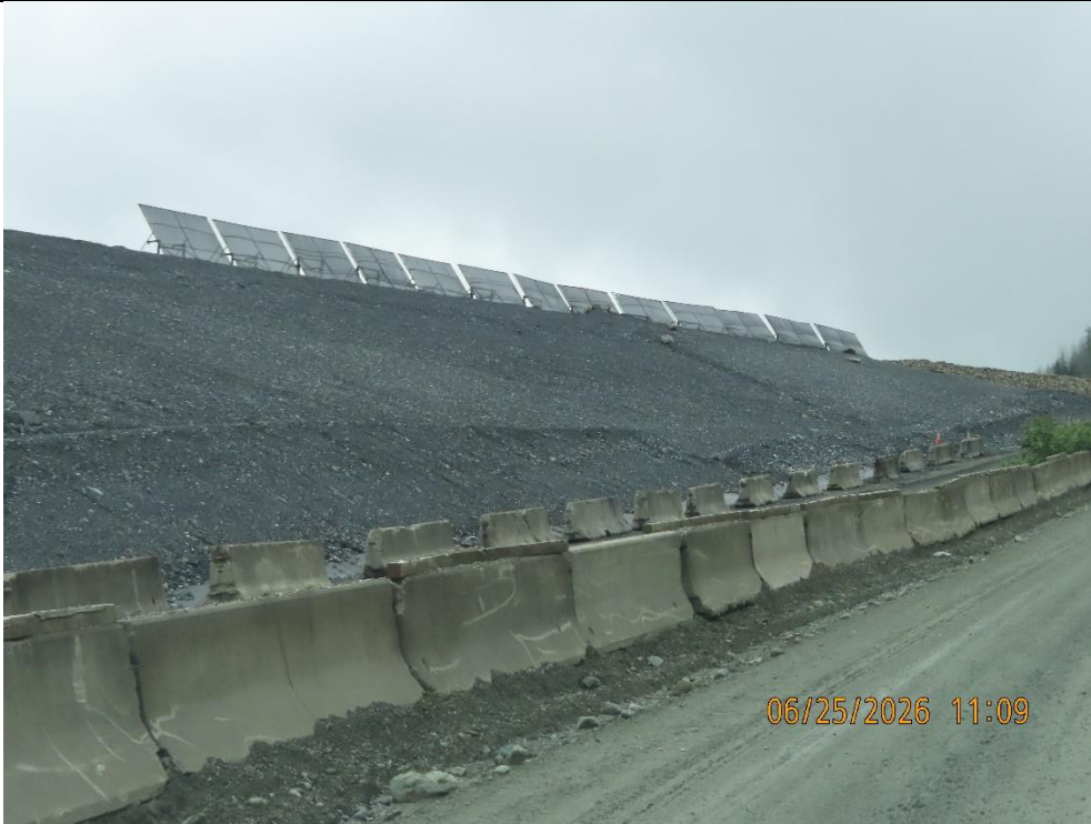
Photo 35: Portable Fugitive Dust Mitigation at the Tailings Disposal Facility.
