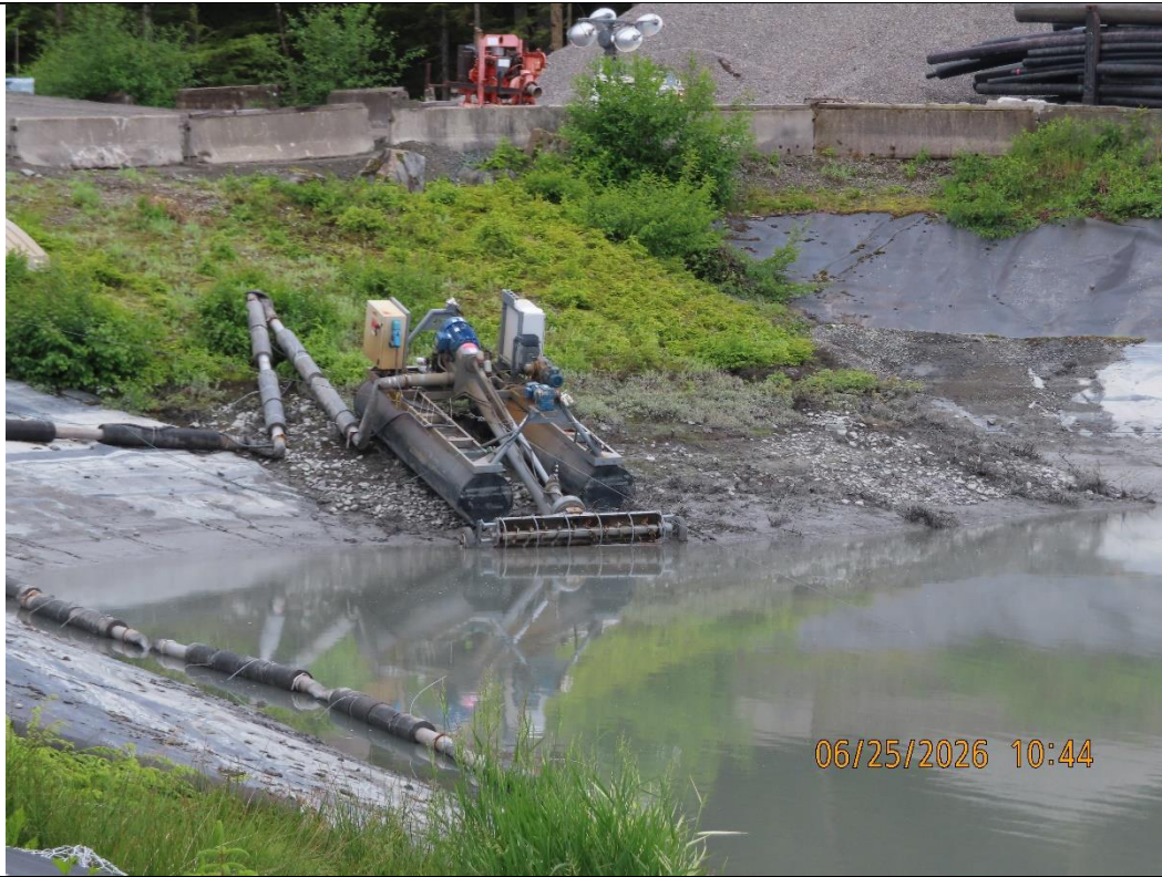
Photo 31: Pond 7 dredge staged.
