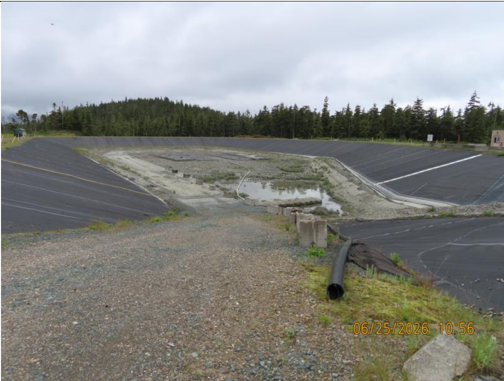
Photo 33: Overview of Pond 10 with tails bags in background and fill pipe in foreground.
