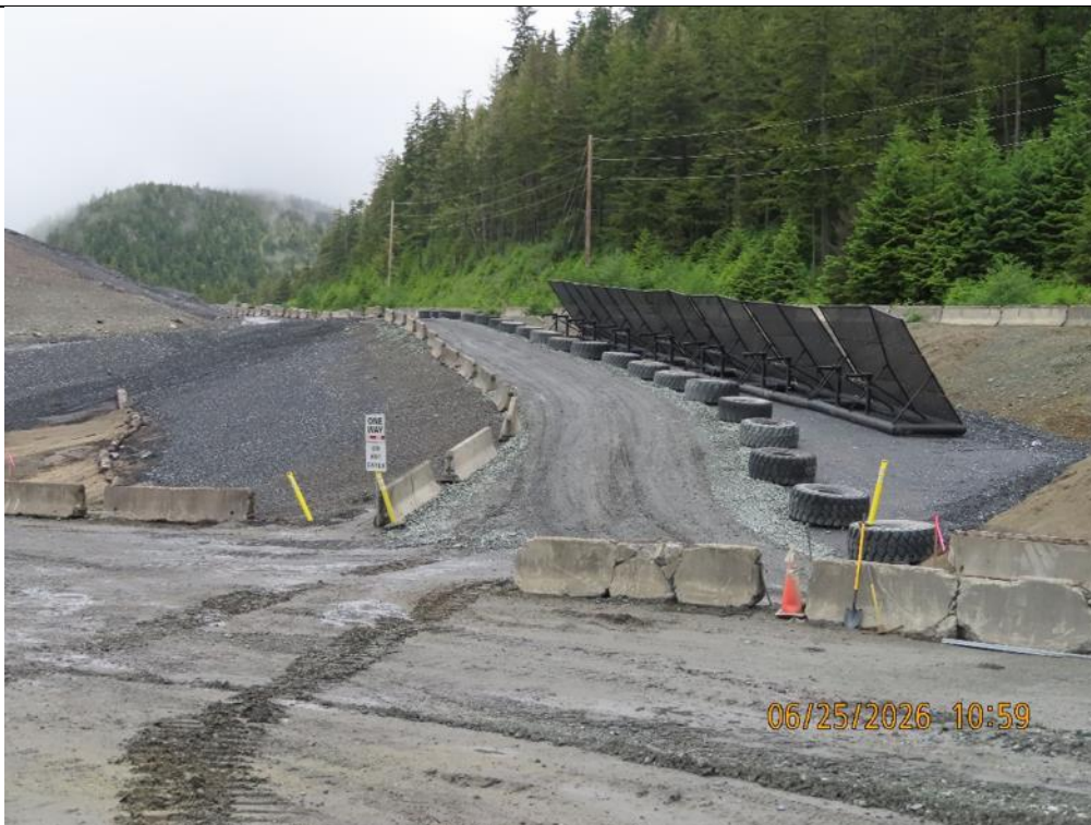
Photo 36: Portable Fugitive Dust Mitigation at the Tailings Disposal Facility.
