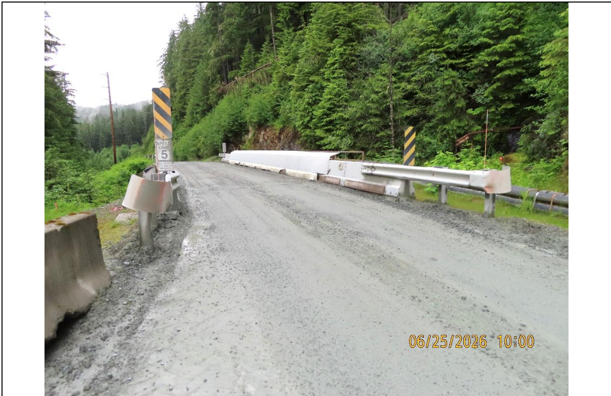
Photo 23: 3.4 Mile B-Road Bridge (Falls Creek).
