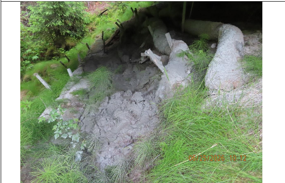
Photo 26: 3.0 Mile B-Road Bridge (Zinc Creek) sediment collected before decking replacement.
