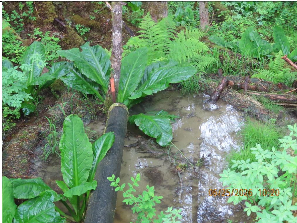
Photo 28: Gnome Ponds outfall.
