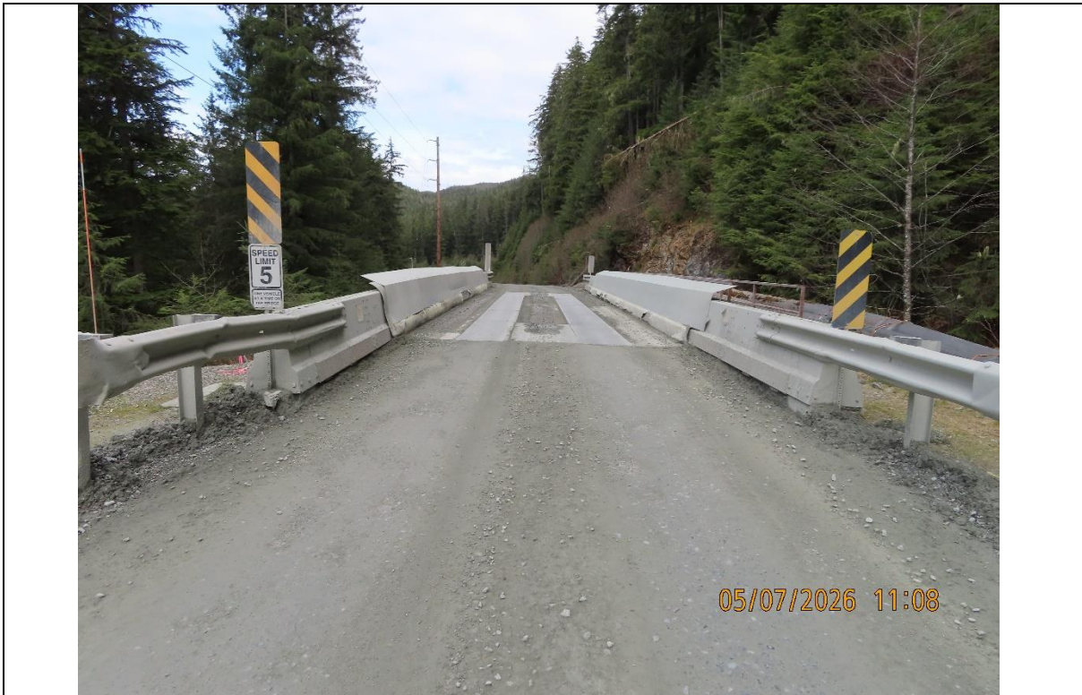
Photo 19: 3.4 Mile B-Road Bridge (Falls Creek).
