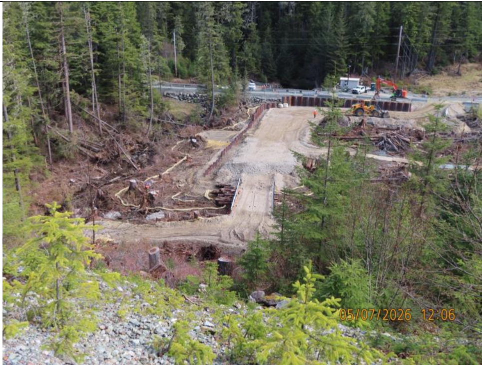
Photo 34: North Expansion Project area looking back at B Road.
