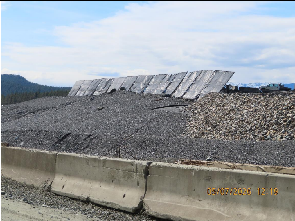
Photo 32: Portable Fugitive Dust Mitigation at the Tailings Disposal Facility.
