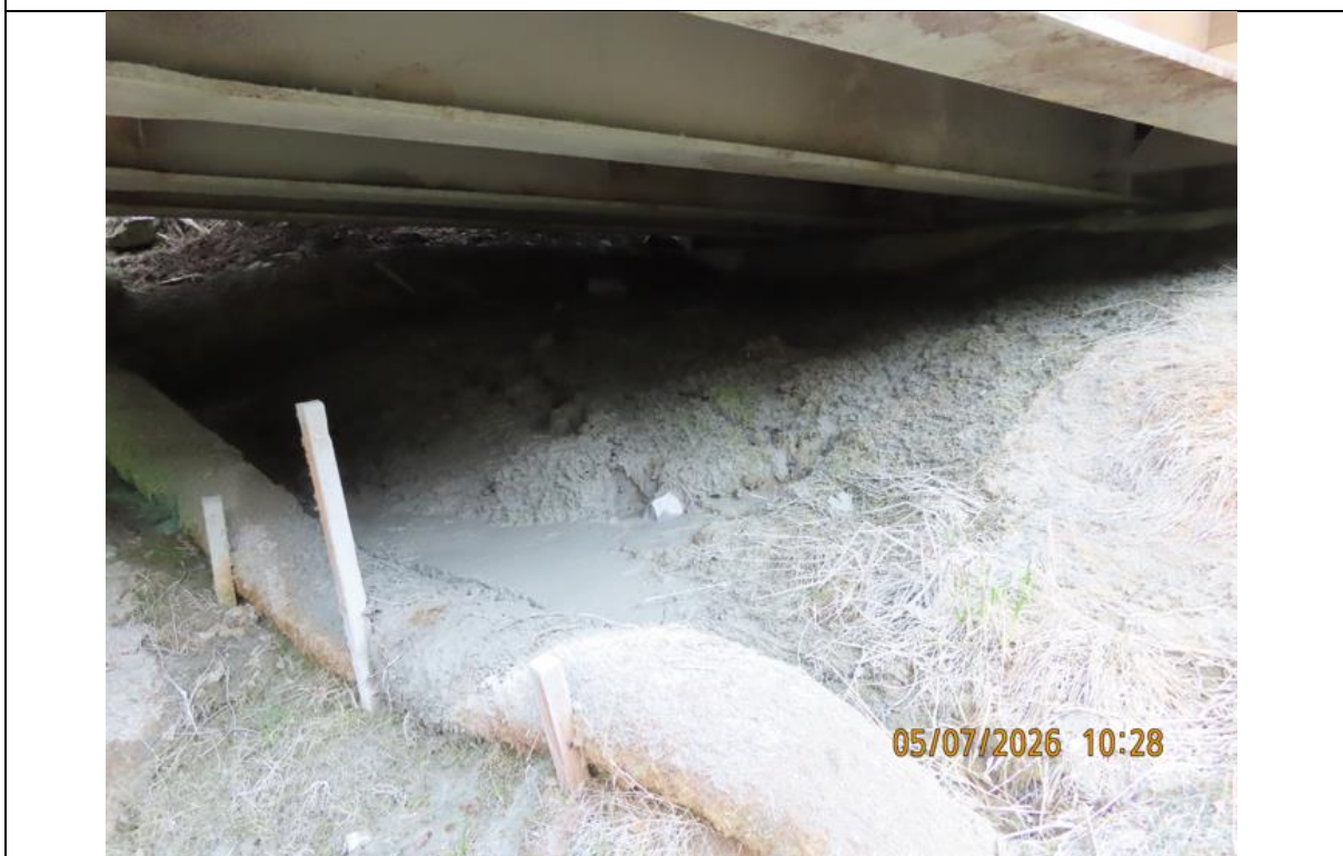
Photo 16: 7.4 Mile Bridge (Killer Creek) waddles and hydroseed present collecting sediment.
