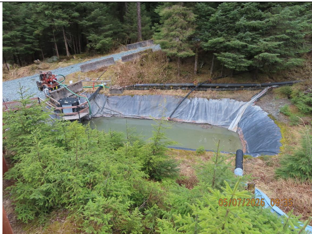
Photo 10: Upper C Pond. Evidence of raised pond level but no overflow outside of the pond.
