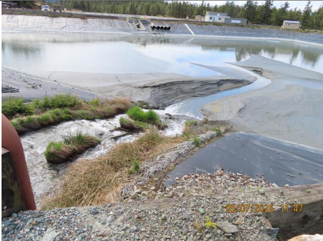
Photo 30: Pond 7 tails to be dredged and pumped to bags in Pond 10.
