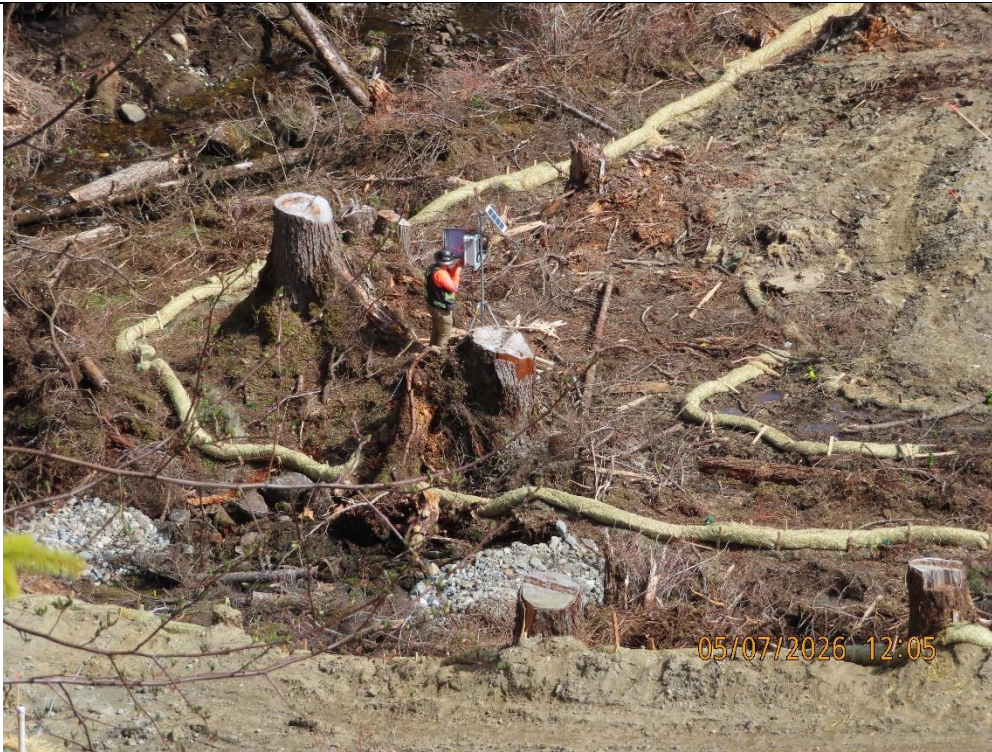
Photo 33: North Expansion Project area.
