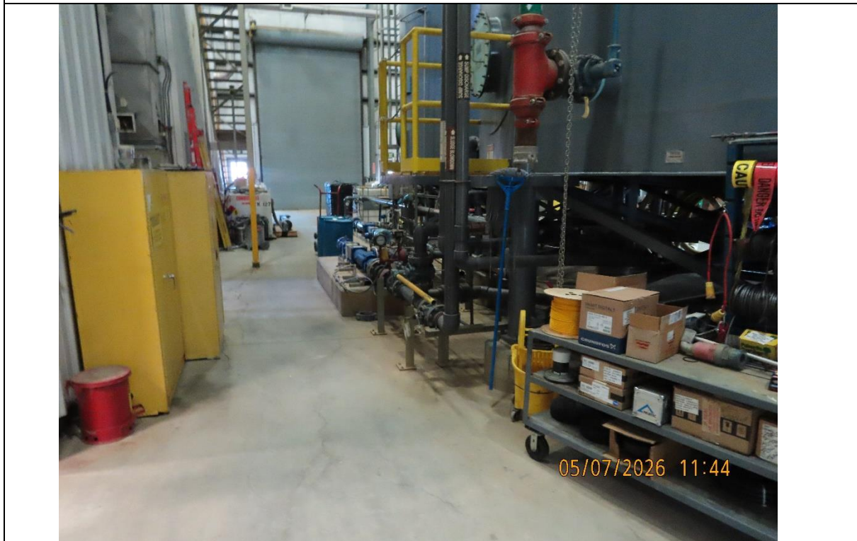
Photo 28: TDF Water Treatment Plant.
