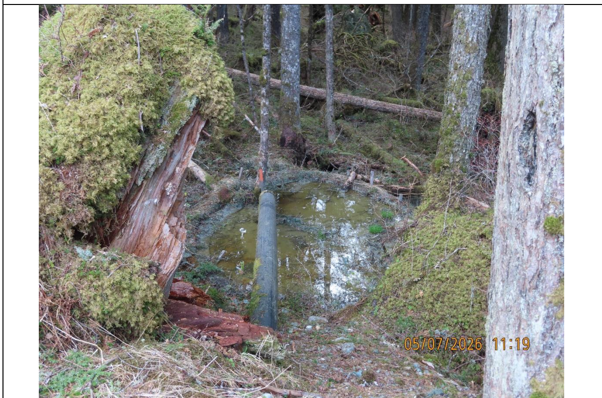
Photo 24: Gnome Ponds outfall.
