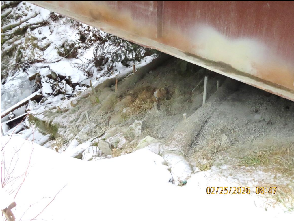
Photo 17: 7.4 Mile Bridge (Killer Creek) waddles and hydroseed present collecting sediment.
