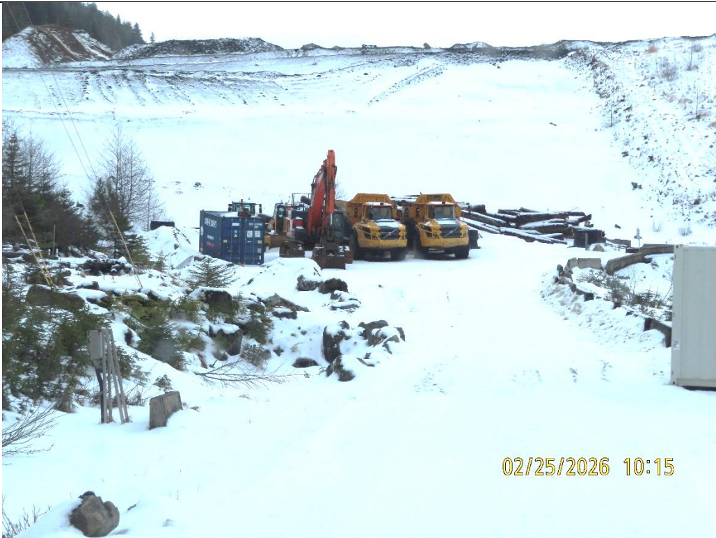
Photo 33: North Expansion Project prework storage area.
