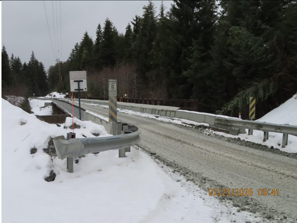
Photo 21: 3.0 Mile B-Road Bridge (Zinc Creek).
