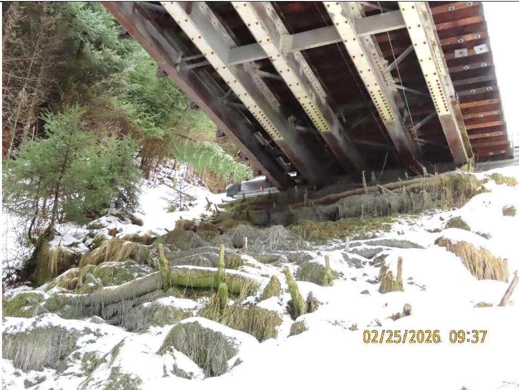
Photo 23: 3.0 Mile B-Road Bridge (Zinc Creek) showing sediment catchment features.
