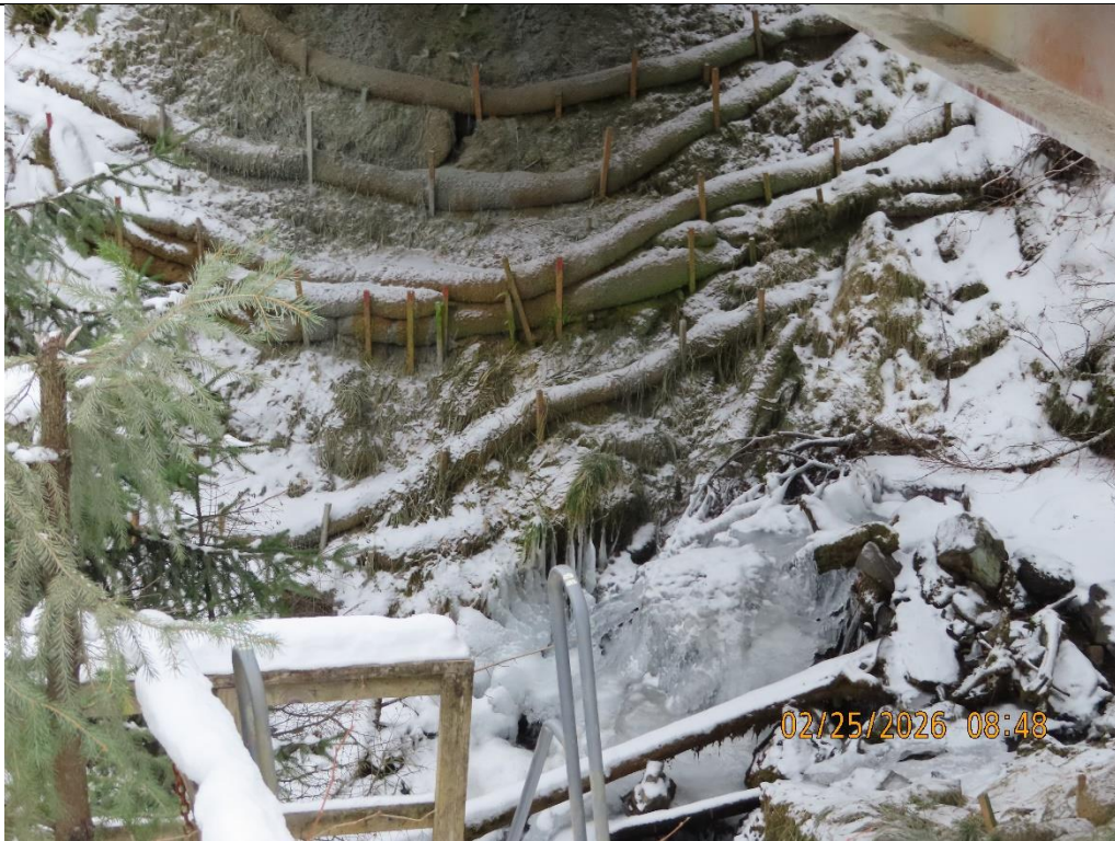
Photo 16: 7.4 Mile Bridge (Killer Creek) waddles and hydroseed present collecting sediment.
