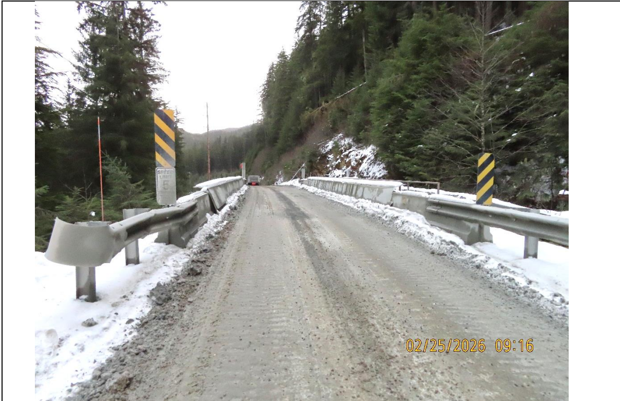
Photo 19: 3.4 Mile B-Road Bridge (Falls Creek).
