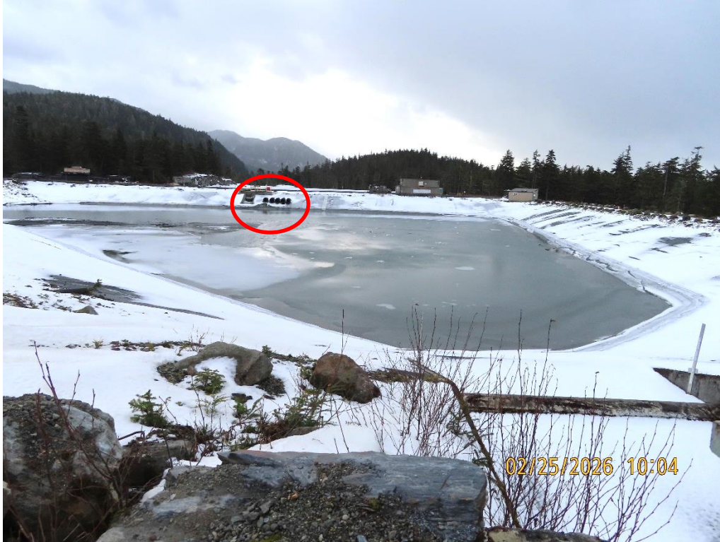
Photo 29: Pond 7 from spillway with culverts connecting Pond 7 to 10 in the background
