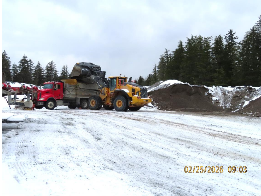
Photo 18: Disposal Site E showing road maintenance activity and gravel storage.
