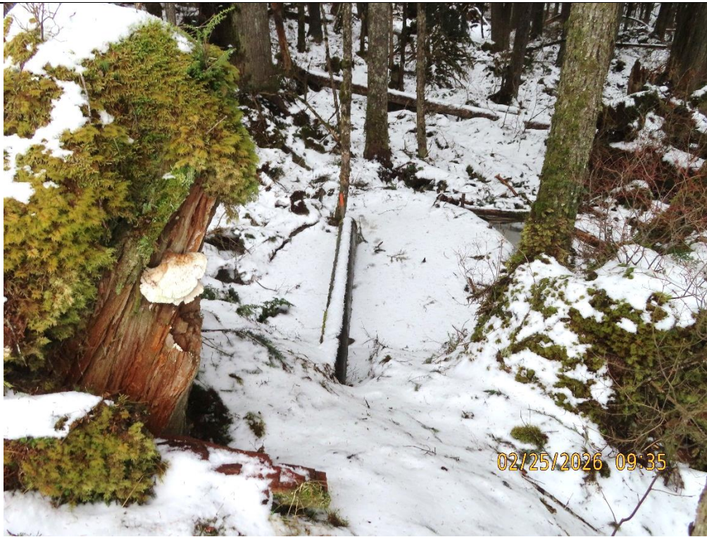
Photo 25: 3.0 Mile B-Road Gnome Ponds outfall.
