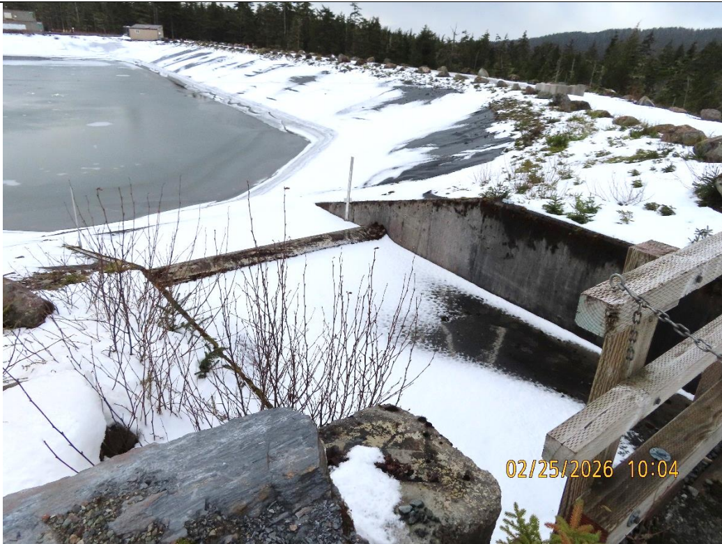
Photo 27: Spillway at Pond 7. No evidence of water overflow.
