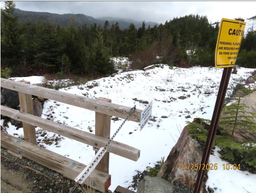
Photo 28: Pond 7 spillway outfall. No signs of overflow entering this area.
