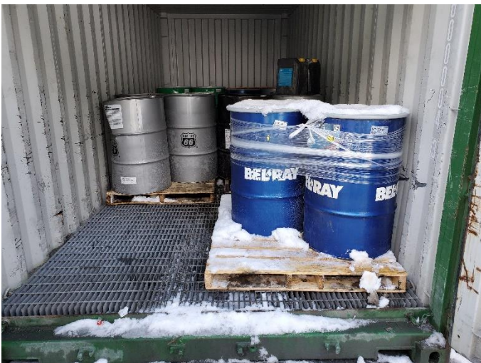
Storage behind the 920 Warehouse. <=Secondary containment
