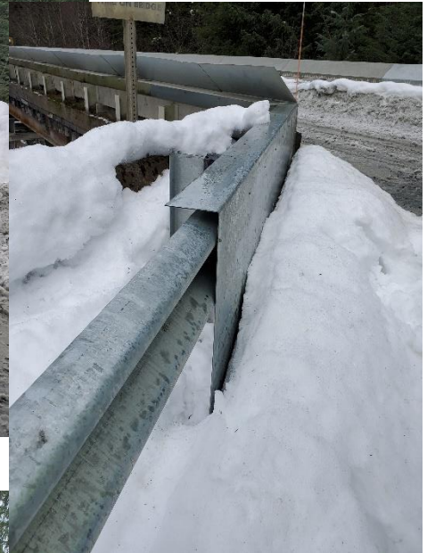
New Splash Guard installed.
