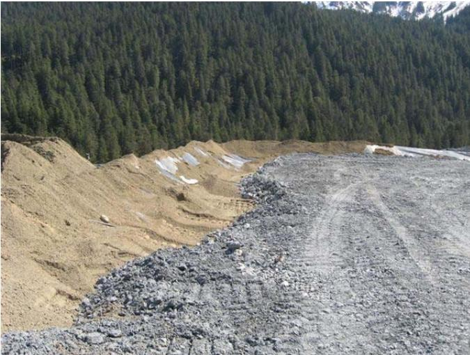
**Site 23 pad with sand and class 3 rock over synthetic liner.**
