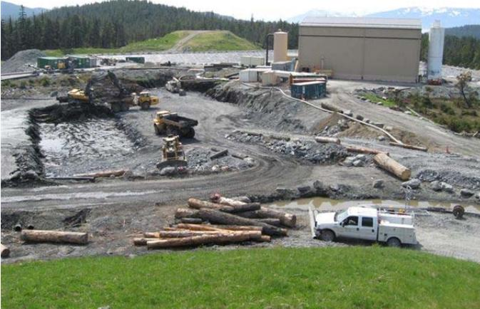
**Pond 6 excavation showing the new access road constructed to the right of the photograph to bring rock in from the “clean” road.**
