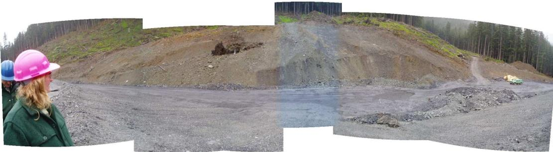
*Site 23 – waste placement regime showing progressive placement of a 5-foot layer of Class I production rock at the lower aspect of the facility (upgradient FWMP well #57 in background near treeline)*
