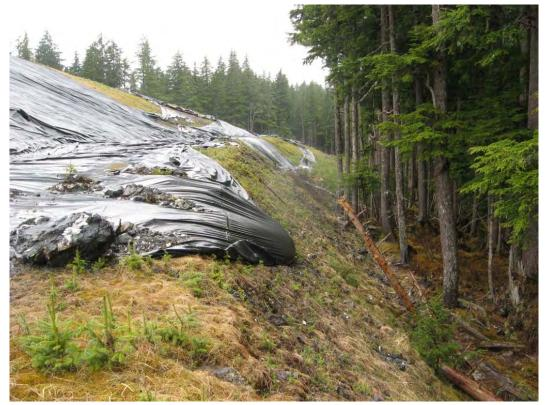
Photo 14: Part of Site E has been covered by a geomembrane to reduce infiltration in the short term
