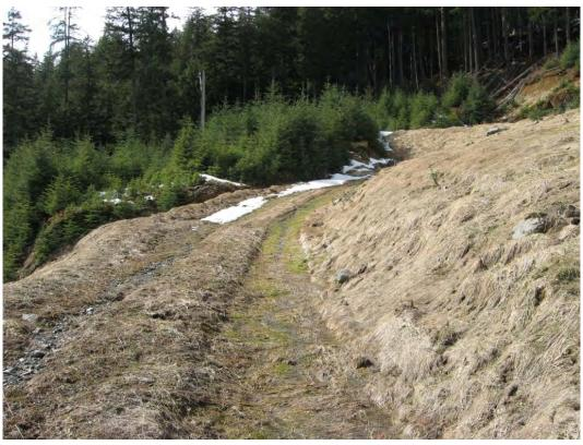
Photo 15: Access ramp across the front of the reclaimed and revegetated production rock at Pit 405
