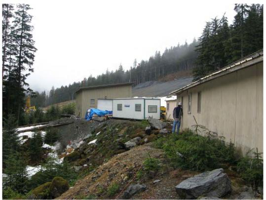
Photo 12: Side view, looking west at mine buildings which have been constructed on fill within Site C, part of Site C has no production rock
