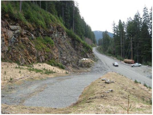
Photo 19: Looking down the access ramp that overlies reclaimed and revegetated production rock in Pit 174
