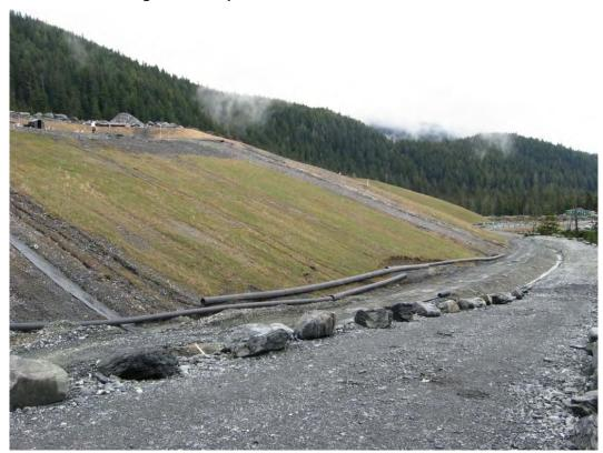
Photo 6: A revegetated slope, with a granular toe buttree, on the west side of the Tailings Disposal Facility
