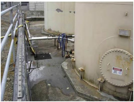
Photo 29: Secondary Containment for Fuel Storage at 920 Area
