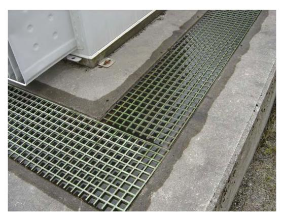
Photo 3: Transformer Secondary Containment
