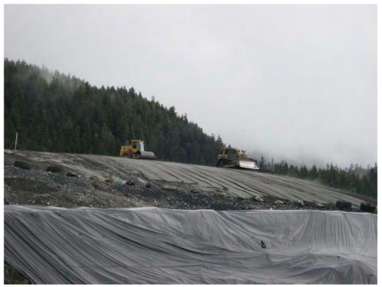
Photo 5: After spreading, the tailings are compacted with a self propelled, vibratinng drum compactor
